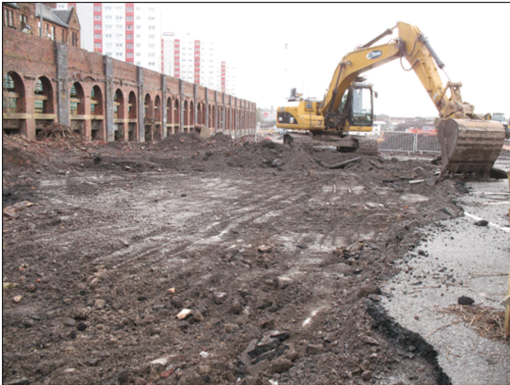
Figure 3b: Shot of sensitive area from the northwest after the general reduction by 350-400mm
