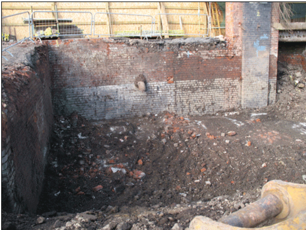
Figure 4b: Northeast excavated area from the southwest
