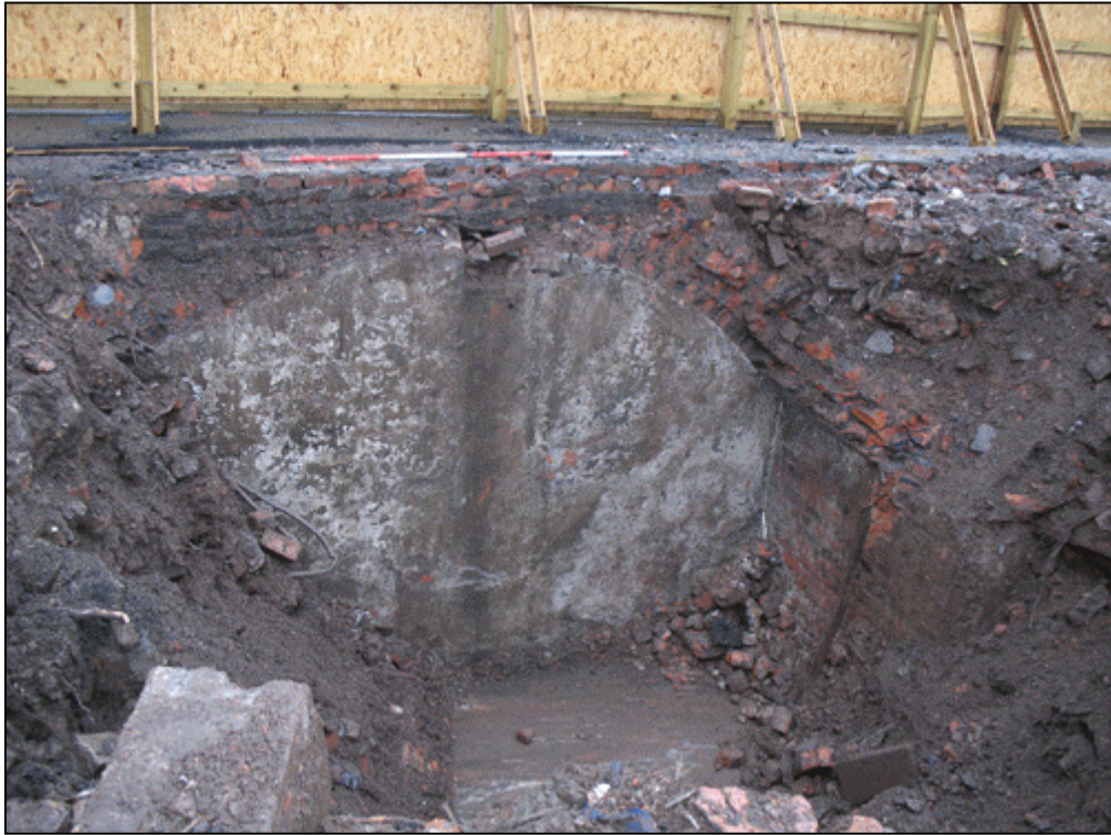
Figure 4a: Northwest excavated area from the southwest
