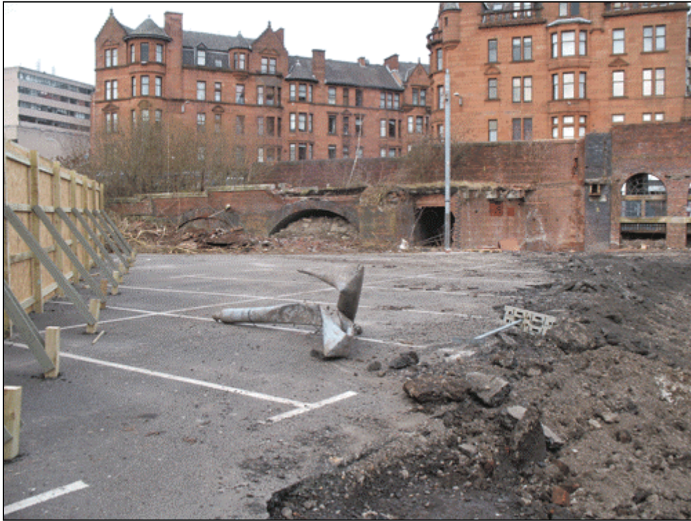
Figure 3a: Pre ex shot of sensitive area from the southeast, showing the access ramp in the background prior to its demolition
