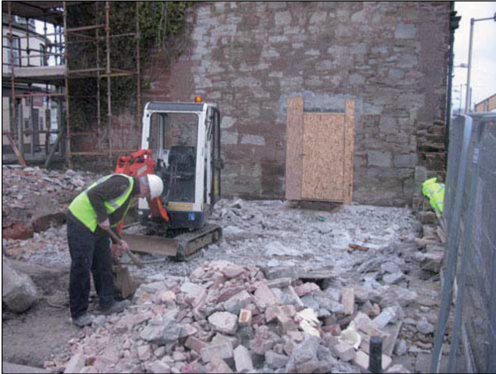
Figure 5a: After breaking the concrete slab
