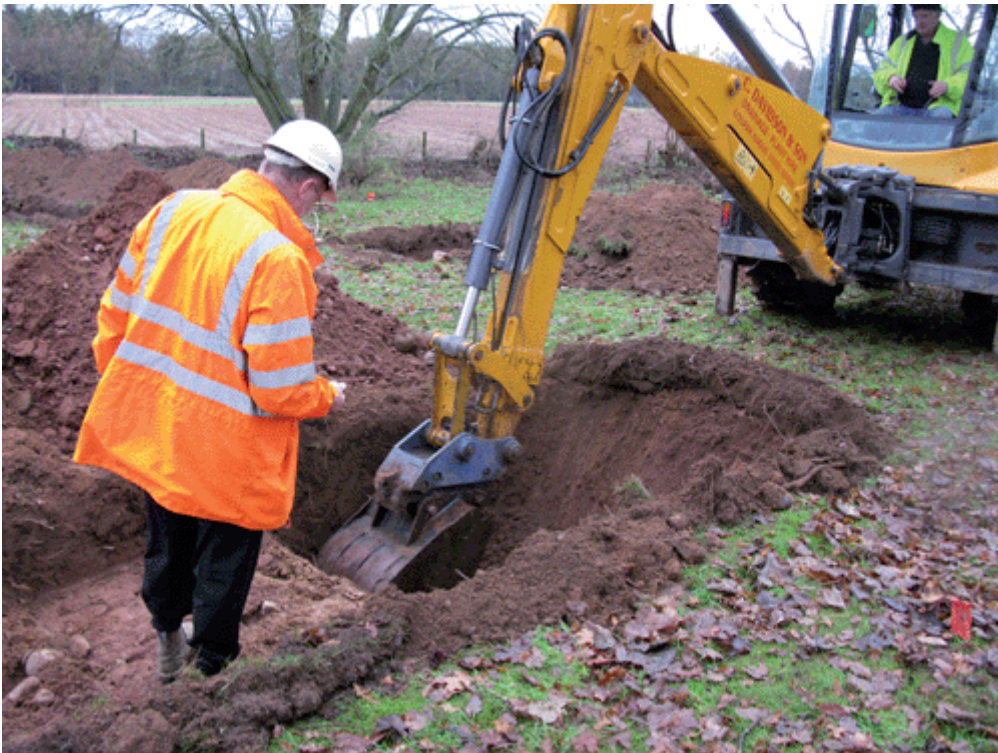
Figure 5b: Geo-technical test pitting in Trench 2 from the southwest
