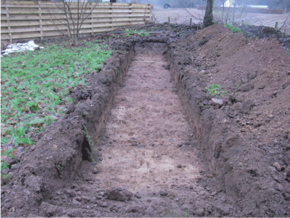
Figure 5a: Trench 4 from the south-south-west
