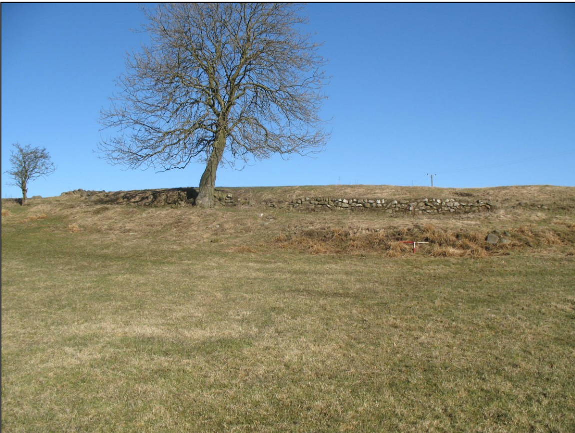
Figure 3b: West Kitchen Green ( RA10007.5 ) - Access Track with Stone Revetment Beyond
