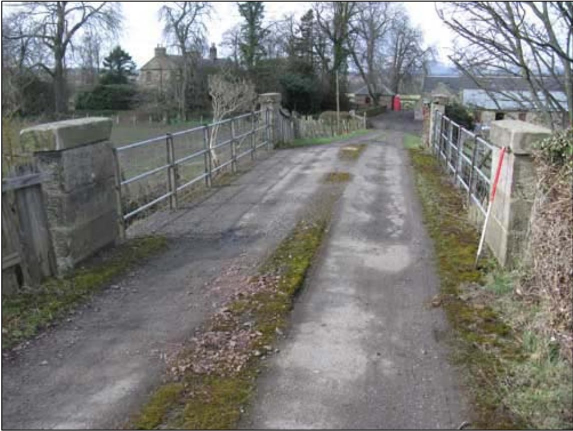
Figure 9a: Railway Overbridge near Redheugh - Original Masonry and Later Railings
