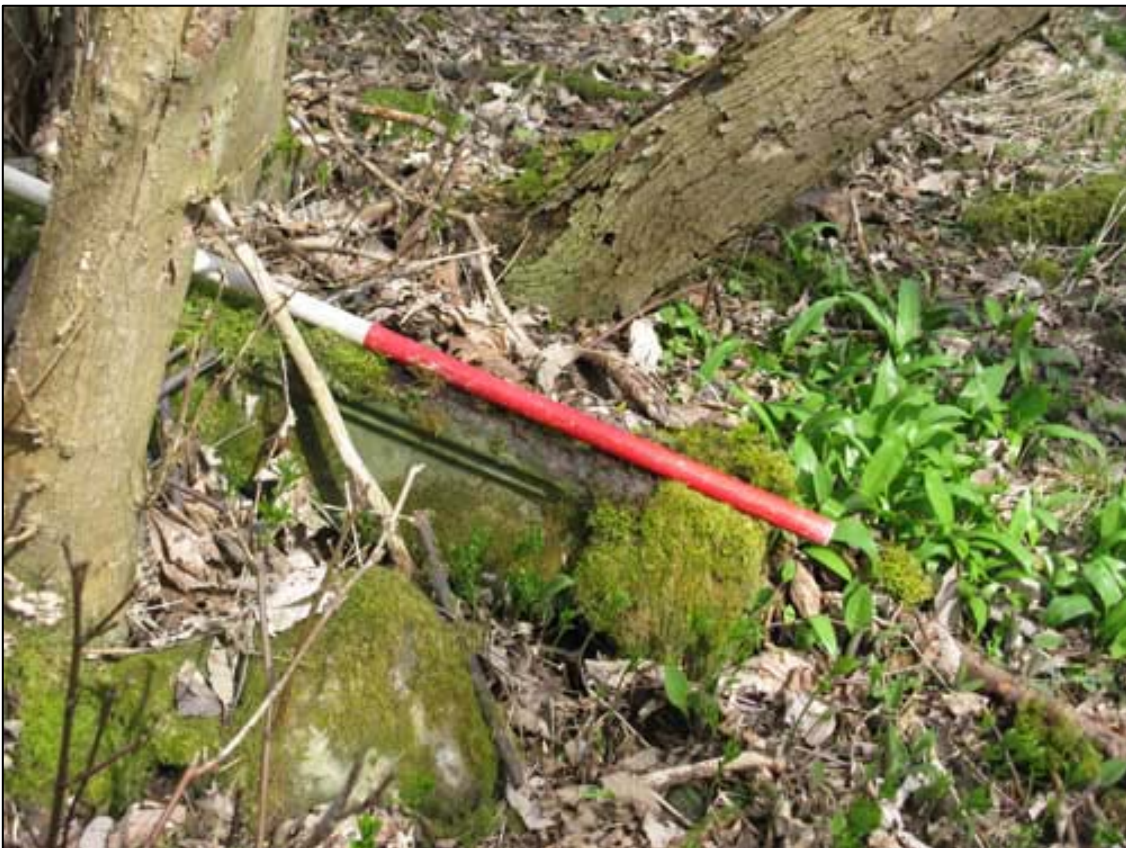
Figure 7b: Prestonholm House S1 – Worked Stone Lintel of 19th Century Date
