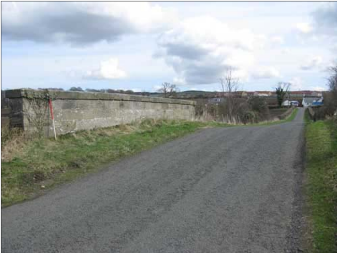
Figure 9b: Railway Overbridge to south of Redheugh – Original Parapet
