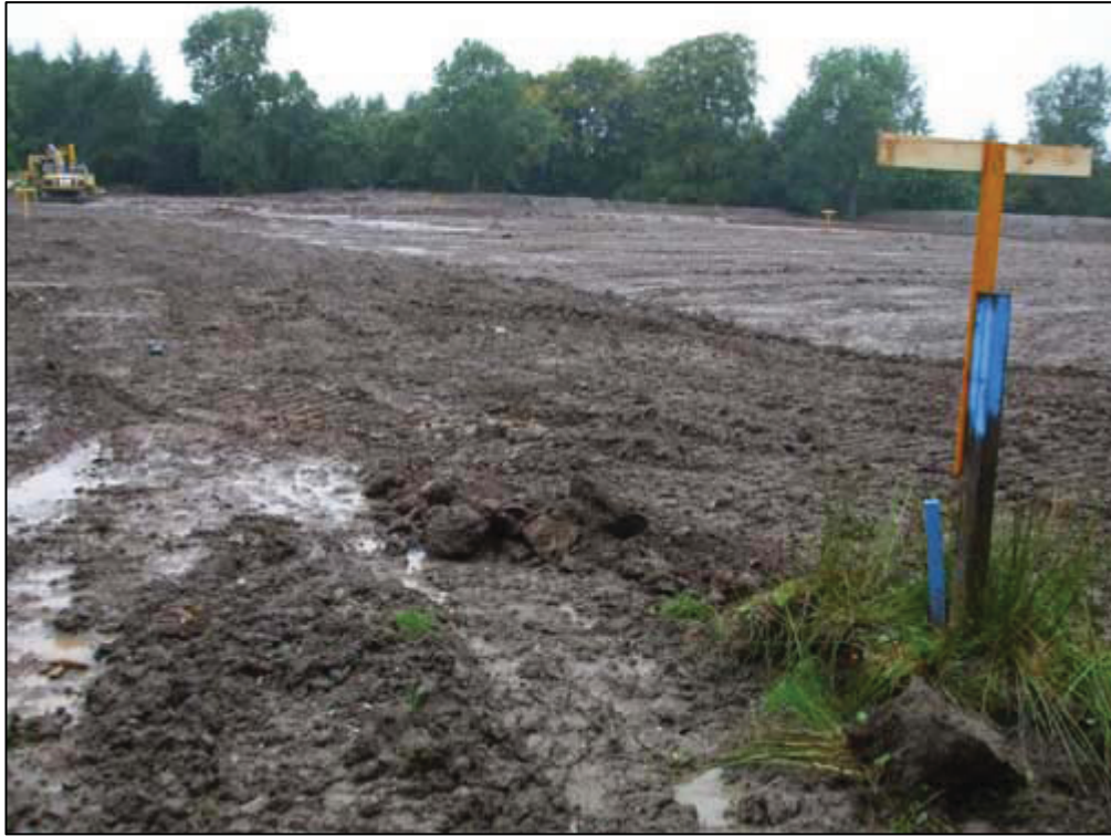
Figure 3a: Trench 1, Subsoil exposed
