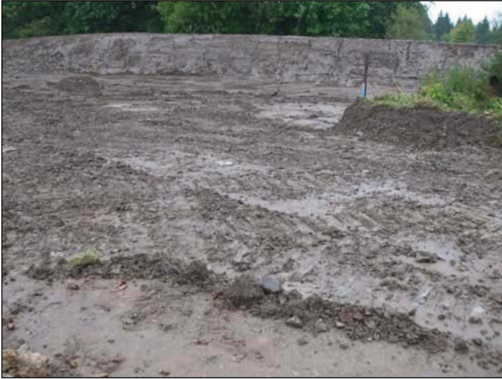
Figure 4a: Ground Reduction in North-East Corner of Sports Arena
