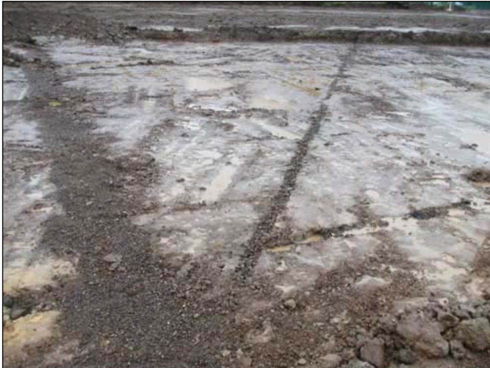
Figure 4b: Network of Field Drains in Southern Portion of Site
