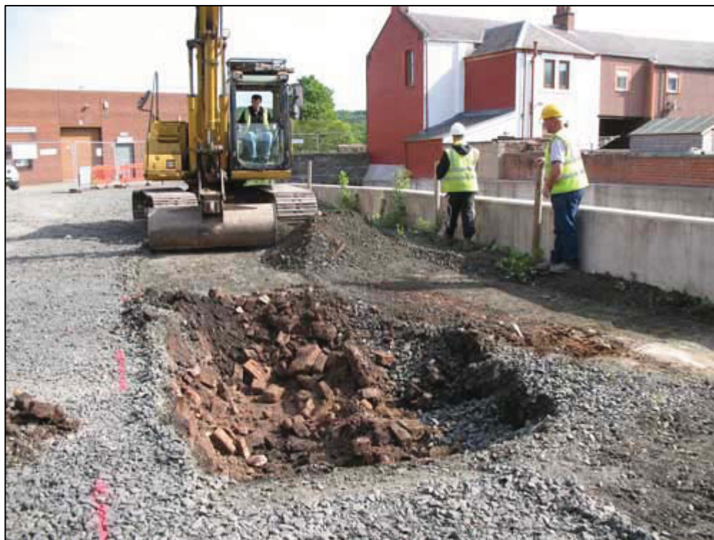
Figure 3a: Demolition Layer (002) revealed at E side of Site (Area A)
