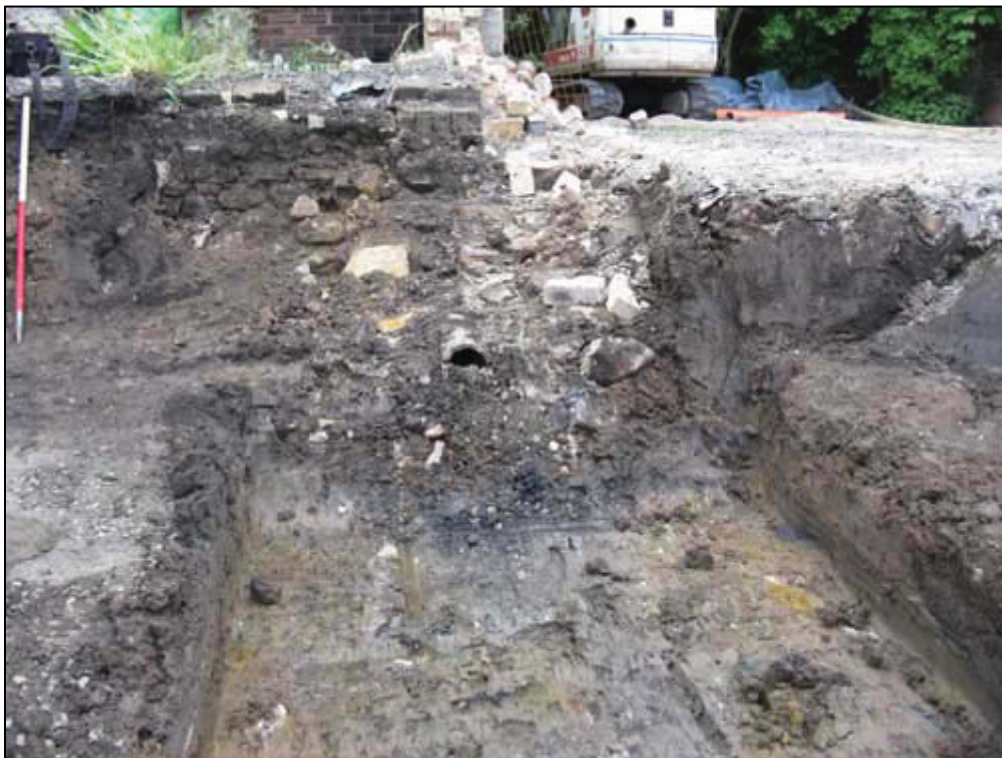
Fig. 5b: View along Line of Wall (005) & Underlying Drain, with Revetment Wall (012) to Left
