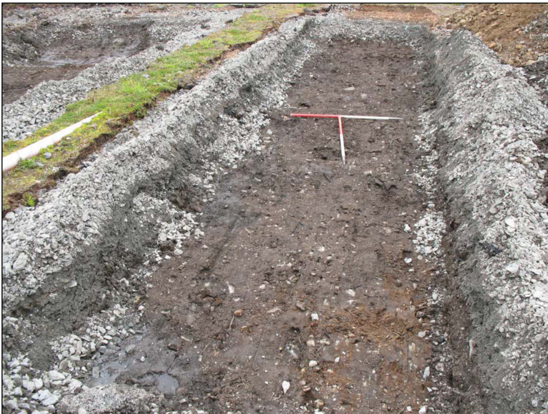
Figure 4b: Trench 1 – Subsoil exposed
