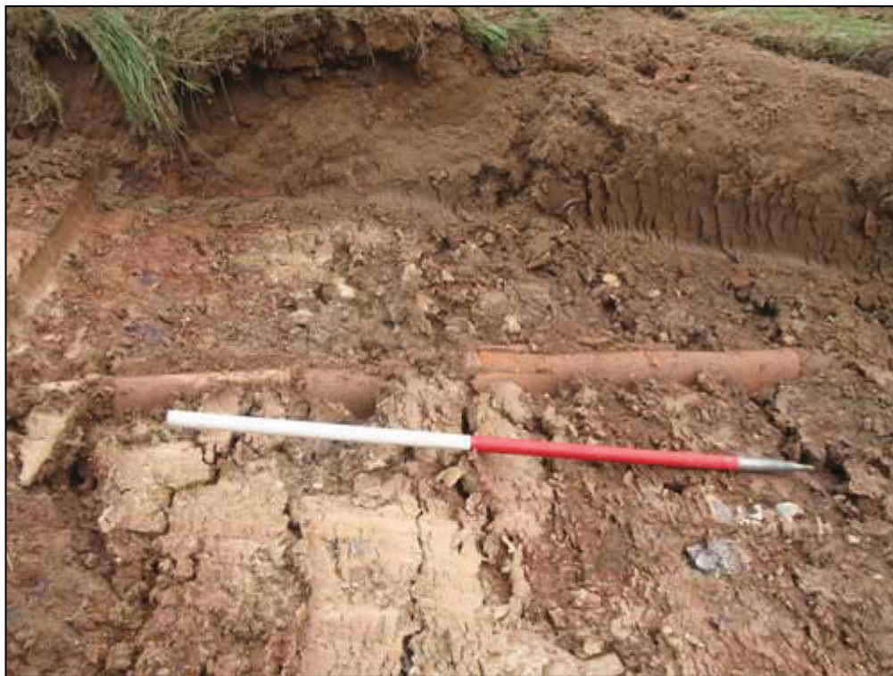
Figure 4b: Linear Feature (110) - (Ceramic Tile Field Drain)
