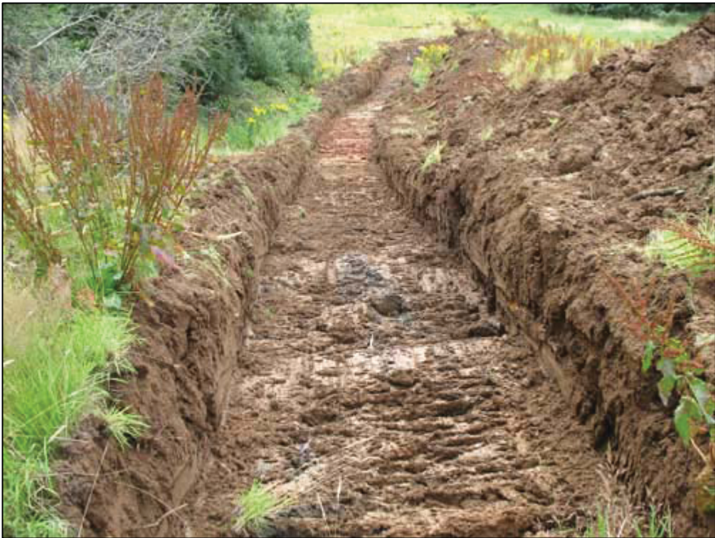
Figure 5a: Trench 1, Fully Excavated
