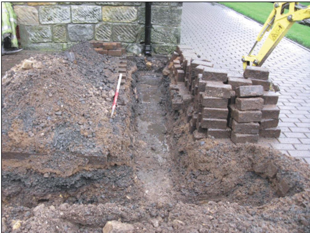
Figure 3b: Drainage trench running north-south
