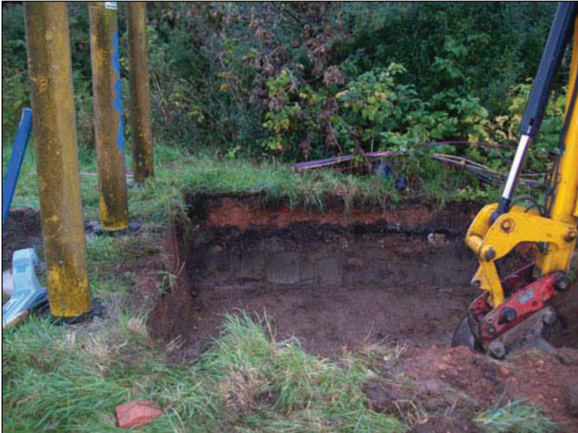
Figure 5b: Pit for new lighting base
