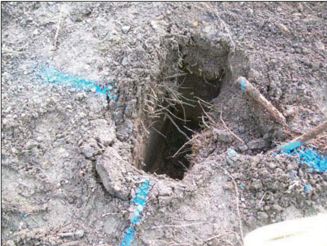
Figure 6b: Pit for fence line
