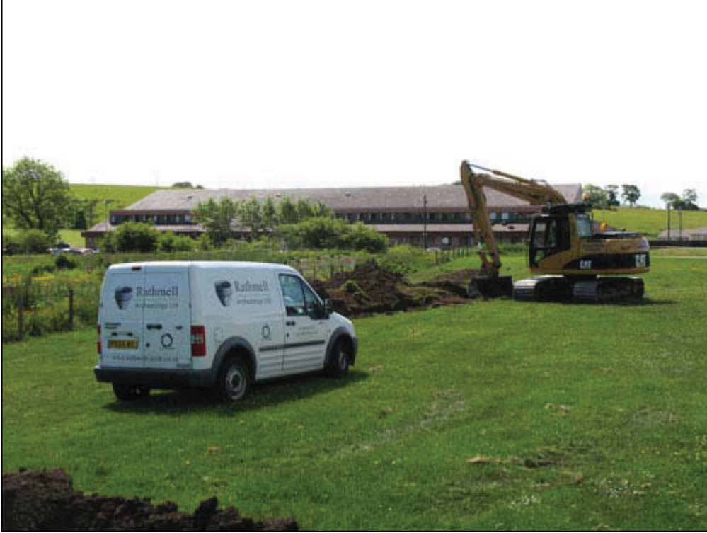
Figure 3a: Working in western boundary of development area
