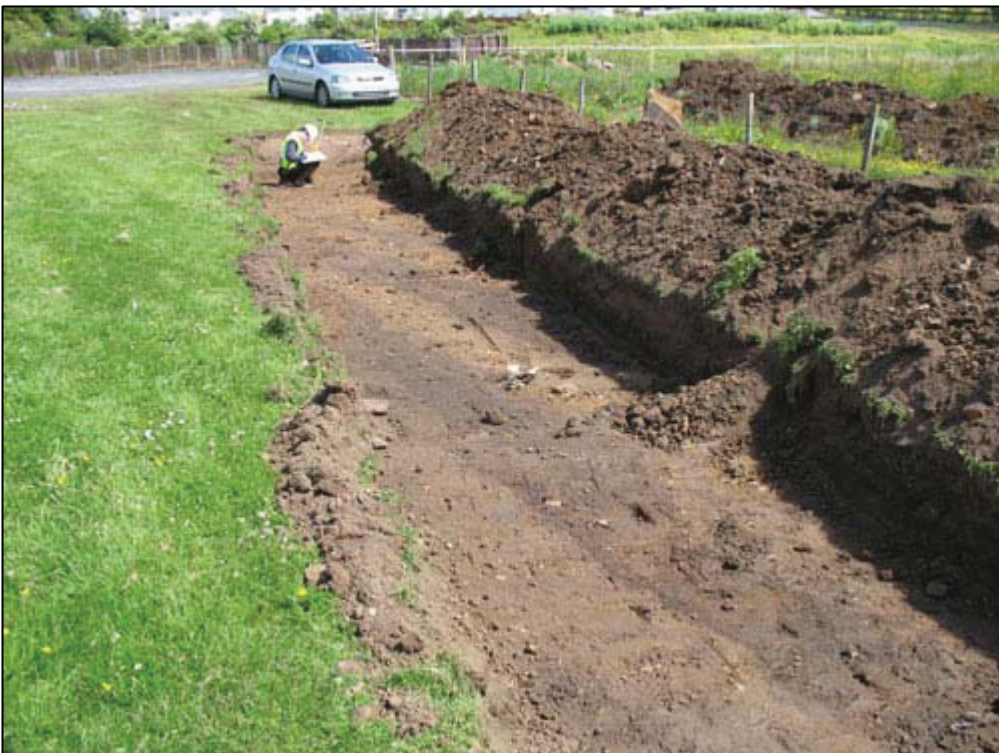
Figure 6b: Trench 24, showing (008), (009) and (010)
