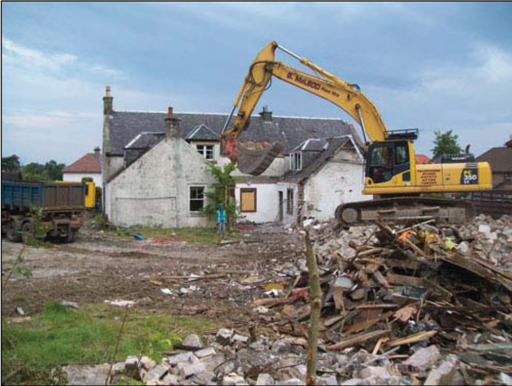
Figure 2a: Prior to demolition of main house
