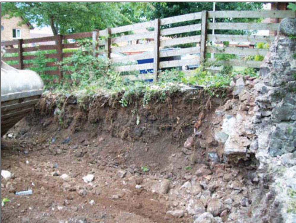
Figure 2b: Section in NE corner
