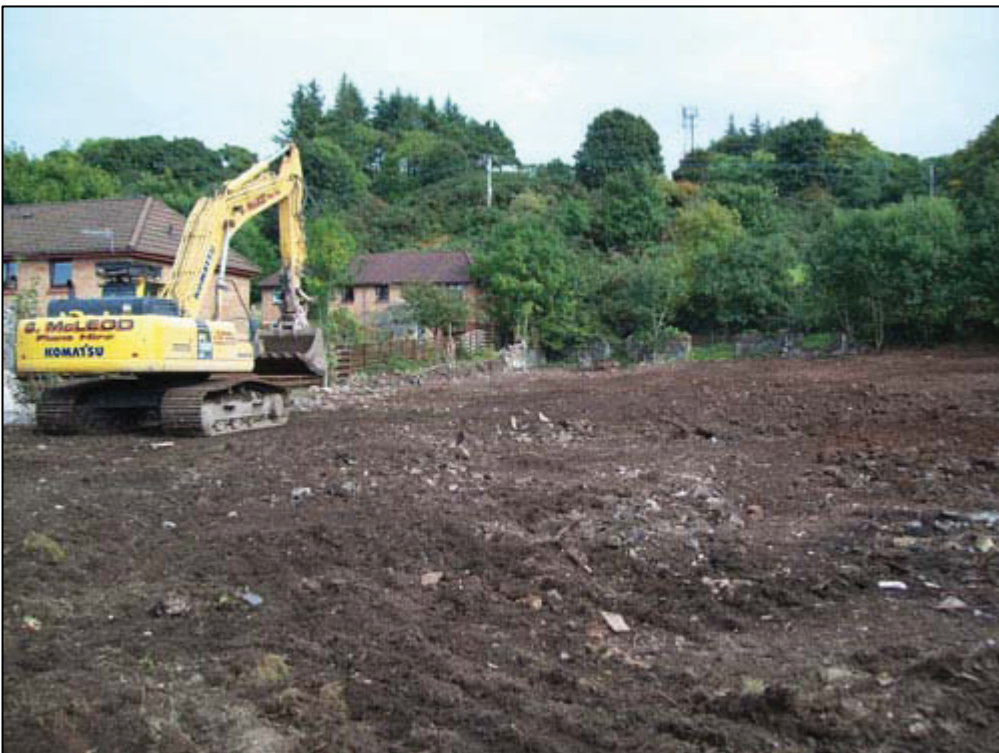
Figure 6b: Site after demolition work
