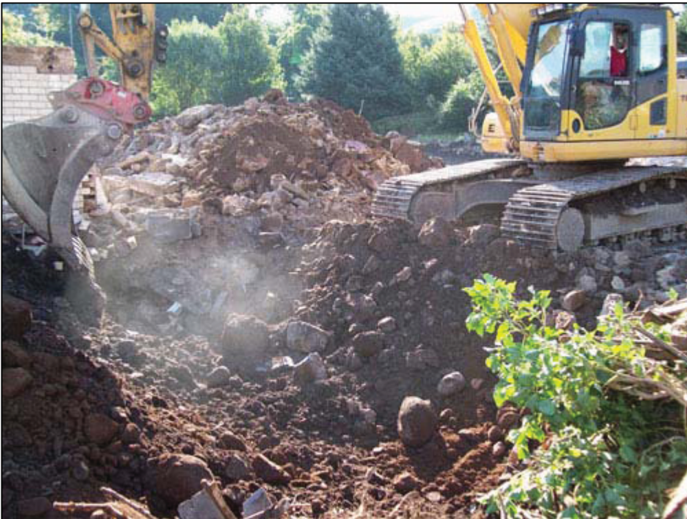
Figure 4b: Foundation removal in NW corner
