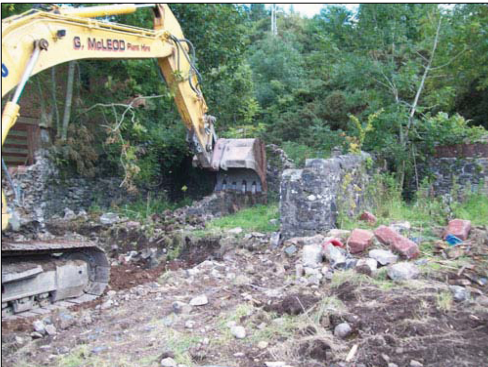
Figure 5b: Removing wall in NE corner
