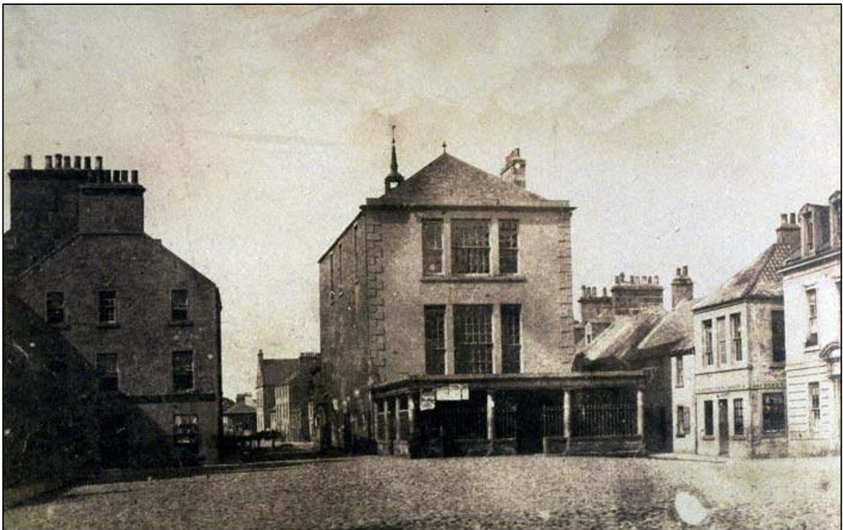
Figure 4: Image of last phase of Tolbooth structure (c.1850)
