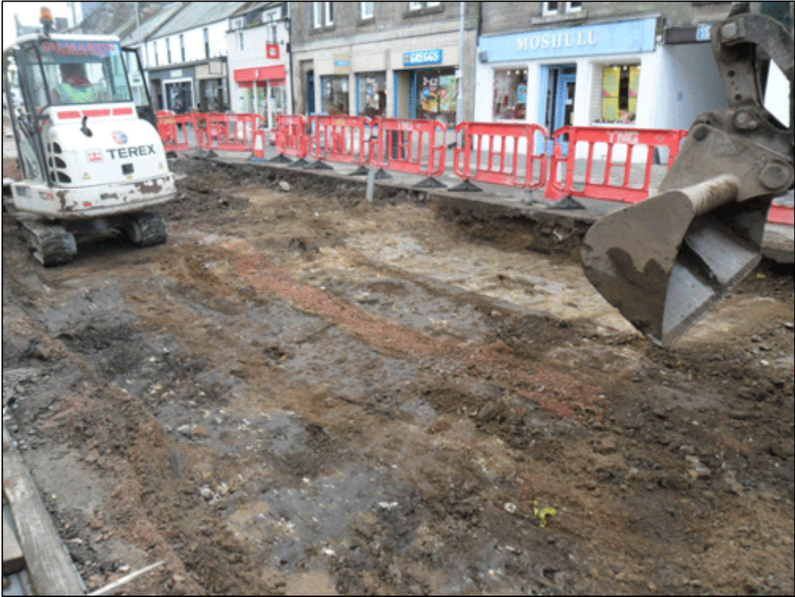
Figure 6: Reduction of Road 4 showing (070) to foreground
