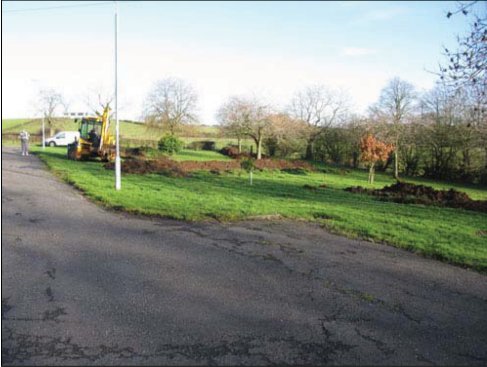
Figure 5a: Site after excavation
