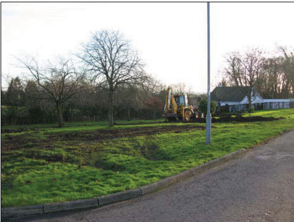
Figure 5b: Backfilling in progress
