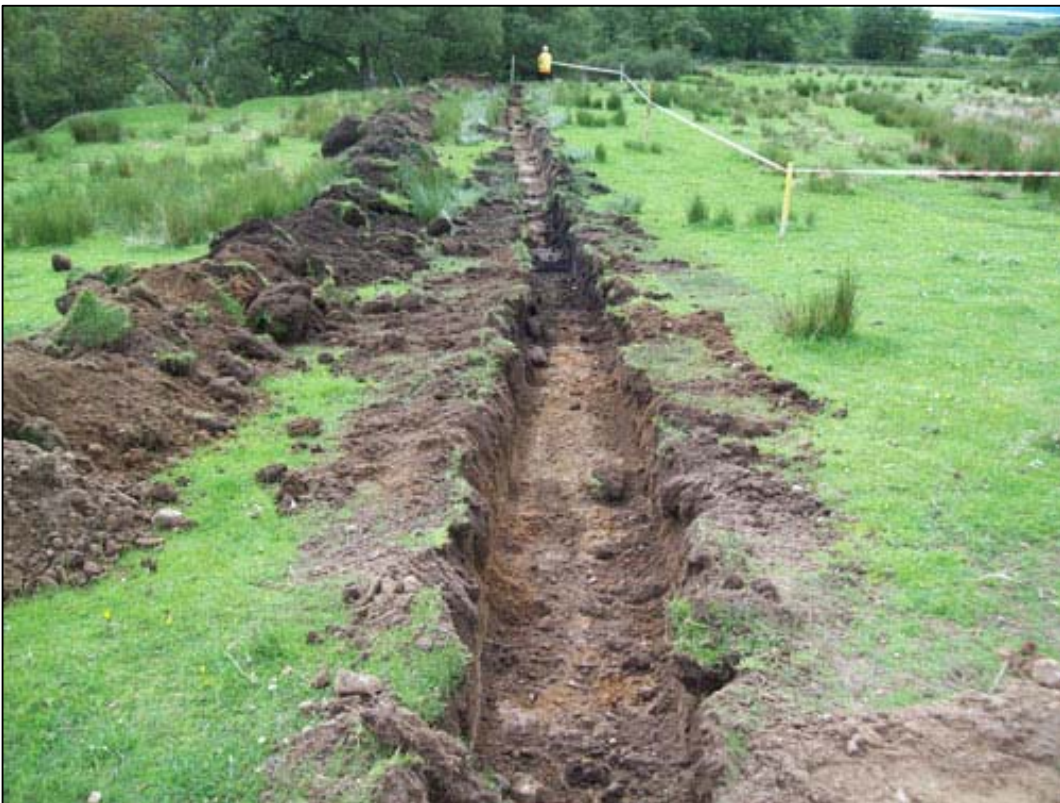
Figure 3b: Pipe Trench Spur from the East
