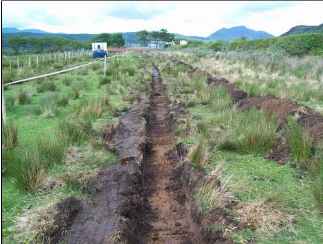
Figure 2b: Pipe Trench from South
