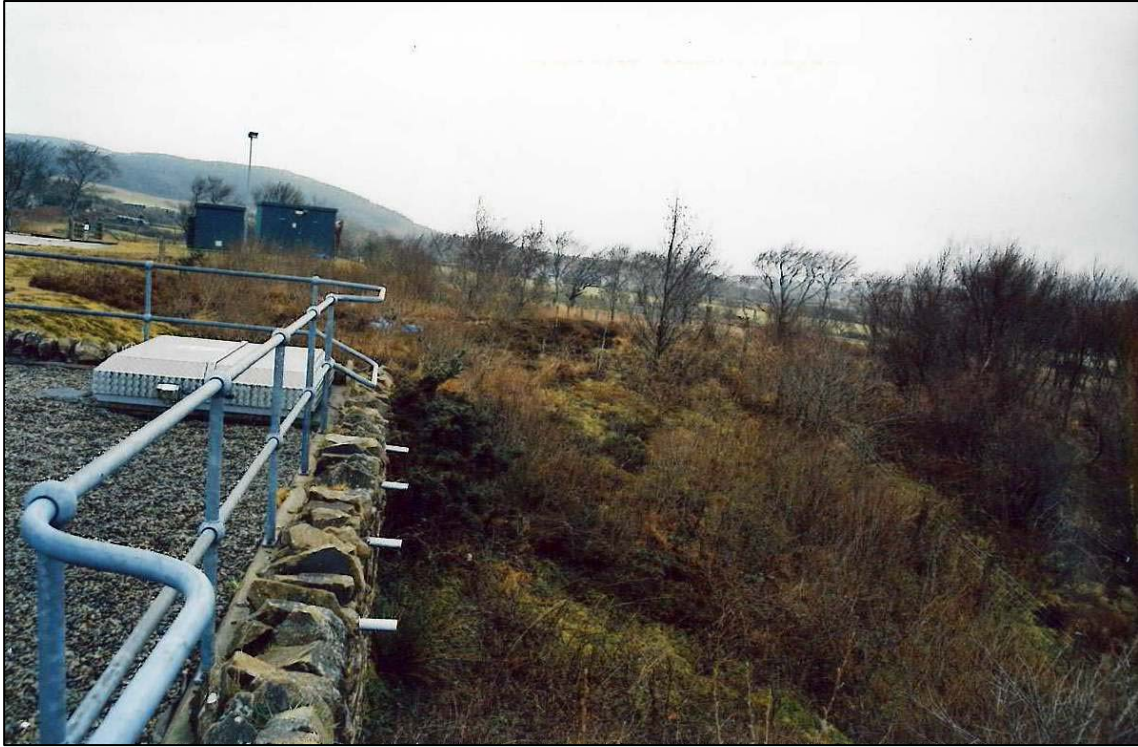
Figure 2a: NW Knoll at Balmichael WTW from the North
