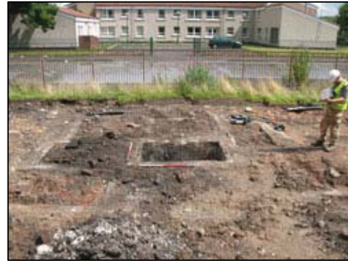
Figure 9h: Test Pit (206)
