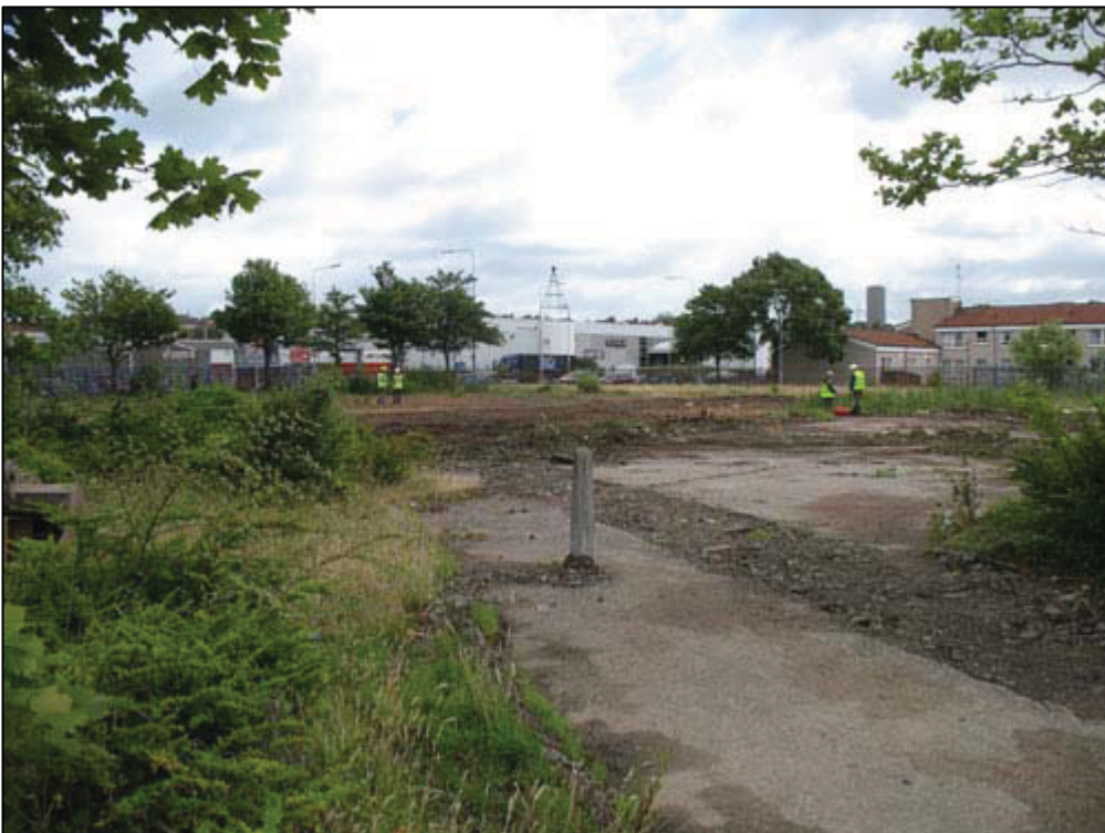
Figure 2b: Site prior to excavation
