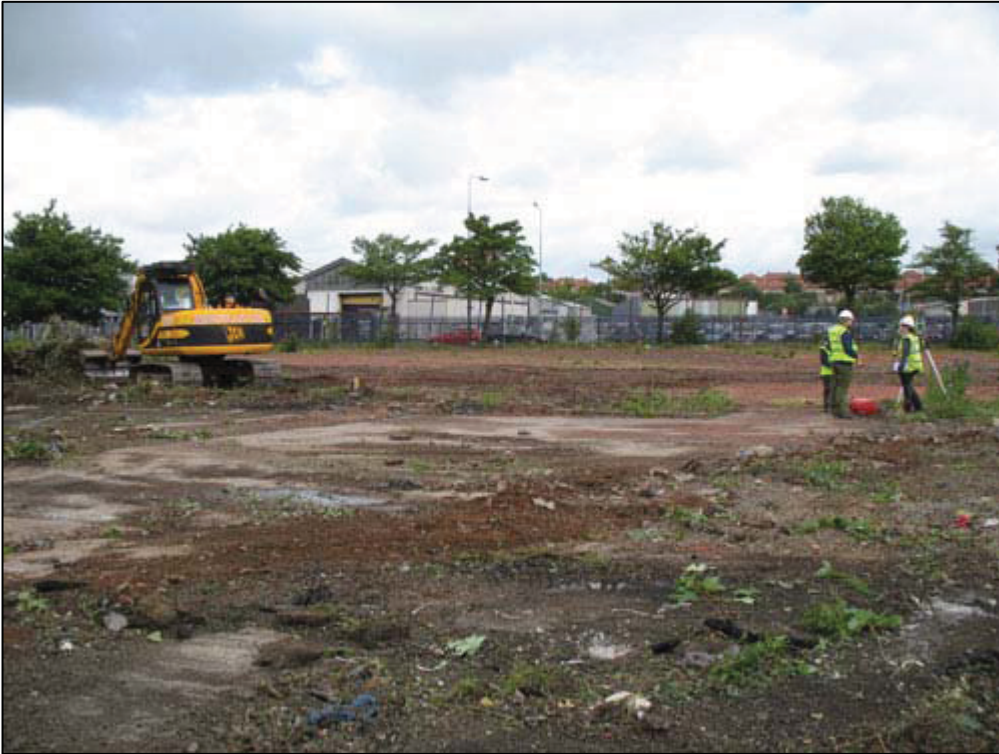
Figure 2a: Site after clearing trees.
