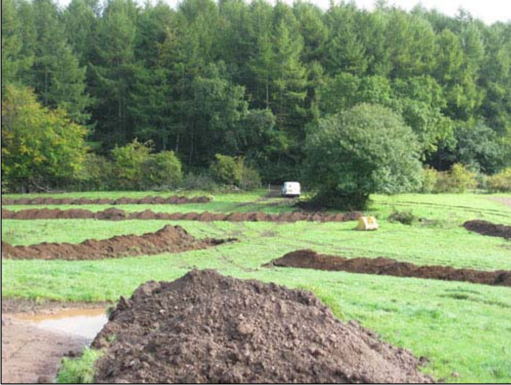
Figure 5a: Looking east to area of trees
