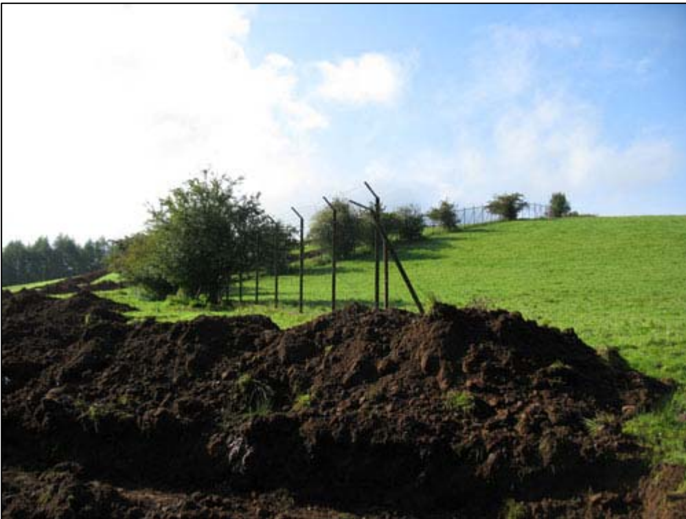
Figure 5b: Fence along northern site boundary
