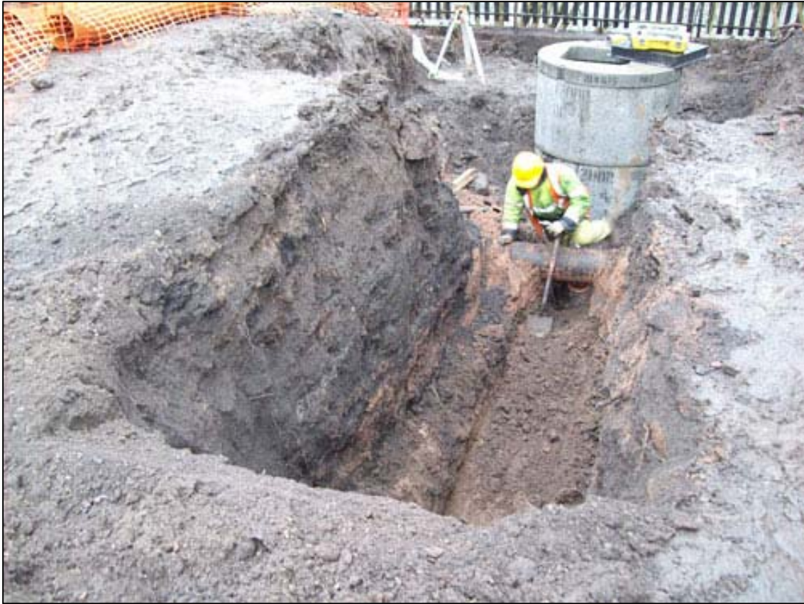
Figure 5a: Excavation beyond the gas pipe
