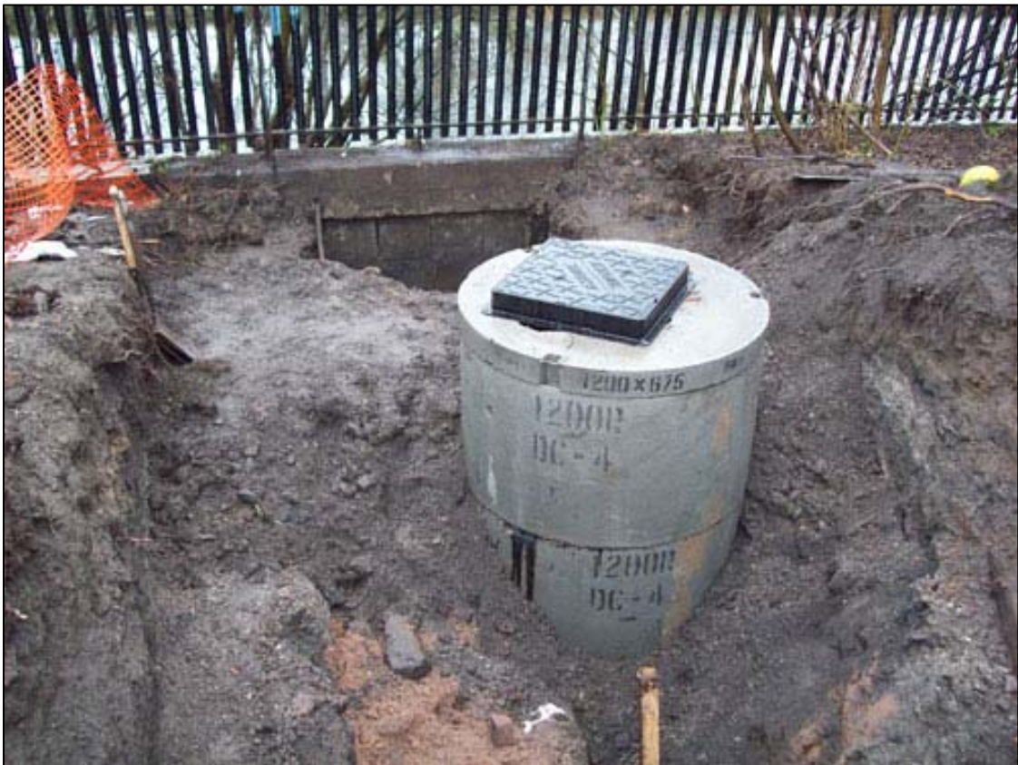
Figure 4b: Placement of manhole
