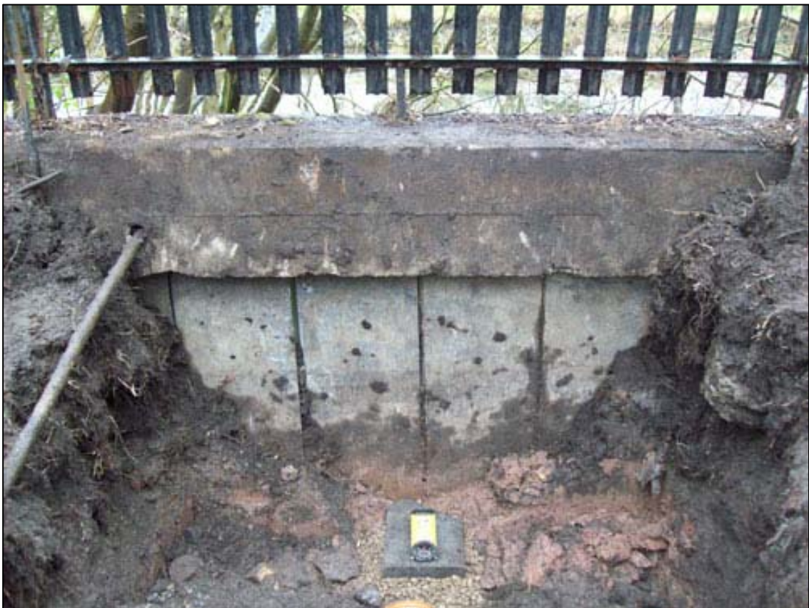
Figure 3b: Canal wall
