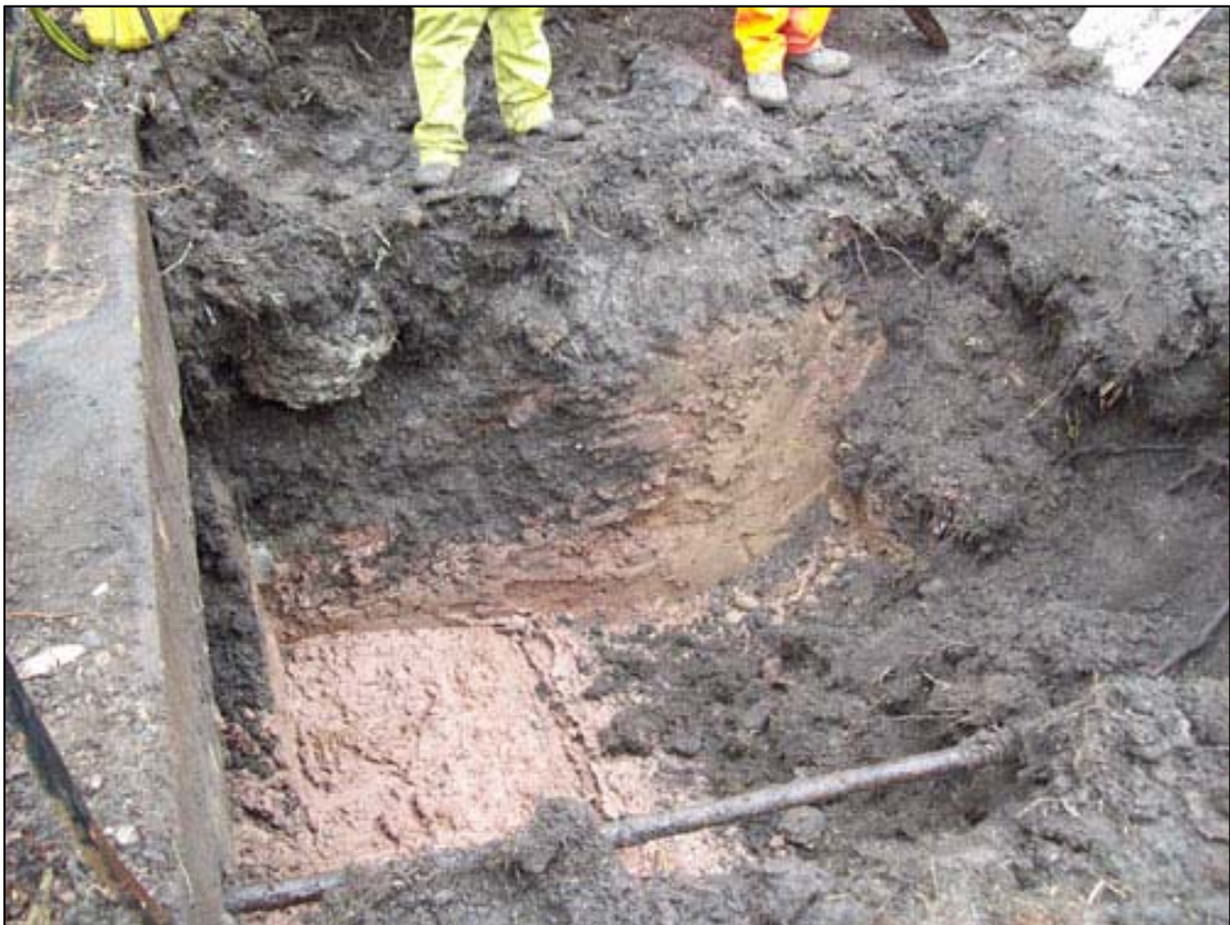
Figure 2b: Excavation close to the canal wall
