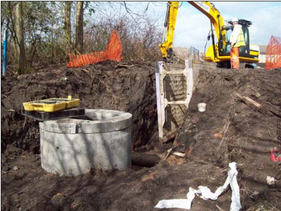
Figure 5b: Excavated area looking from the canal
