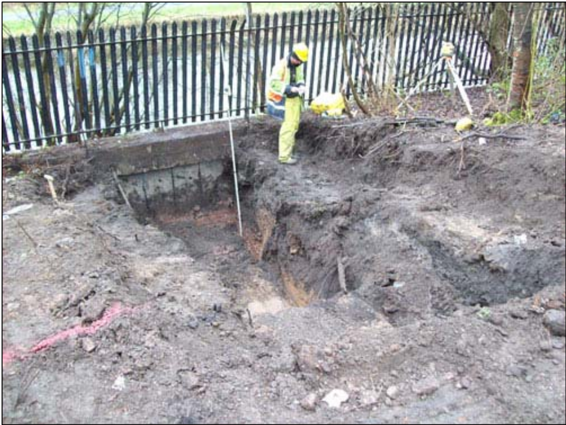
Figure 3a: Excavation extending away from the canal
