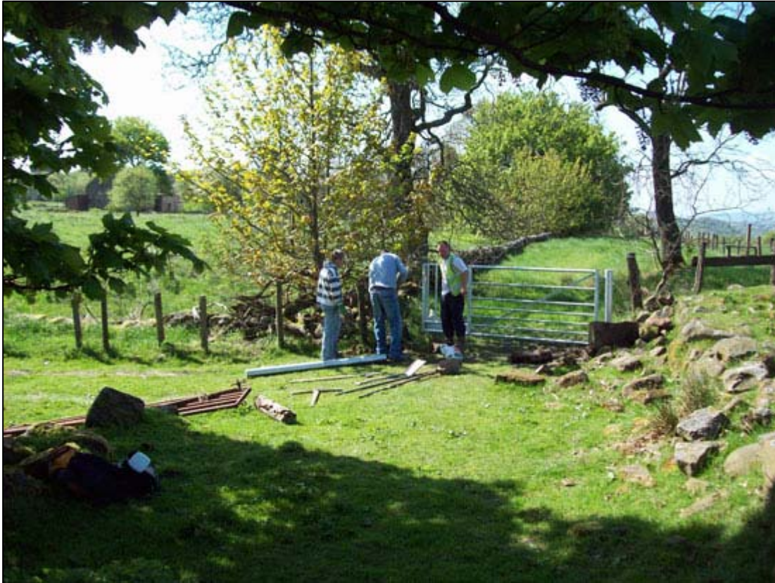
Figure 5a: New gate at Location 16
