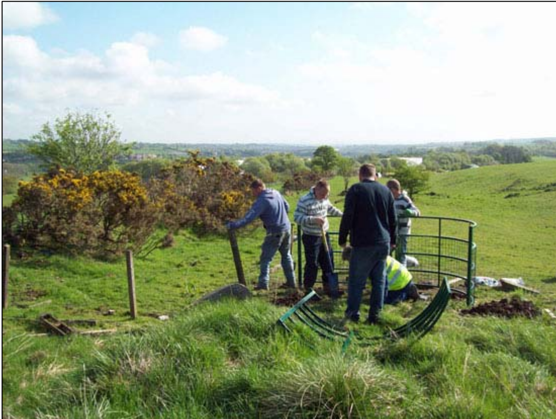
Figure 6a: New kissing gate at Location 31
