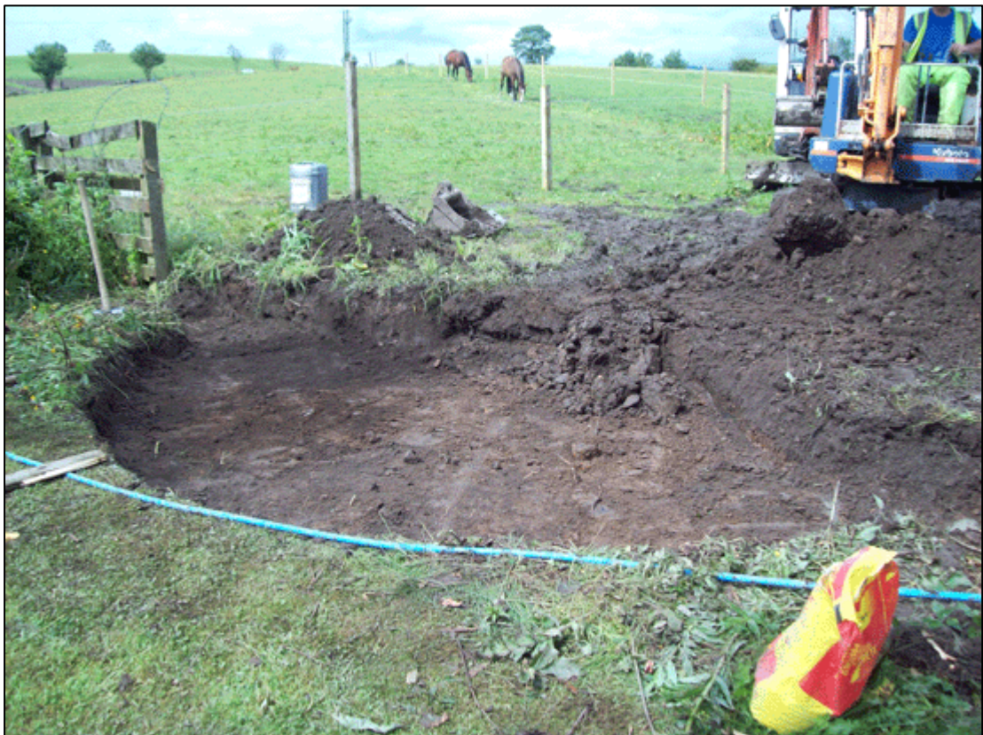
Figure 8b: Area stripped for new entrance gate at the location of ENT 2
