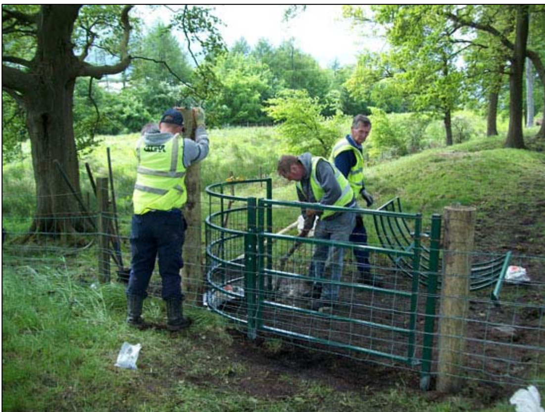
Figure 6b: New kissing gate at Location EX 2
