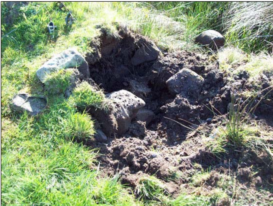
Figure 7b: Removal of fencepost at Location 26
