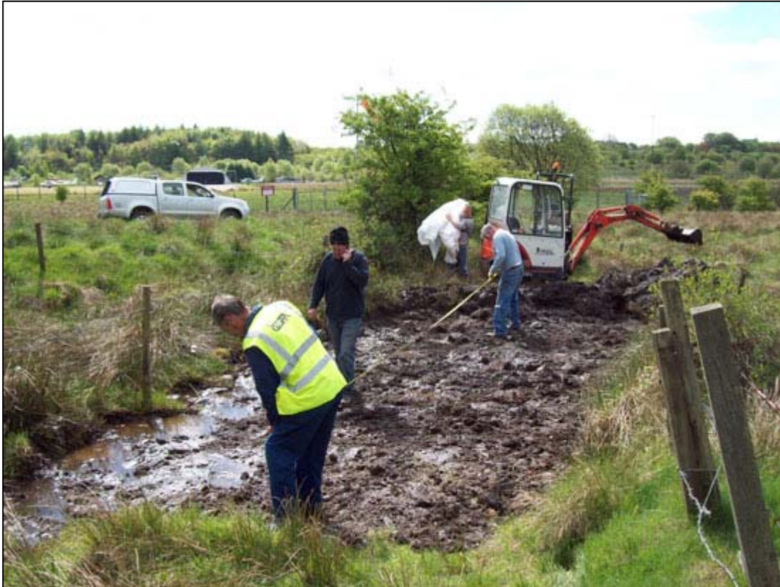
Figure 7a: Area of topsoil stripped at Location 25
