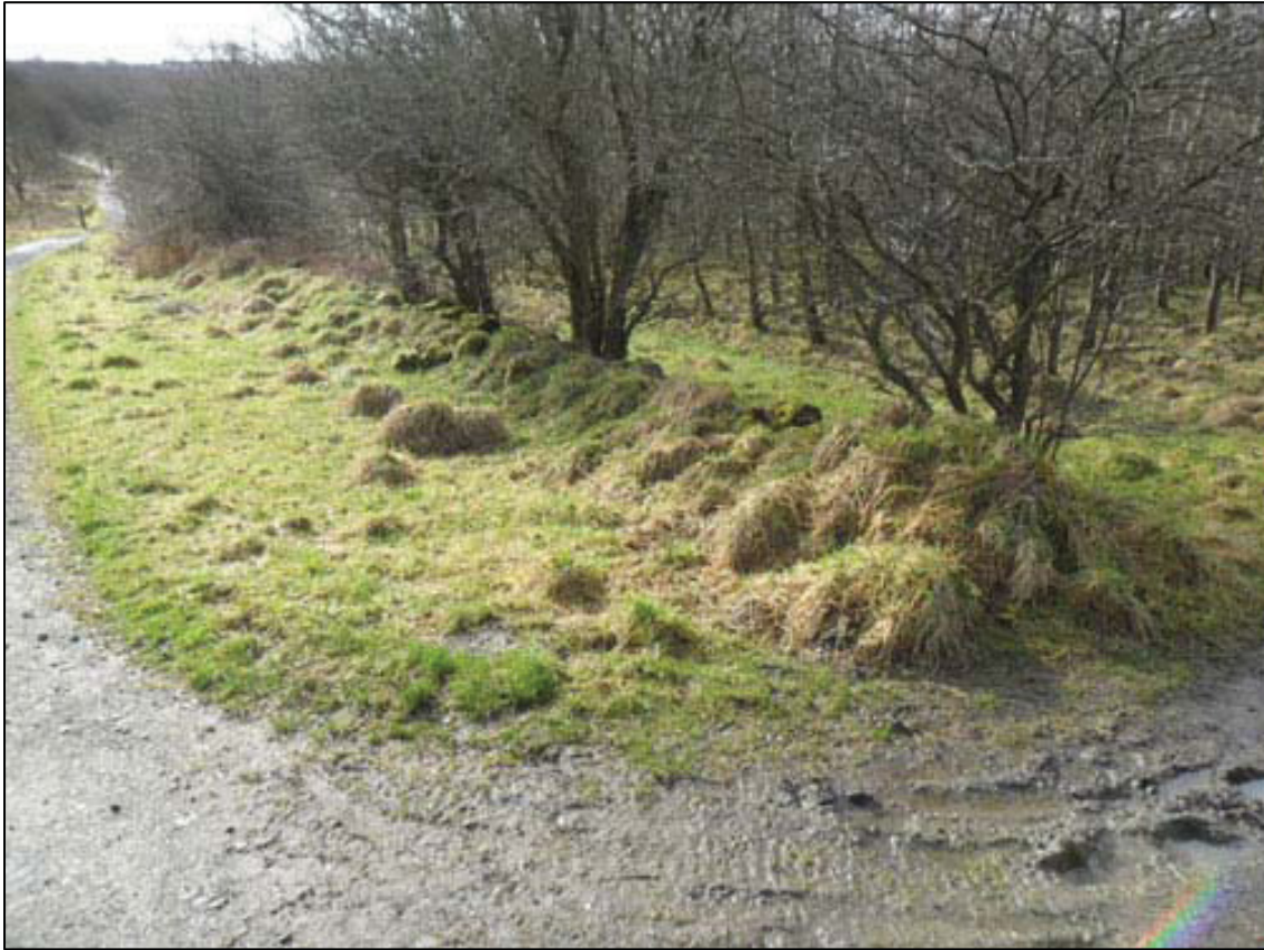
Figure 5a: Boundary wall ( RA11009b.03 )
