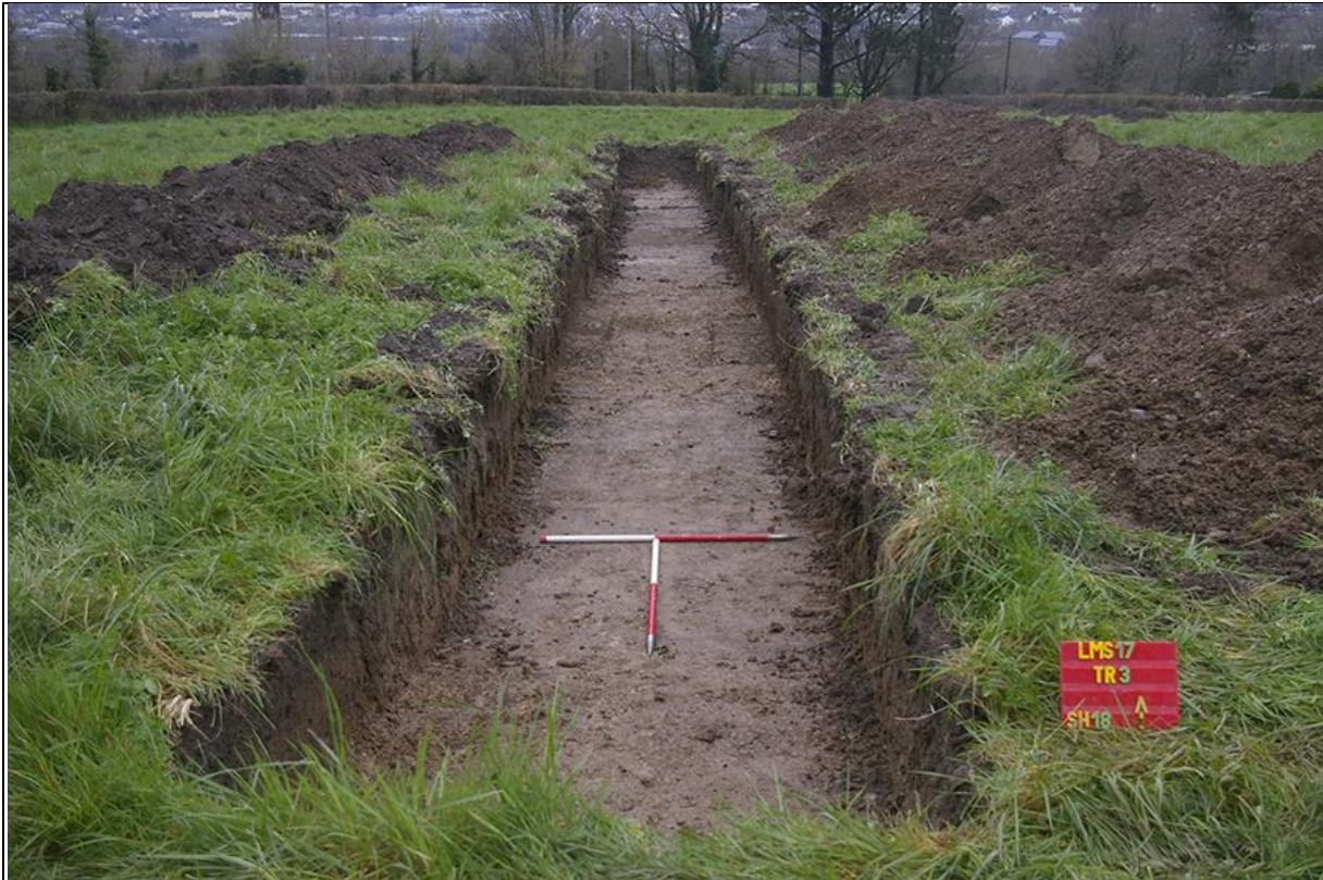
TRENCH 3 POST-EXCAVATION SHOT FROM THE SOUTH (2 x 1M SCALES).
