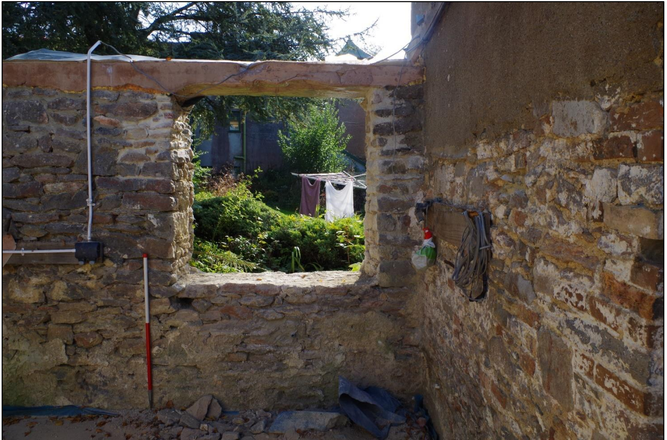
47. UNBLOCKED WINDOW OPENING (BW5) IN ROOM BS3C, VIEWED FROM THE WEST (1M SCALE).
