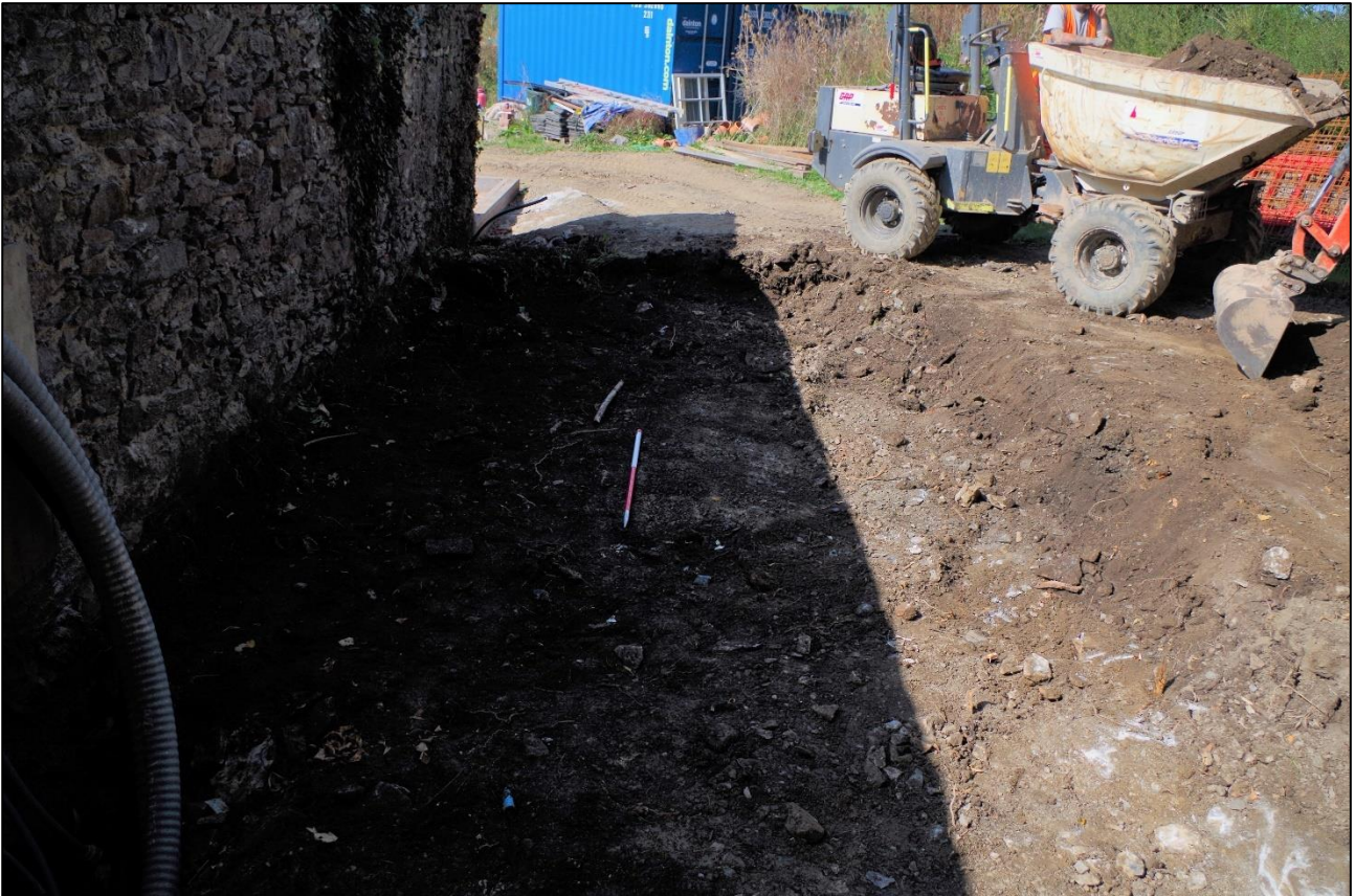
51. AREA TO NORTH OF THE GARAGES, POST-EXCAVATION (1M SCALE).
