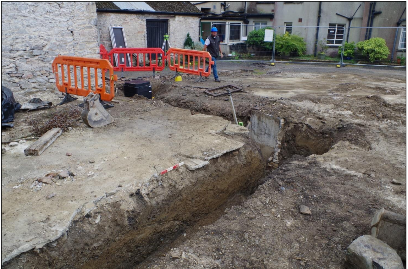
44. FOOTING TRENCHES, VIEWED FROM THE NORTH-WEST (0.4M SCALE).
