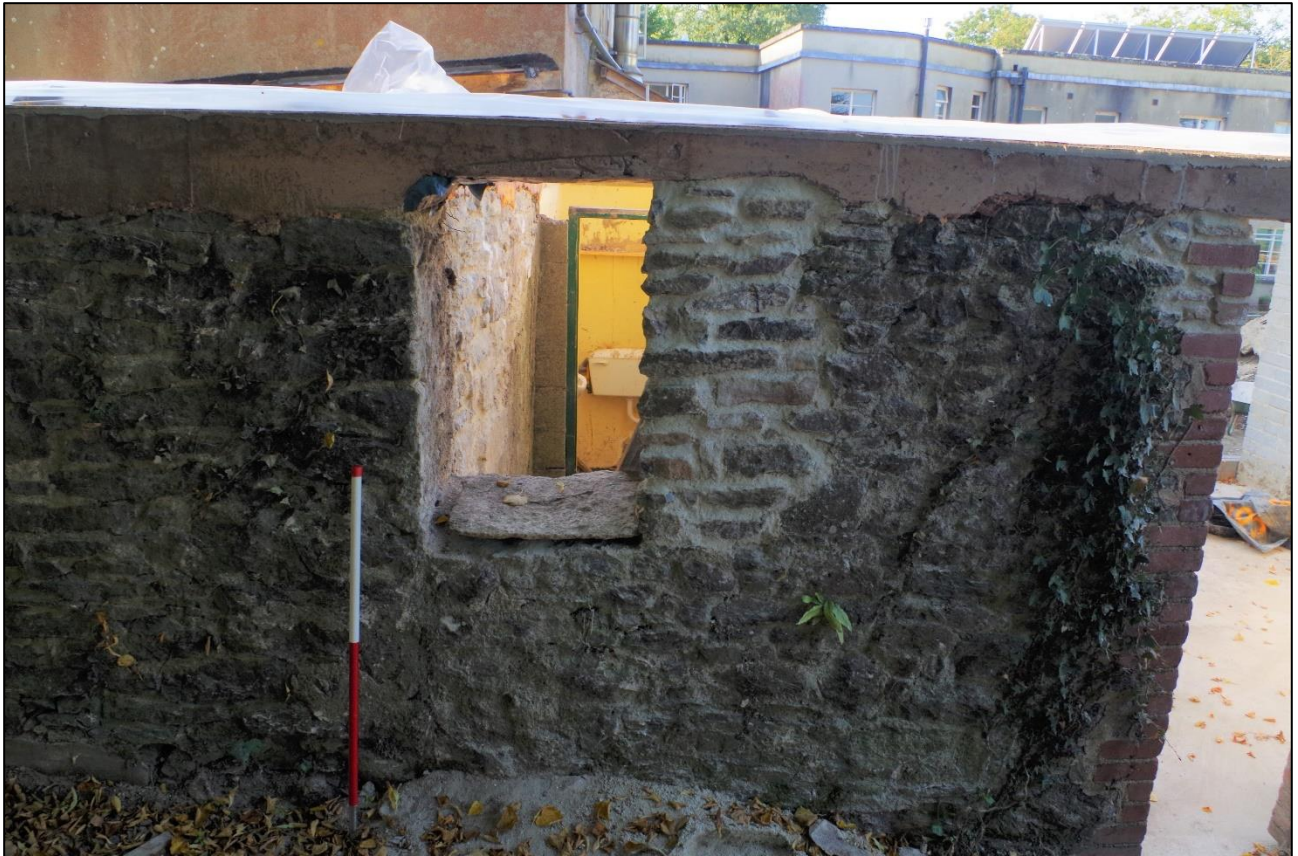
49. OPENING UP OF PART OF BLOCKED WINDOW (BW6), FROM THE NORTH (1M SCALE).
