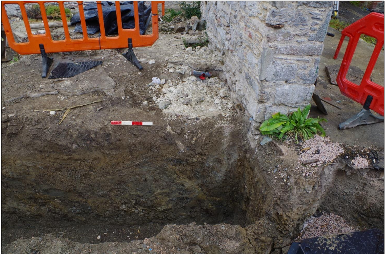
45. FOUNDATION TRENCH CUT FOR WALL {111}; VIEWED FROM THE SOUTH (0.4M SCALE).
