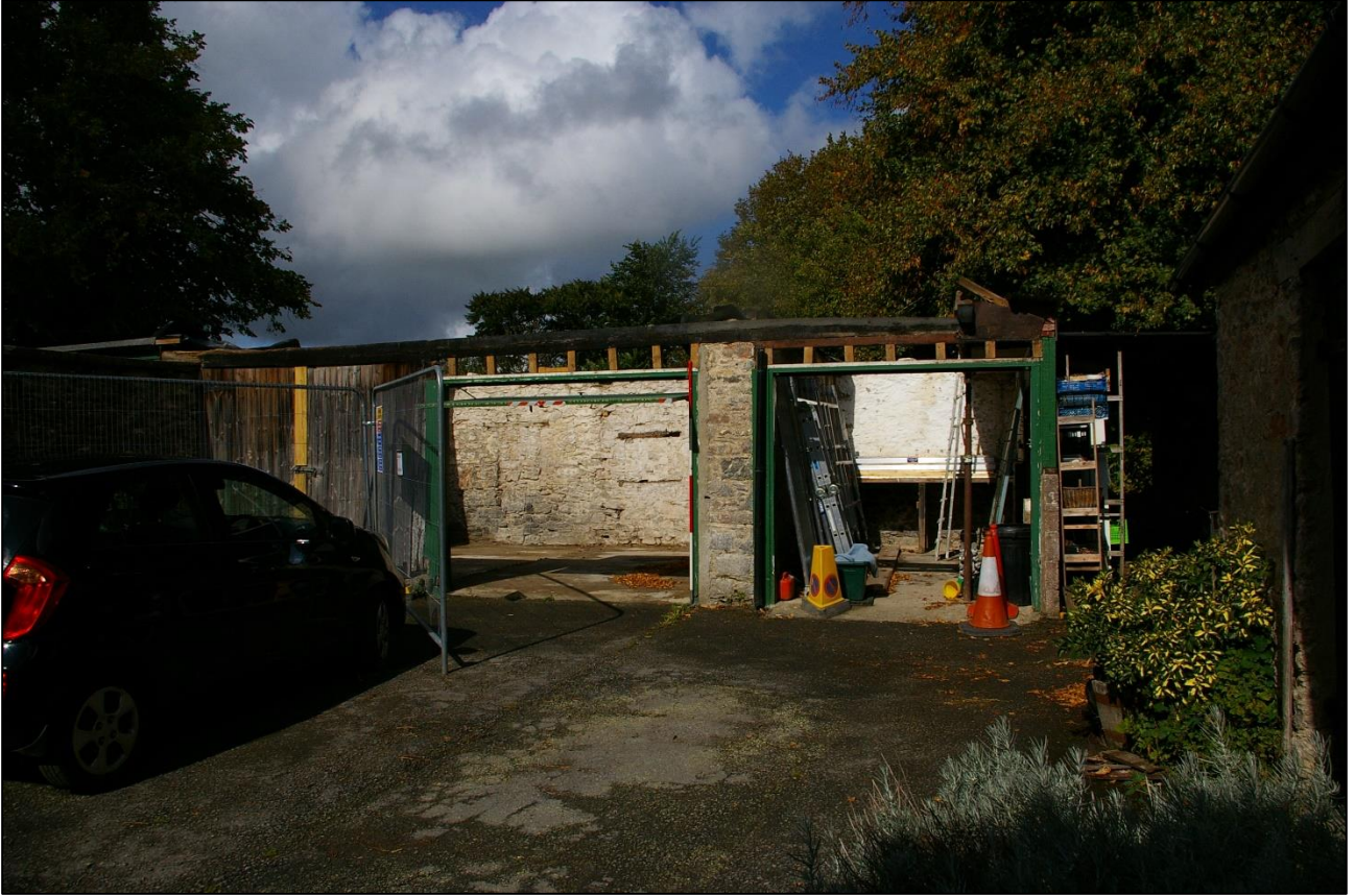
1. THE SOUTH ELEVATION OF B2, WITH 2M SCALE; FROM THE SOUTH.
