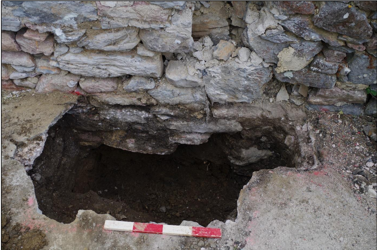
FIGURE 4: UNDERPINNING PIT 1, VIEWED FROM THE WEST (0.4M SCALE).
