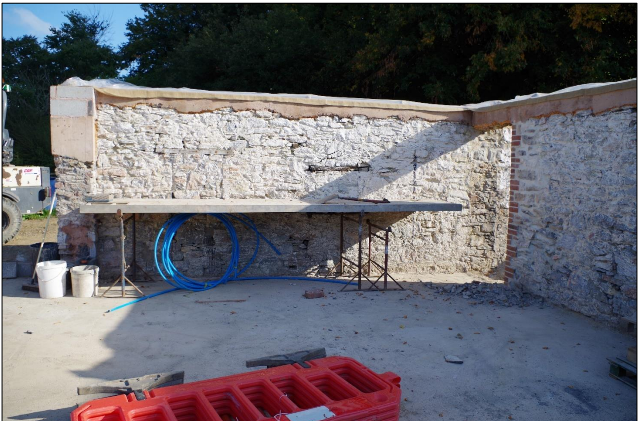
48. ROOM B2A FOLLOWING COMPLETION OF GROUNDWORKS, FROM THE SOUTH (NO SCALE).
