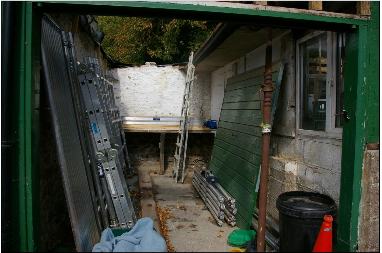
41. B2B, USED AS A WORKSHOP, FROM THE SOUTH-SOUTH-WEST (2M SCALE).
