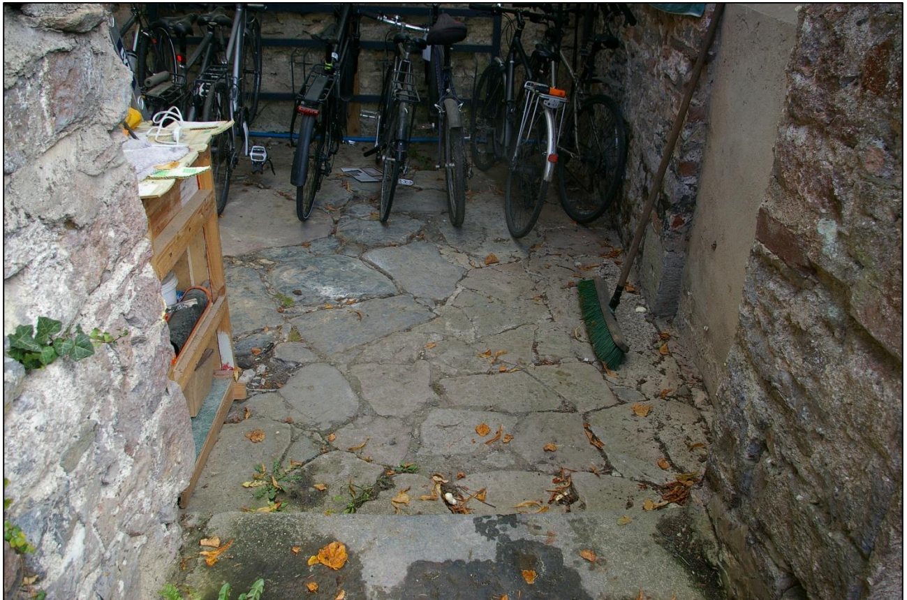
4. THE FLAGSTONE FLOOR IN B3C; FROM THE WEST.
