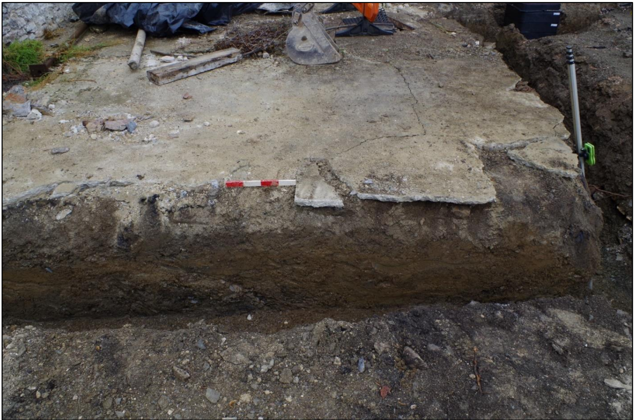
FIGURE 6: WEST FACING SECTION OF FOOTING TRENCH, ALONG LINE OF DEMOLISHED WALL {110}, FROM THE WEST (0.4M SCALE).
