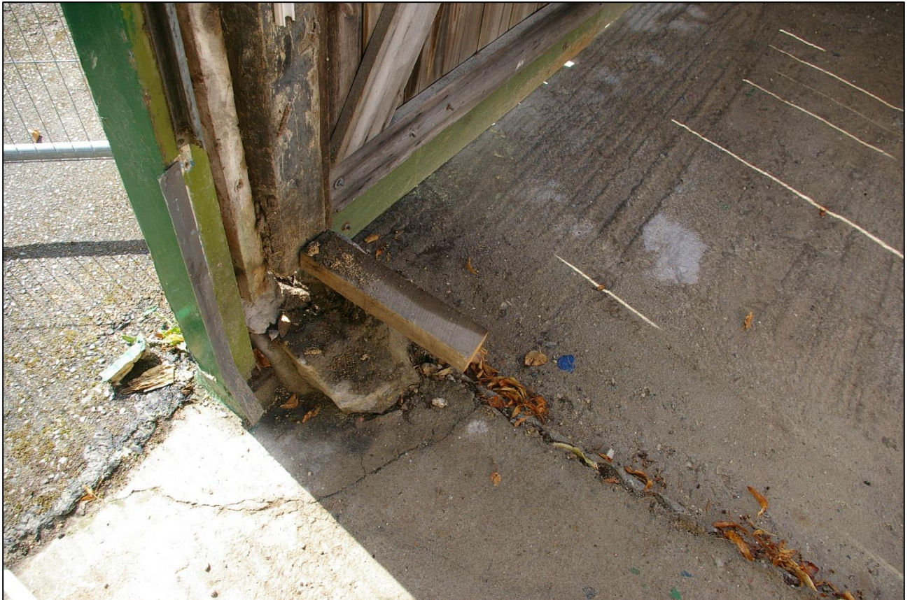
28. THE STUB OF RUBBLE WALLING INDICATING THE POSITION OF A FORMER PARTITION WALL; FROM THE NORTH-EAST.
