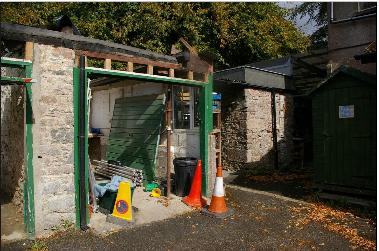
2. THE SOUTH ELEVATION OF B3; FROM THE SOUTH-WEST.
