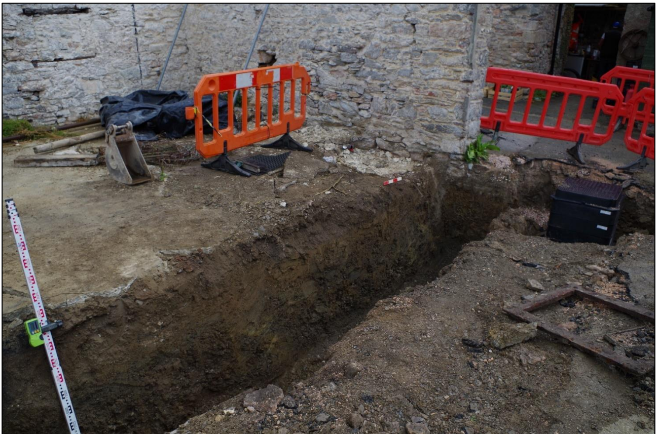
46. SOUTHERN FOOTING TRENCH, VIEWED FROM THE SOUTH-WEST (0.4M SCALE).
