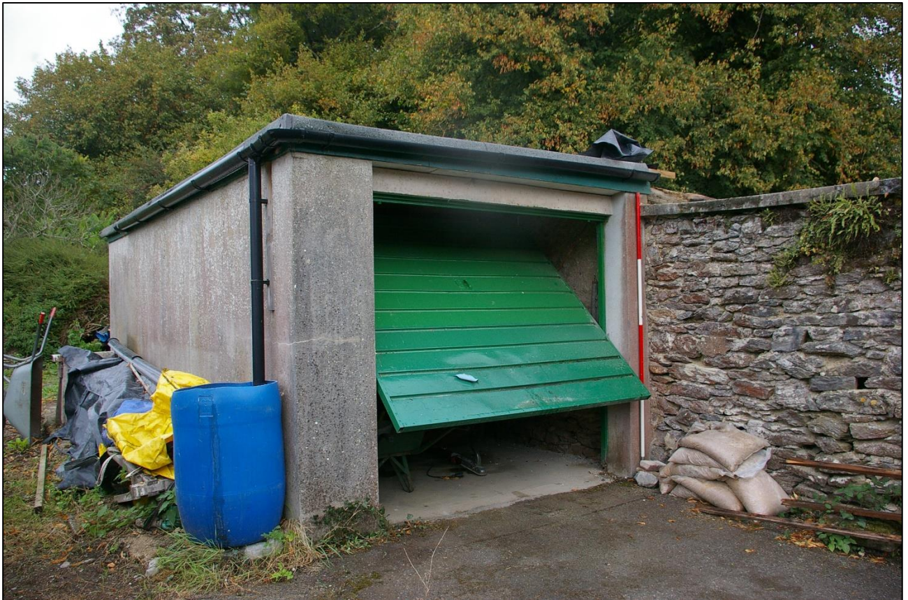
21. THE SOUTH AND WEST WALLS OF B1, SHOWING HOW IT ABUTS THE WEST WALL OF B2; FROM THE SOUTH-WEST (2M SCALE).
