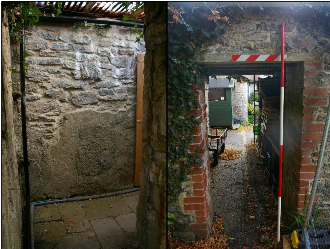
13. LEFT: THE EAST WALL OF B3B, SHOWING PART RENDER PLASTER AND POSSIBLE BLOCKINGS; FROM THE WEST-NORTH-WEST.
