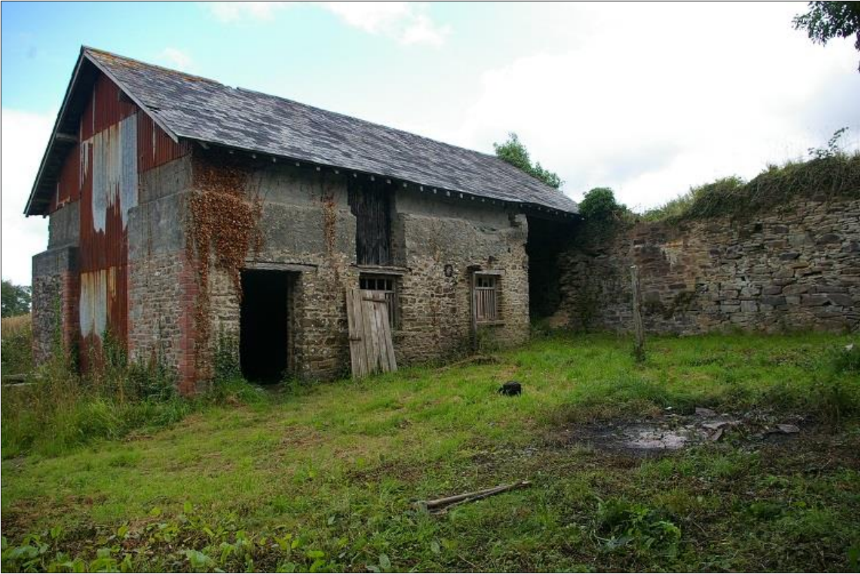
1. THE COMPLEX FROM THE SOUTH-WEST.
