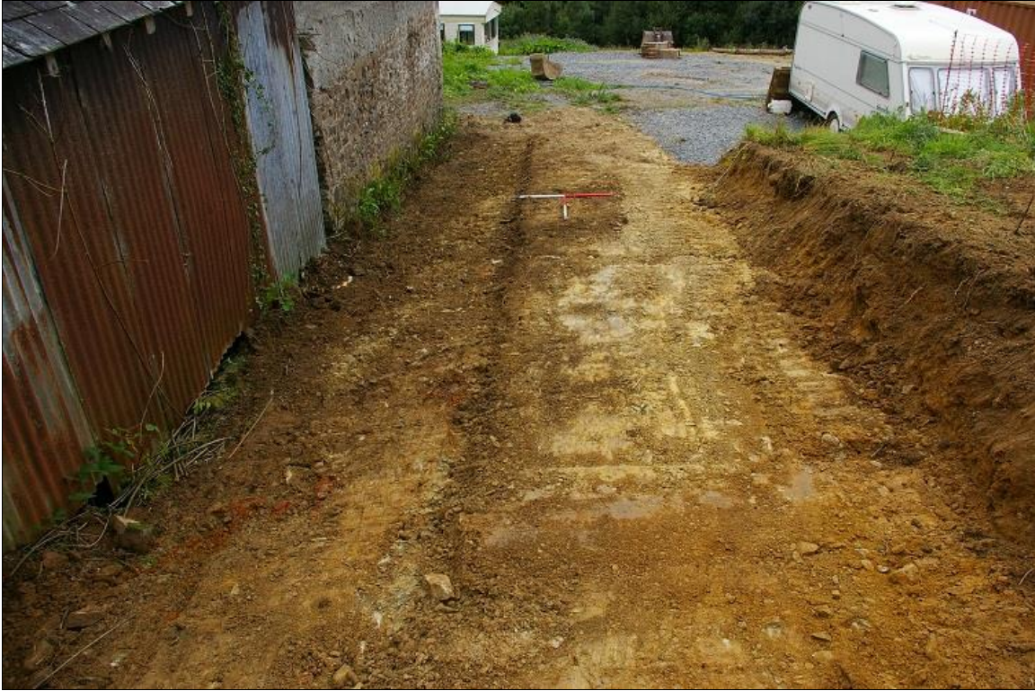
15. VIEW BACK ALONG THE NORTH ELEVATION, (2 X 1M SCALES); FROM THE EAST.
