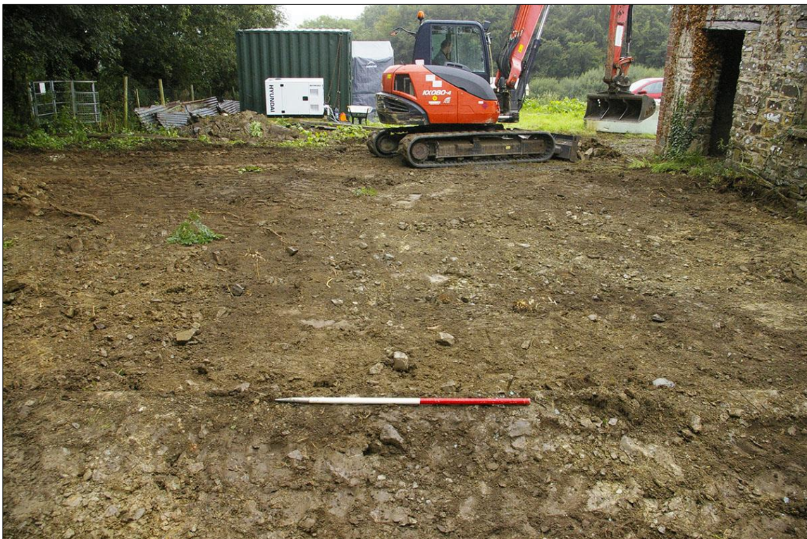
37. STRIPPED YARD AREA; FROM THE SOUTH-EAST (1M SCALE).
