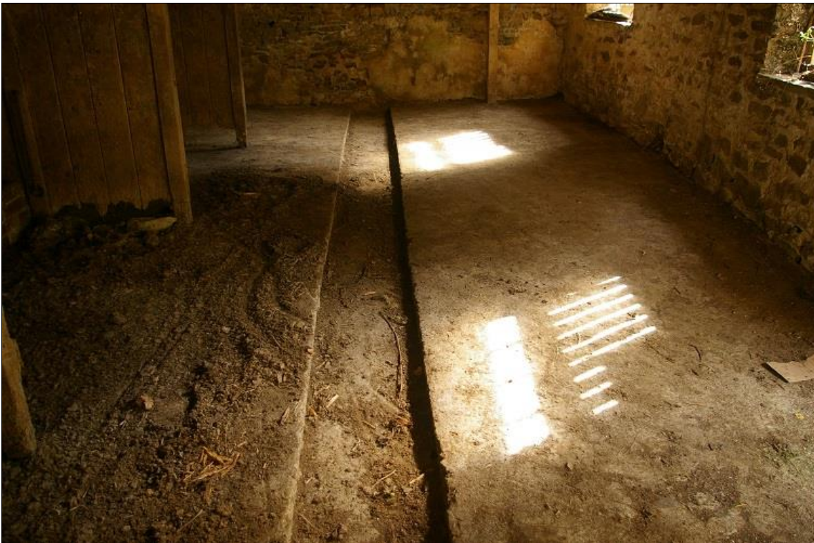
18. THE CONCRETE FLOOR, COVERING AN OLDER COBBLED FLOOR AND DRAIN; FROM THE WEST.
