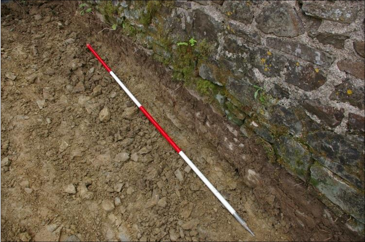
13. THE BASE OF THE NORTH WALL OF THE BARN, BUILT ONTO THE ROCKY SUBSOIL AND SHILLET (2M SCALE); FROM THE WEST-NORTH-WEST.
