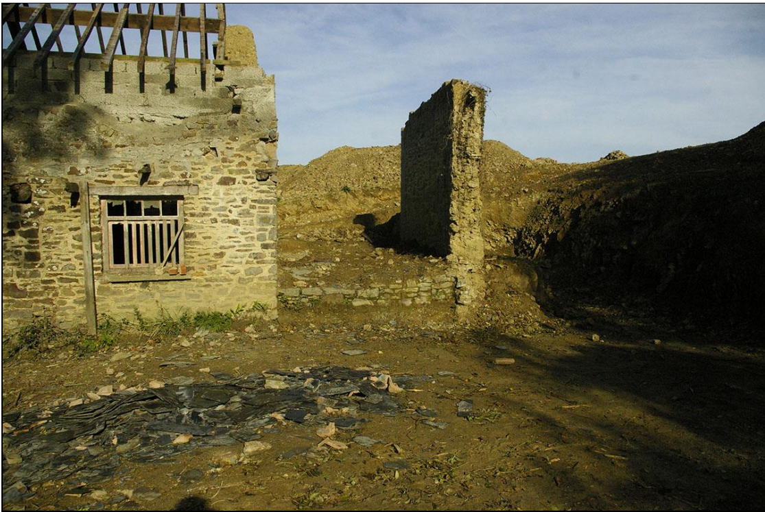
43. EAST WALL AND STANDING RANGE; FROM THE SOUTH.
