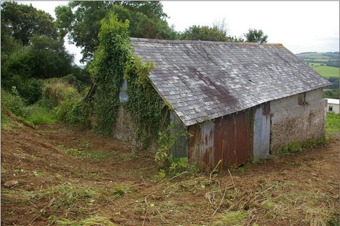
5. THE BUILDING COMPLEX, VIEWED FROM THE NORTH-EAST, WITH FOLIAGE REMOVED.
