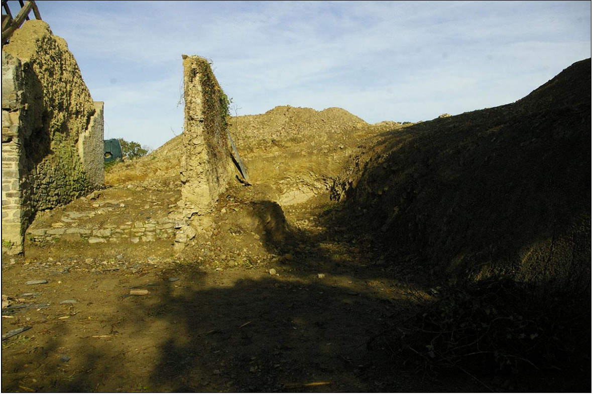
42. THE EAST END OF THE STANDING RANGE, SHOWING IT IS BUILT ONTO THE BEDROCK, WHICH HAS BEEN UNDERCUT FOR FOUNDATIONS AND DRAINAGE; FROM THE SOUTH.
