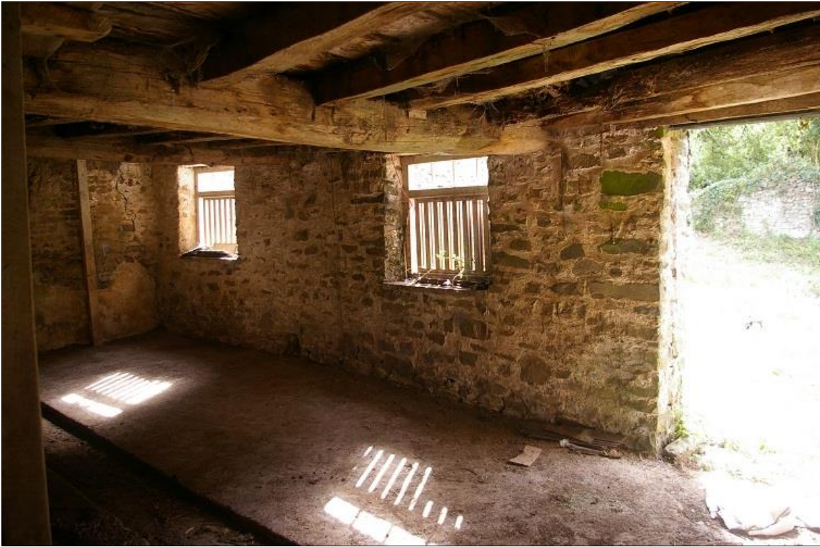
17. THE INTERIOR OF THE BARN, SOUTH WALL; FROM THE NORTH-WEST.
