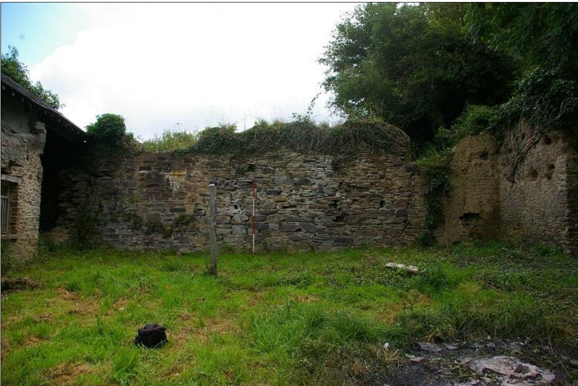
10. THE EAST WALL, LINKING THE EARLIER COB RANGES (2M SCALE); FROM THE WEST.
