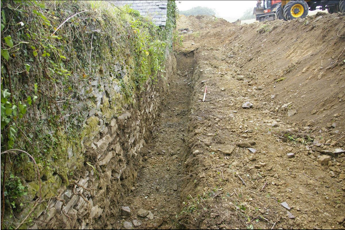
26. VIEW ALONG THE TRENCH, SHOWING THE WALL IS MERELY BUILT ON SUBSOIL ABOVE THE BEDROCK, WITH NO DEFINED FOUNDATIONS, WITH 1M SCALE; FROM THE SOUTH-SOUTH-EAST.
