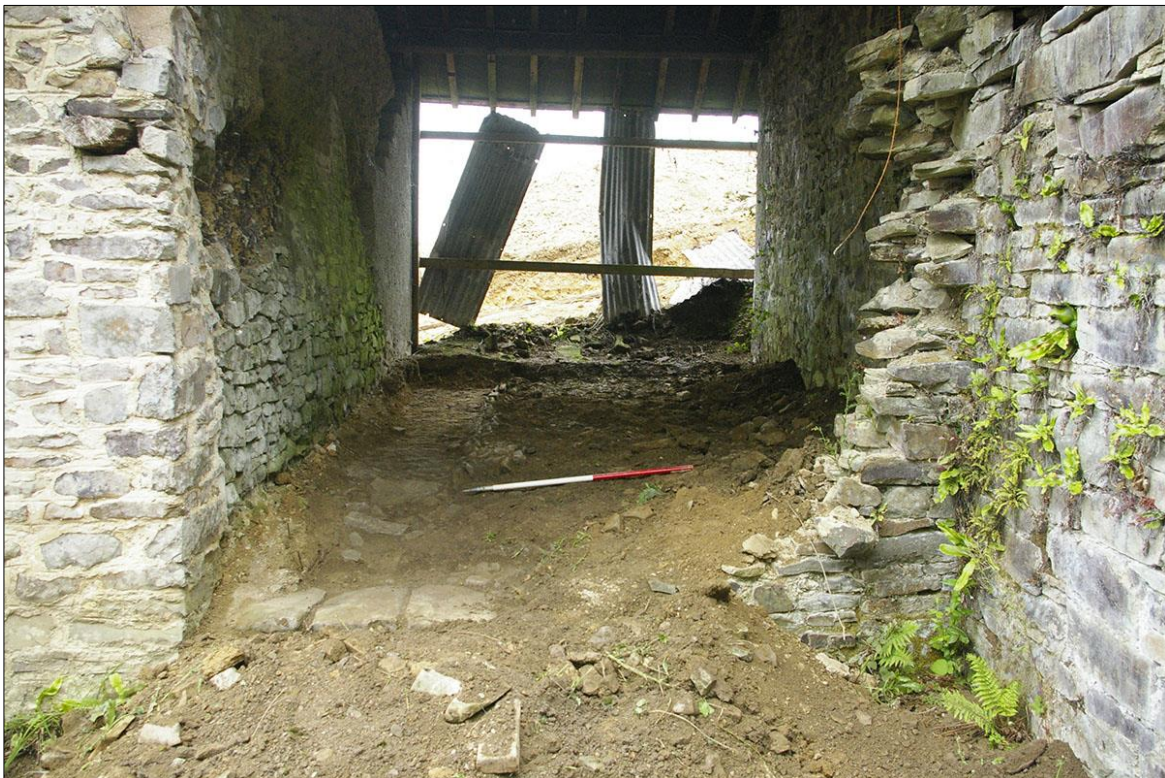
35. BARN ROOM WITH COBBLES (104); FROM THE SOUTH-WEST (1M SCALE).
