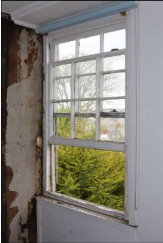
LEFT FIGURE 21: R9, THE RESET EARLY C19 SASH WINDOW; VIEWED FROM THE SOUTH-EAST.
