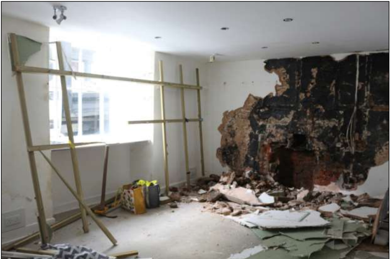
FIGURE 14: R1, VIEWED FROM THE NORTH-EAST.
