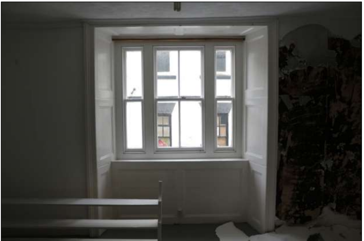
FIGURE 16: R7, AS ABOVE; VIEWED FROM THE NORTH.
