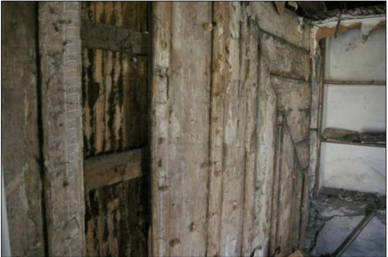
FIGURE 24: R10, DETAIL OF THE VERTICAL PLANK BOARDING; VIEWED FROM THE NORTH.
