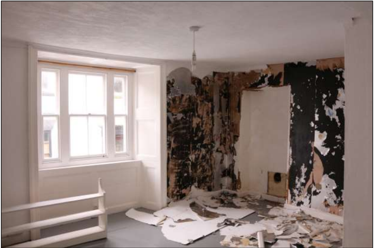
FIGURE 17: R7, VIEWED FROM THE NORTH-EAST.
