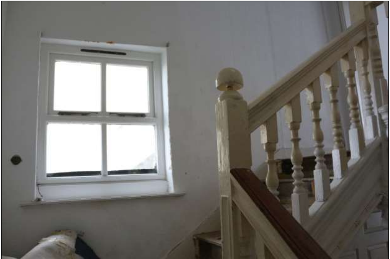
FIGURE 31: R2, THE STAIRS, SHOWING THE NEWEL AND BALUSTERS AT THE SECOND HALF LANDING; VIEWED FROM THE WEST.
