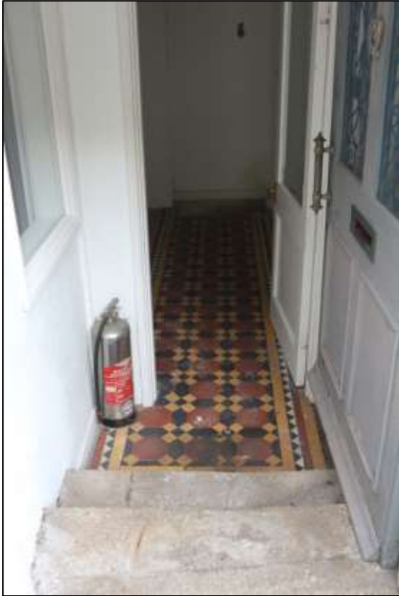
FIGURE 13: THE POLYCHROMATIC GEOMETRIC TILED FLOOR IN THE LATE C19 PASSAGE; VIEWED FROM THE SOUTH.
