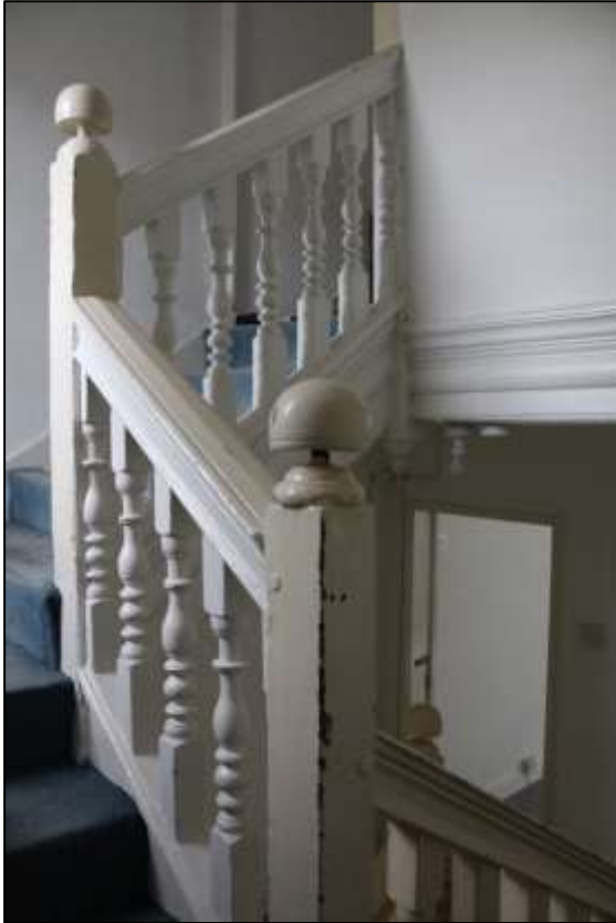
LEFT FIGURE 37: R8, DETAIL OF THE UPPER NEWELS (UNDECORATED) AND BALUSTERS; VIEWED FROM THE NORTH-EAST.
