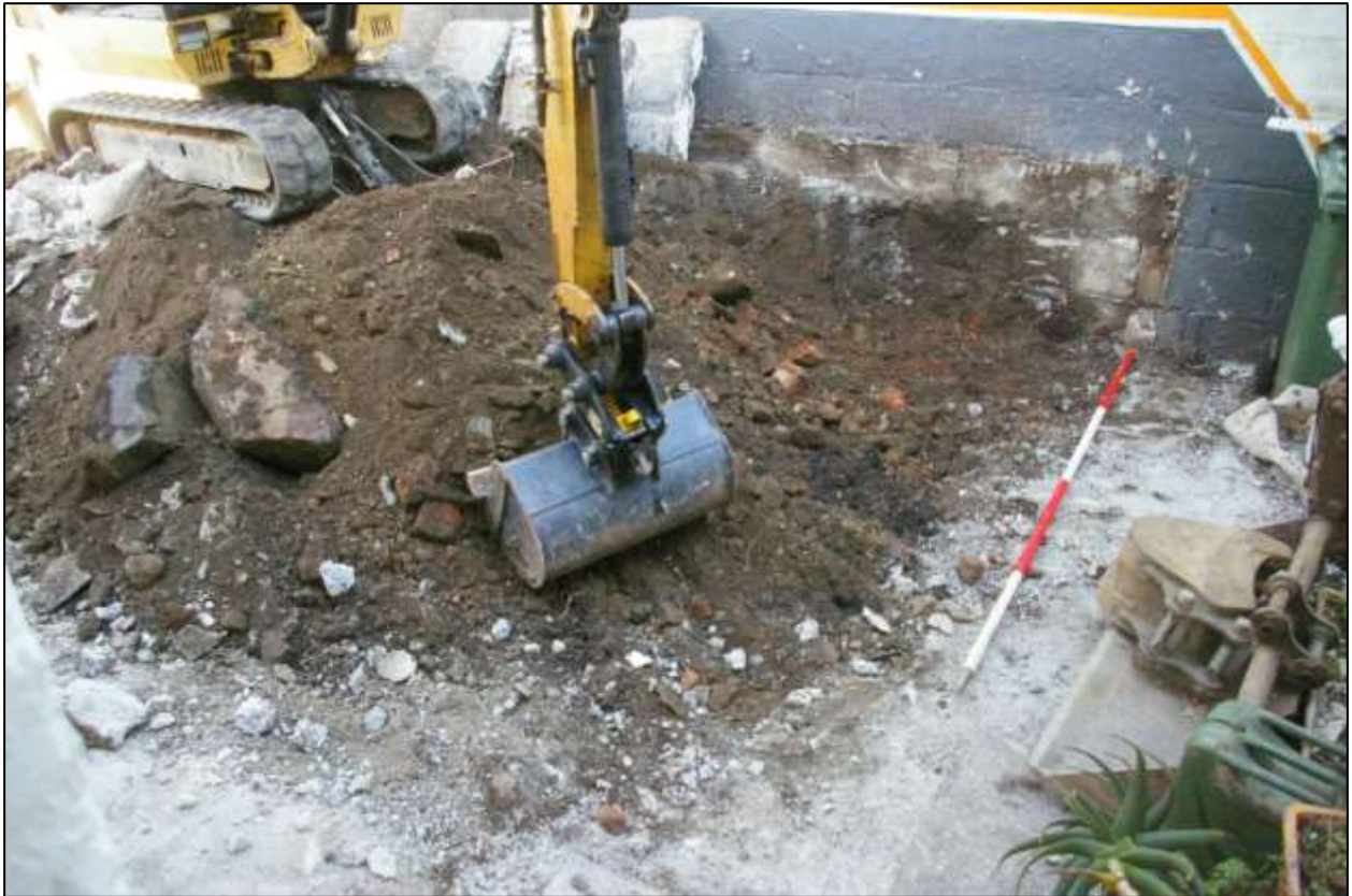
FIGURE 6: THE PATIO AREA UNDER EXCAVATION; VIEWED FROM THE EAST (SCALE 2M).
