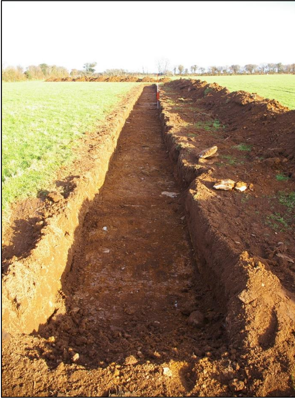
1. LEFT: TRENCH #1; VIEWED FROM THE WEST (SCALE 2M).
