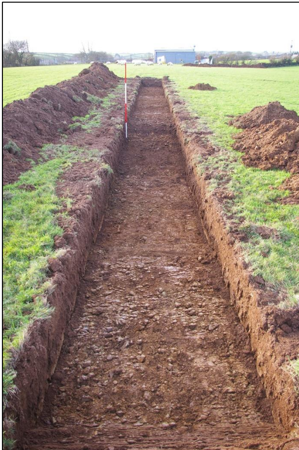
25. LEFT: TRENCH #5; VIEWED FROM THE EAST (SCALE 2M).
