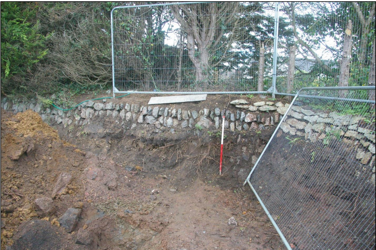
2. WESTERN AND NORTHERN SITE BOUNDARY, VIEWED FROM THE EAST (1M SCALE).
