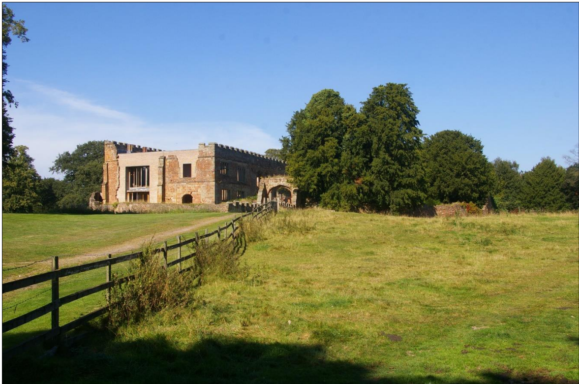
FIGURE 26: ASTLEY CASTLE MOATED SITE; VIEWED FROM THE SOUTH-SOUTH-EAST.
