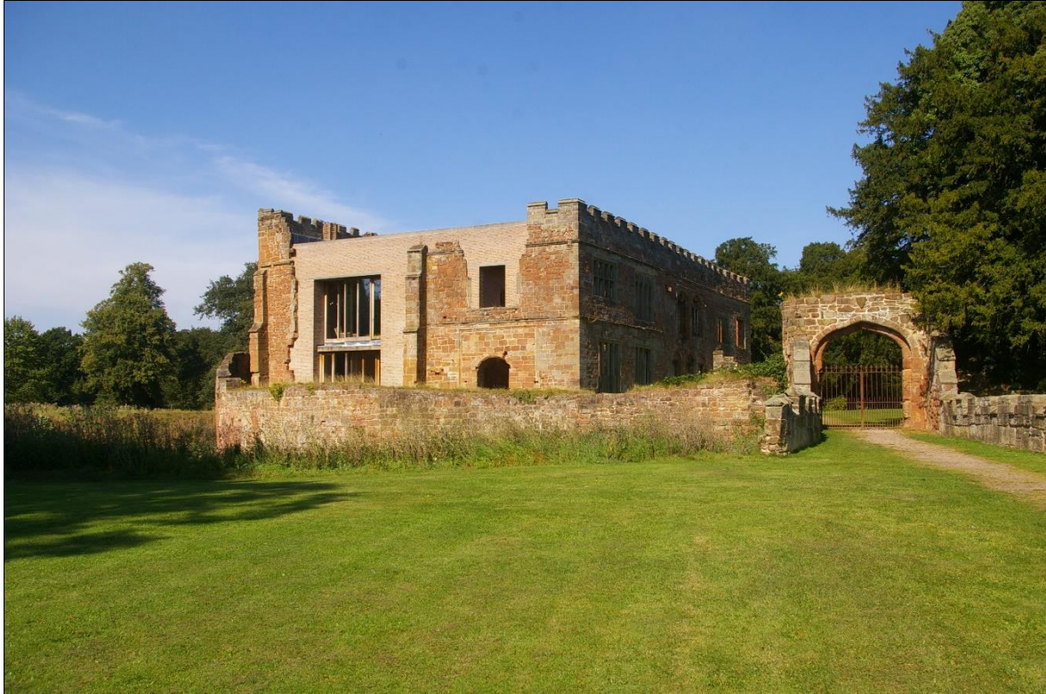
FIGURE 27: ASTLEY CASTLE; VIEWED FROM THE SOUTH-EAST.
