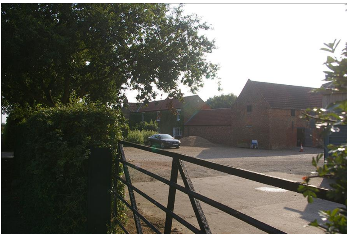
FIGURE 28: WAWNE GRANGE; VIEWED FROM THE NORTH-EAST.
