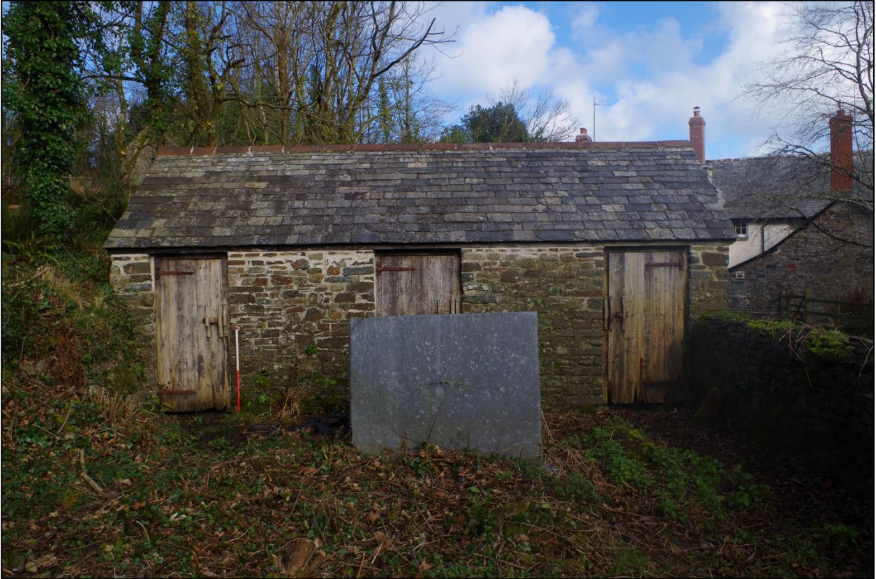
5. THE SOUTH ELEVATION OF THE PIGGERY. TAKEN FROM THE SOUTH WITH 1M SCALES.
