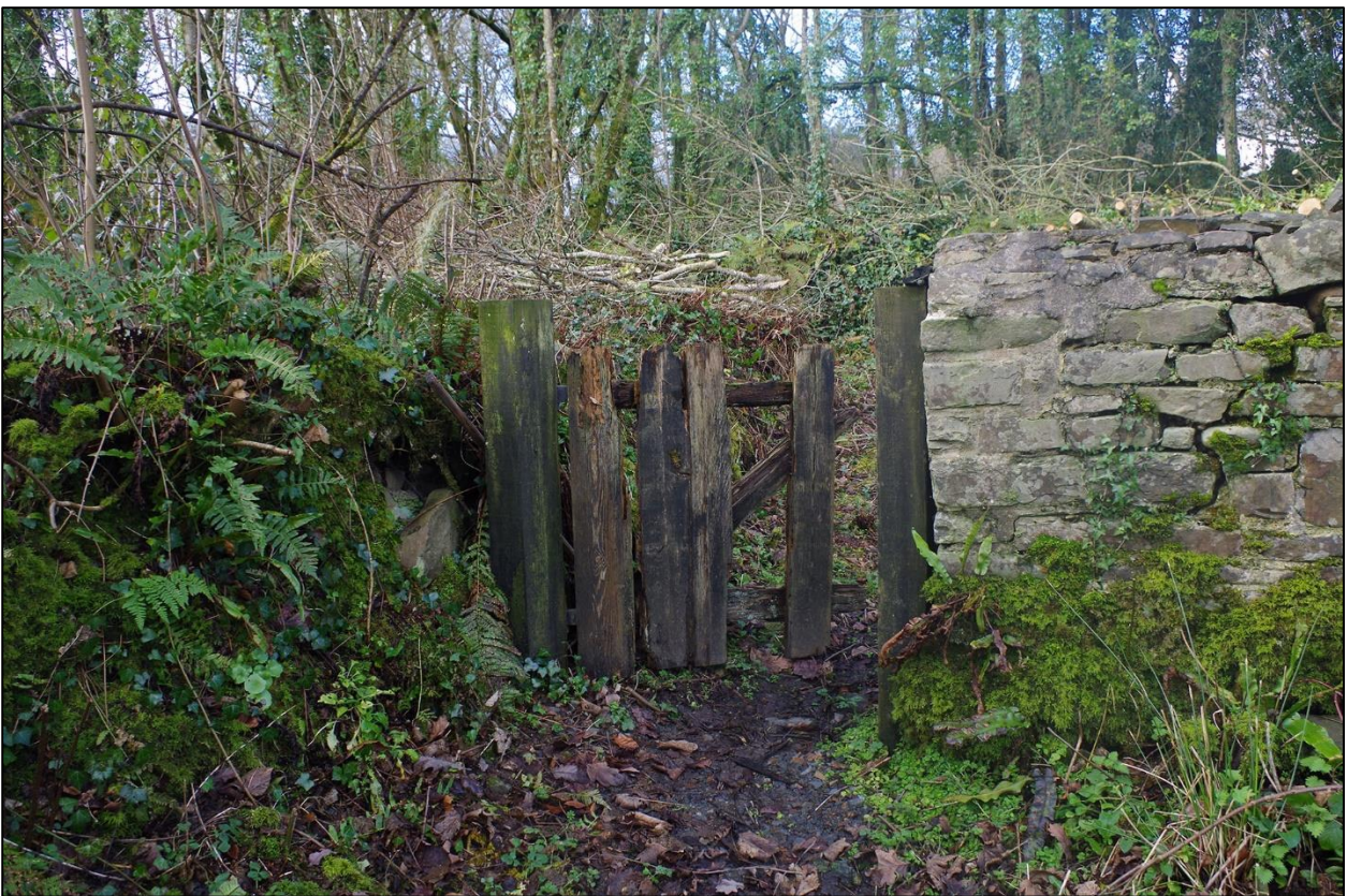
4. THE TIMBER GATE ENTRANCE TO THE YARD. TAKEN FROM THE EAST.
