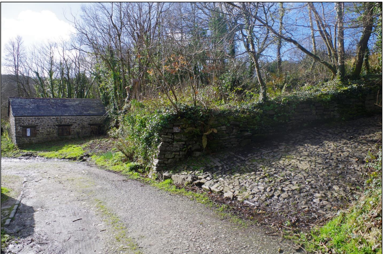
2. ON APPROACH THE PIGGERY FROM THE NORTH, INCLUDING A COBBLED LANE CONNECTING BROWNSHAM COTTAGE TO LOWER BROWNSHAM FARM. TAKEN FROM THE NORTH.
