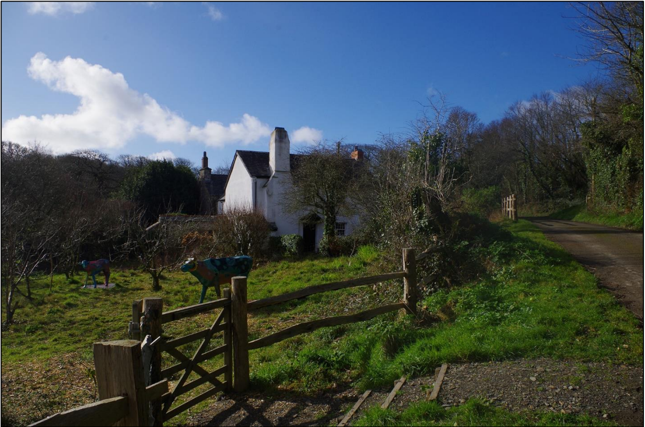
1. BROWNSHAM COTTAGE BY THE NT CAR PARK AT THE TOP OF THE HAMLET. TAKEN FROM THE NORTH-EAST.
