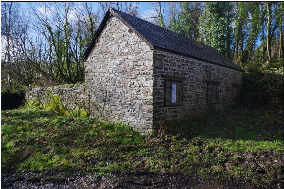
FIGURE 9: THE NORTH AND EAST ELEVATIONS OF THE BUILDING, SHOWING THE LOW-HANGING WINDOWS WITH TIMBER LATCHES AND THE EASTERN BOUNDARY WALL FOR THE YARD. TAKEN FROM THE NORTH-EAST.
