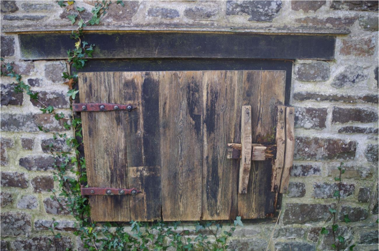
9. THE EXTERNAL FACE OF THE WINDOWS WITH SLIDING TIMBER LATCHES. TAKEN FROM THE NORTH.
