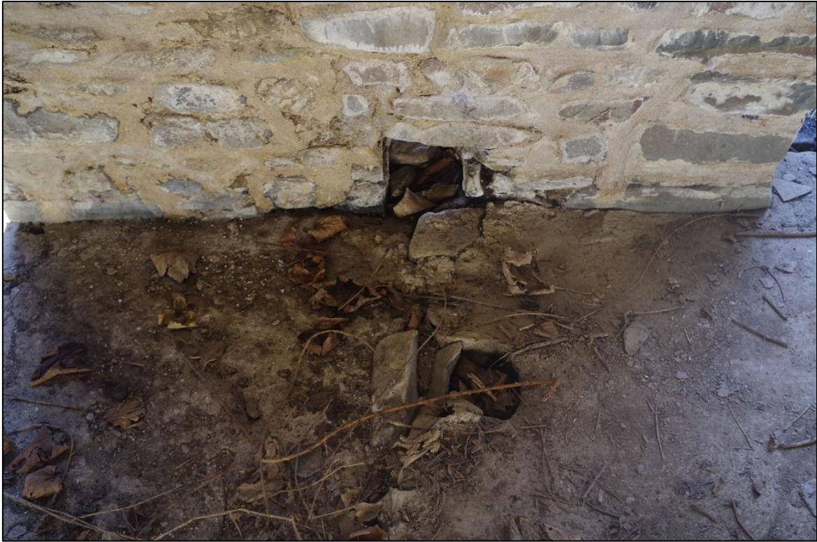
FIGURE 10: REMAINS OF A POSTHOLE WITHIN THE CONCRETED FLOOR IN LINE WITH A STALL SECTION, AND THE GUTTER HOLE IN THE SOUTH ELEVATION.
