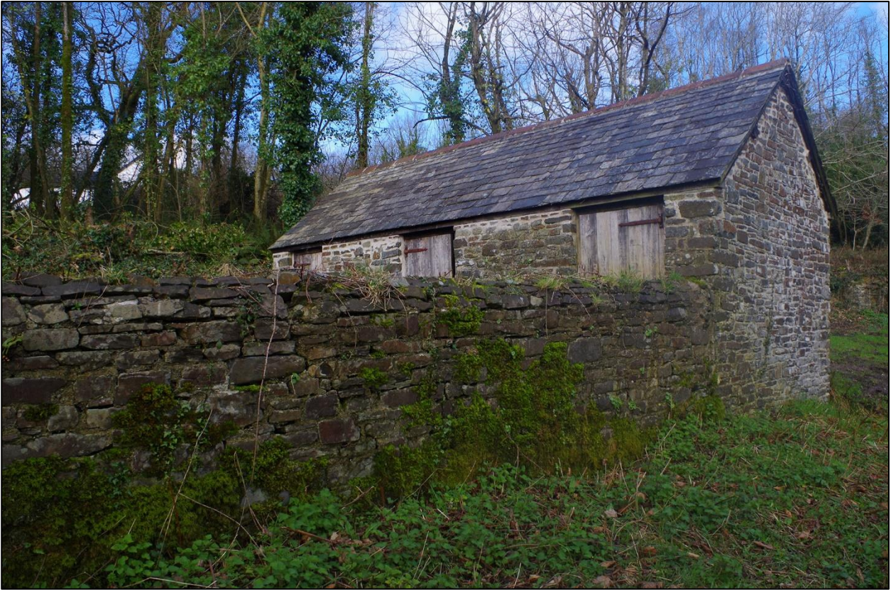
3. THE PIGGERY INCLUDING EAST WALLED ELEVATION. TAKEN FROM THE SOUTH-EAST.
