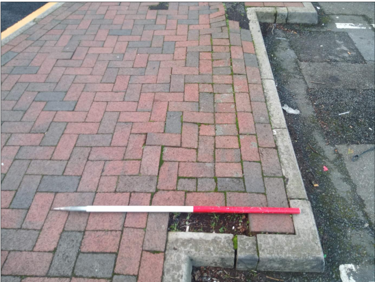
FIGURE 3: SITE OF ORIGINAL LOCATION OF PIT, SHOWING ROOT DISTURBANCE OF PAVING; FROM THE NORTH (1M SCALE).
