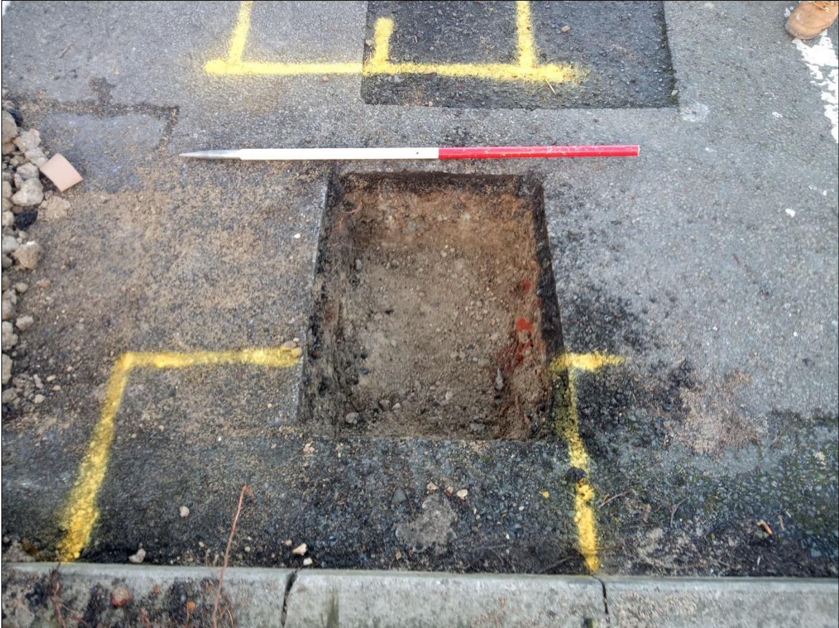
FIGURE 2: EXCAVATED PIT; FROM THE SOUTH-EAST (1M SCALE).
