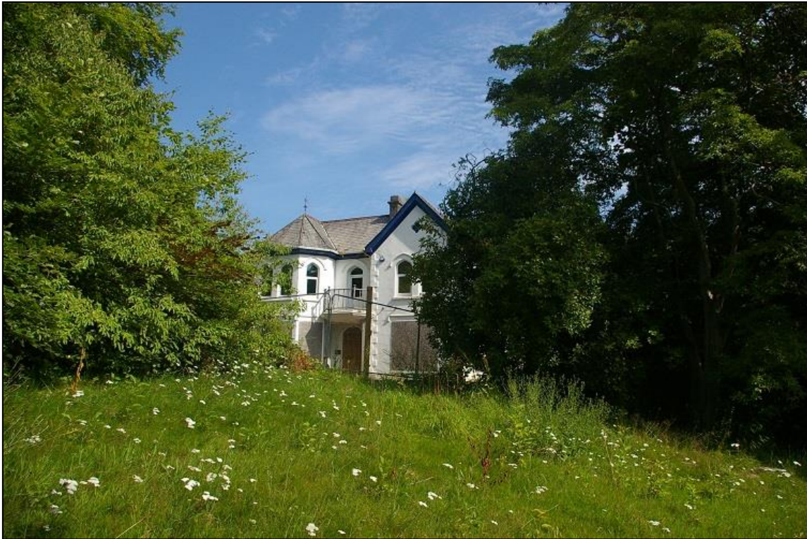
FIGURE 22: VIEW TO THE HOUSE FROM THE SOUTH-EASTERN 'GLADE' IN THE GARDEN.
