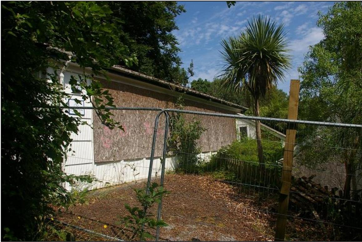
11. ONE OF THE SINGLE STOREY MODERN CLASSROOM BLOCKS; FROM THE SOUTH-EAST.
