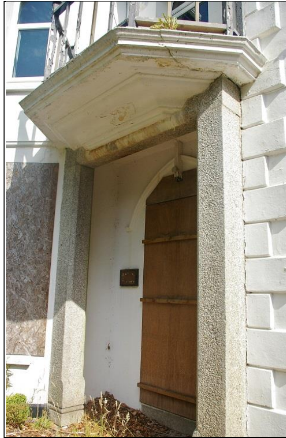
19. THE GRANITE DECORATIVE PORCH; FROM THE SOUTH-EAST.
