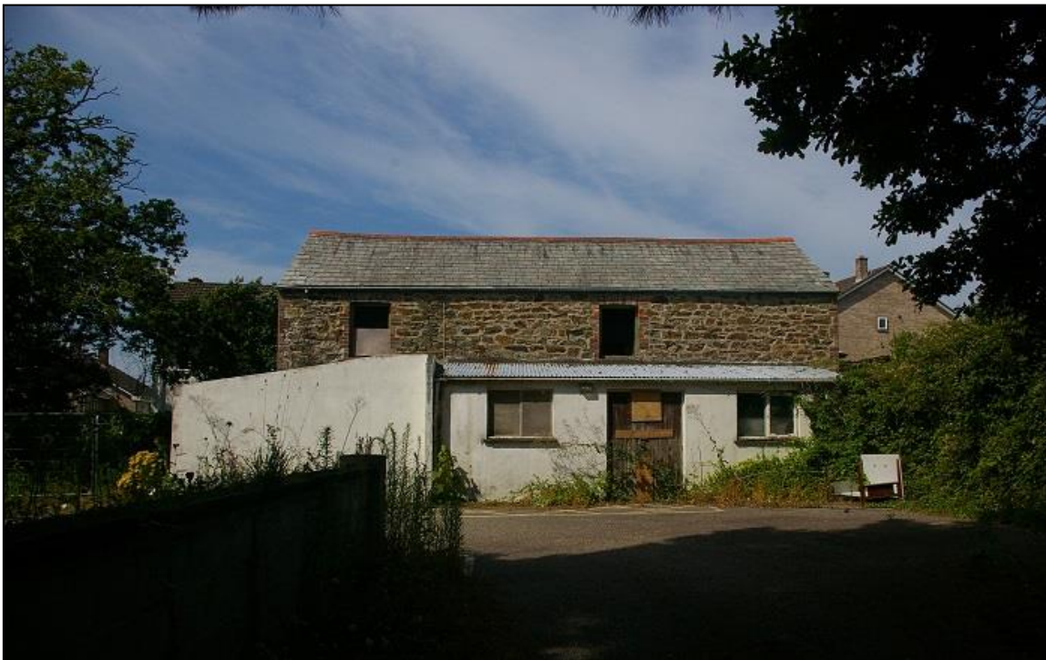
FIGURE 18: THE OUTBUILDING AT THE TOP OF THE SITE; FROM THE EAST.
