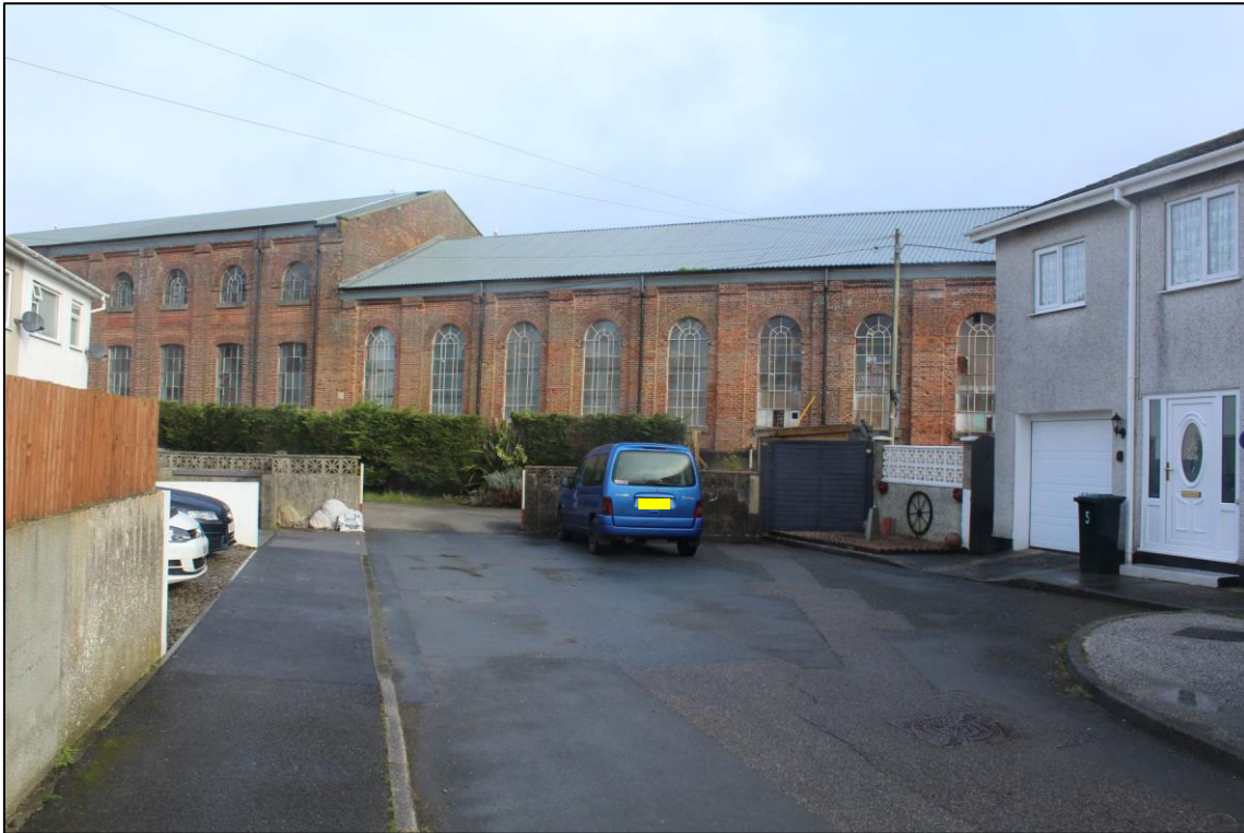
FIGURE 27: THE GII* LISTED ENGINE SHEDS, VIEWED FROM THE SOUTH.
