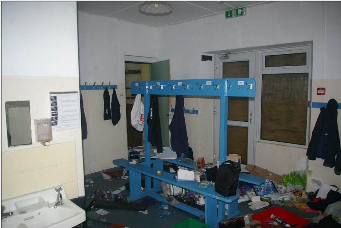
23. ONE OF THE CHANGING ROOMS IN THE NORTH-EAST RANGE; FROM THE SOUTH-WEST.
