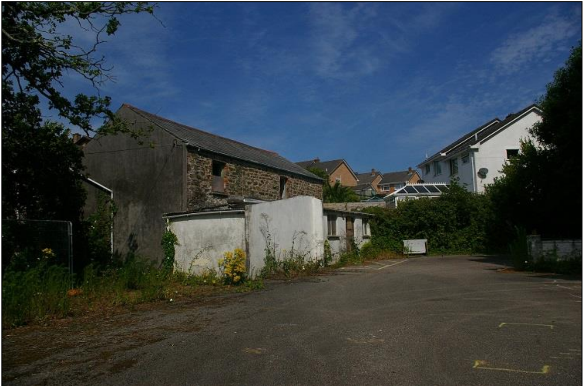
10. THE EDWARDIAN OUTBUILDING TO THE SOUTH-WEST OF THE SITE, SHOWING ITS FRAGMENTED SETTING, ENCLOSED BY MODERN HOUSING; FROM THE SOUTH.
