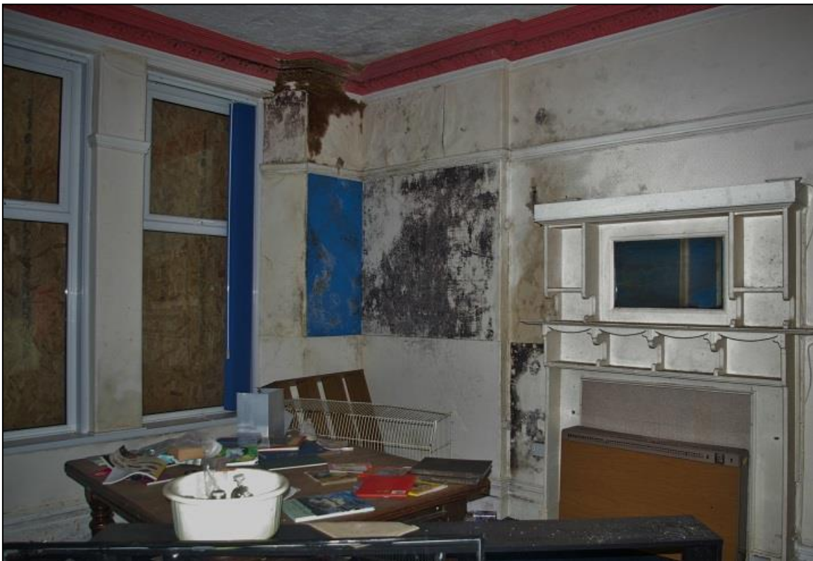
FIGURE 15: THE FRONT EAST RECEPTION ROOM, WITH FINE FIREPLACE AND PLASTER CORNICE, PICTURE RAIL AND SKIRTING BOARDS; FROM THE NORTH-EAST.
