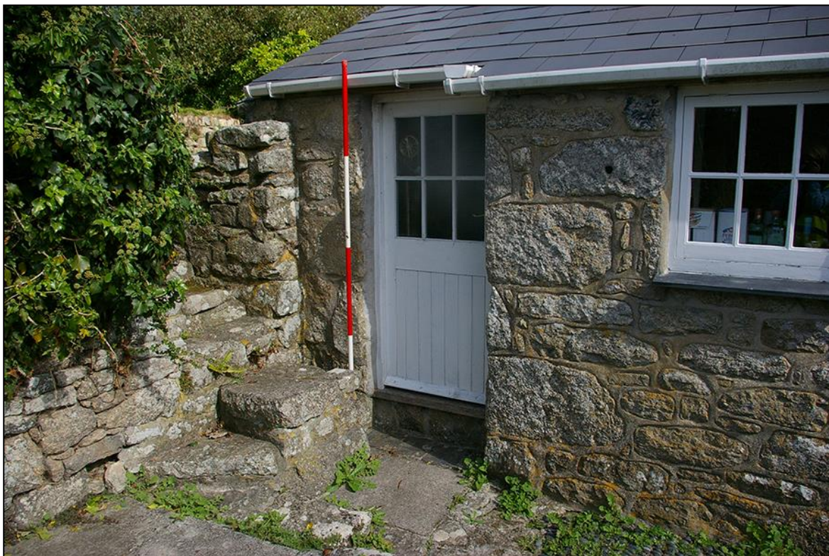
8. THE END OF THE LEAN-TO, BUILDING 2; FROM THE SOUTH-WEST.
