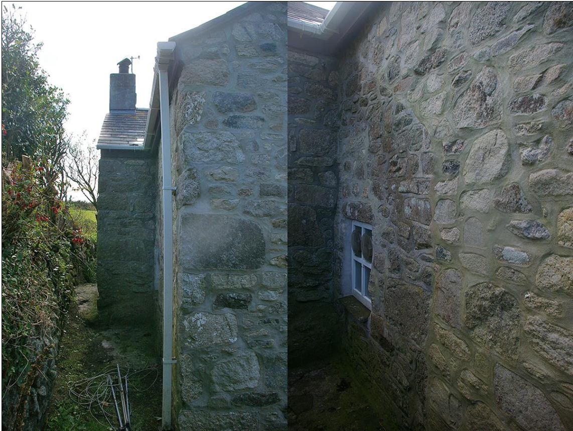
14. LEFT: THE CORNER OF THE BUILDING, SHOWING INTEGRAL CHIMNEY STACK AND RETAINING WALLS; FROM THE NORTH-NORTH-WEST. 15. RIGHT: THE WALL, WITH CLEAR BUILD LINE SHOWING AN EXTENDED LEAN-TO IN THIS POSITION; FROM THE NORTH.
