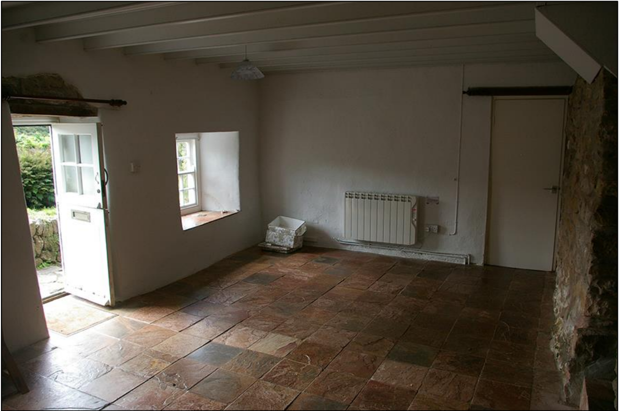
16. ROOM 1, SHOWING THE SOUTH FRONT AND WEST WALL; FROM THE EAST-NORTH-EAST.
