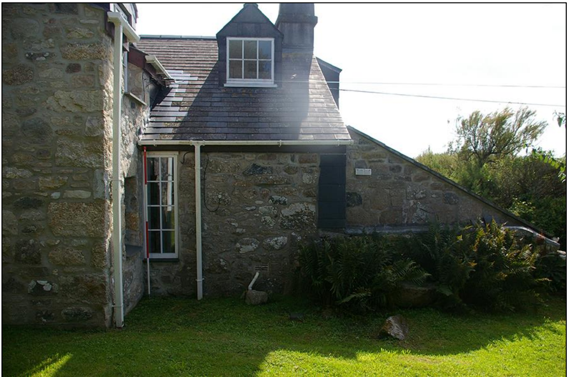
12. THE REAR OF THE HOUSE, WITH 2M SCALE; FROM THE NORTH-NORTH-WEST.
