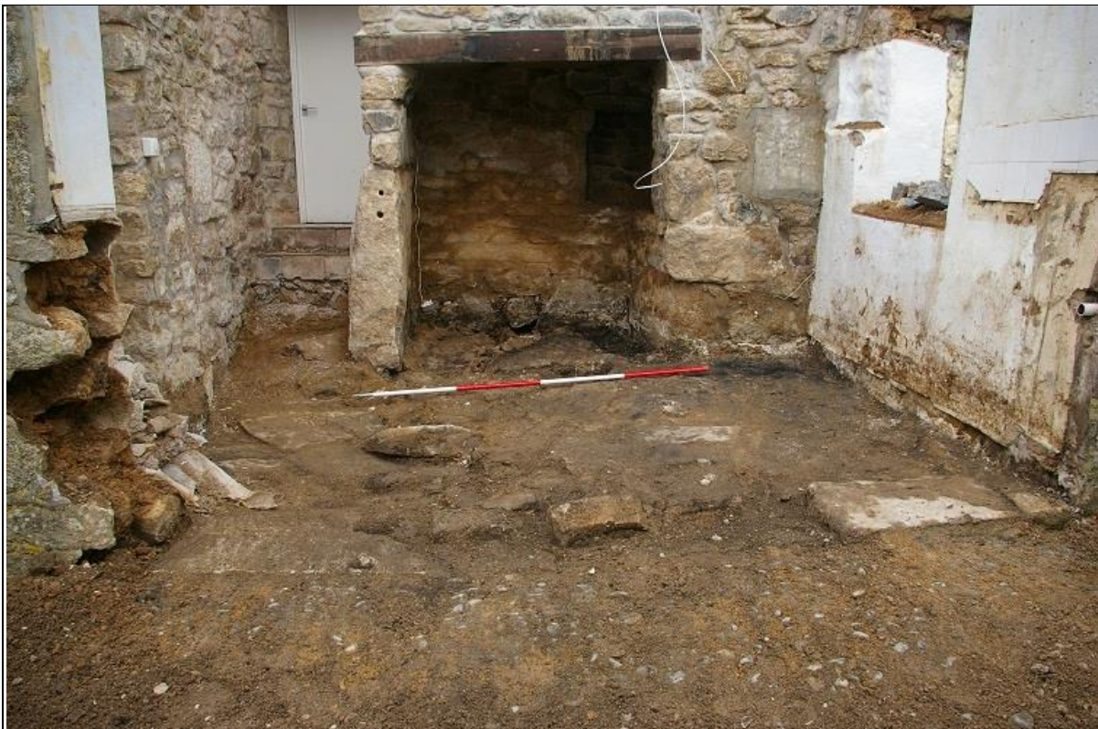
21. THE CLEARED HISTORIC REMAINS UNDER THE LEAN-TO — SHOWING TWO PHASES OF FLOORING (2M SCALE); FROM THE WEST.
