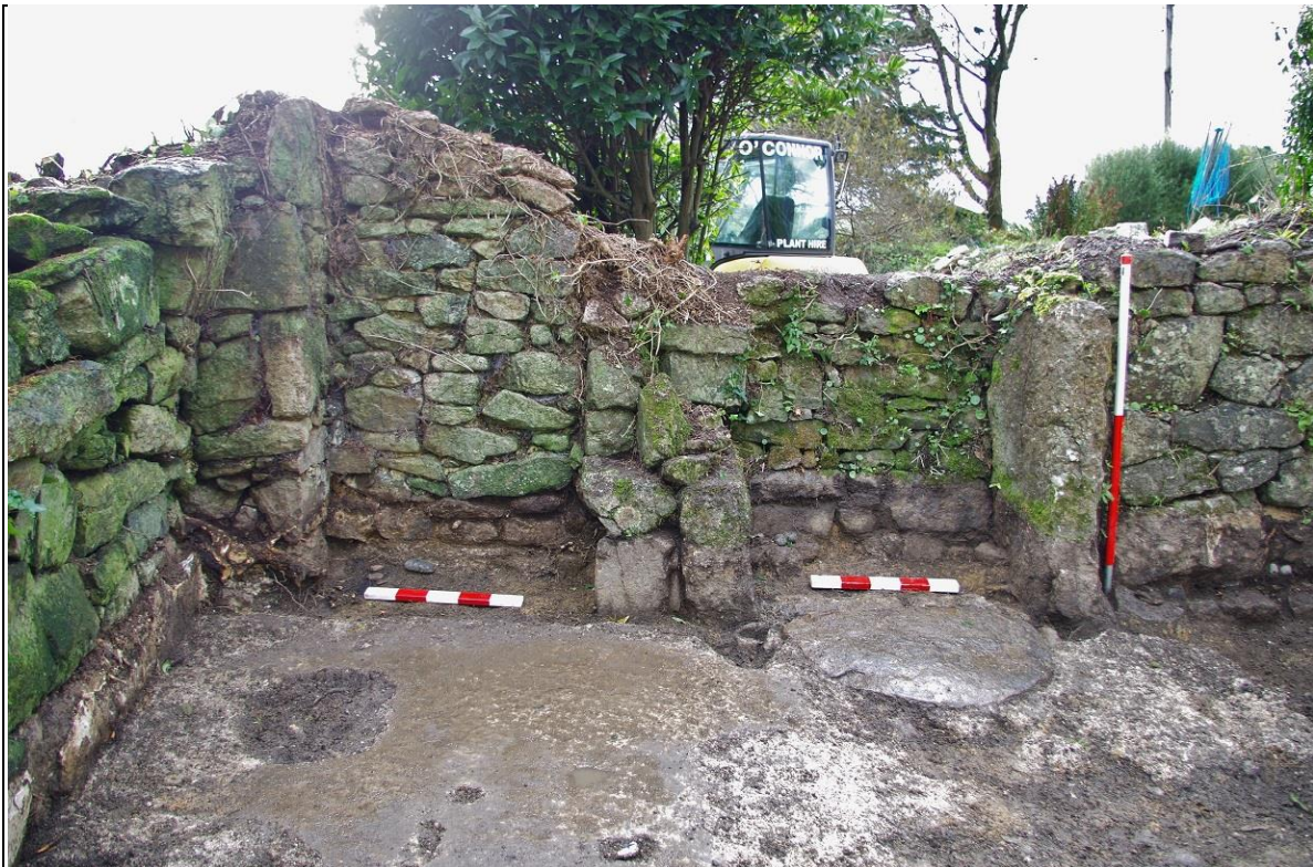
8. THE WEST WALL {041} OF THE RUIN, SHOWING THE BLOCKED DOOR, 'SOUTH' OF THE FIREPLACE AND THE FIREPLACE; FROM THE EAST (1M AND 0.5M SCALES).
