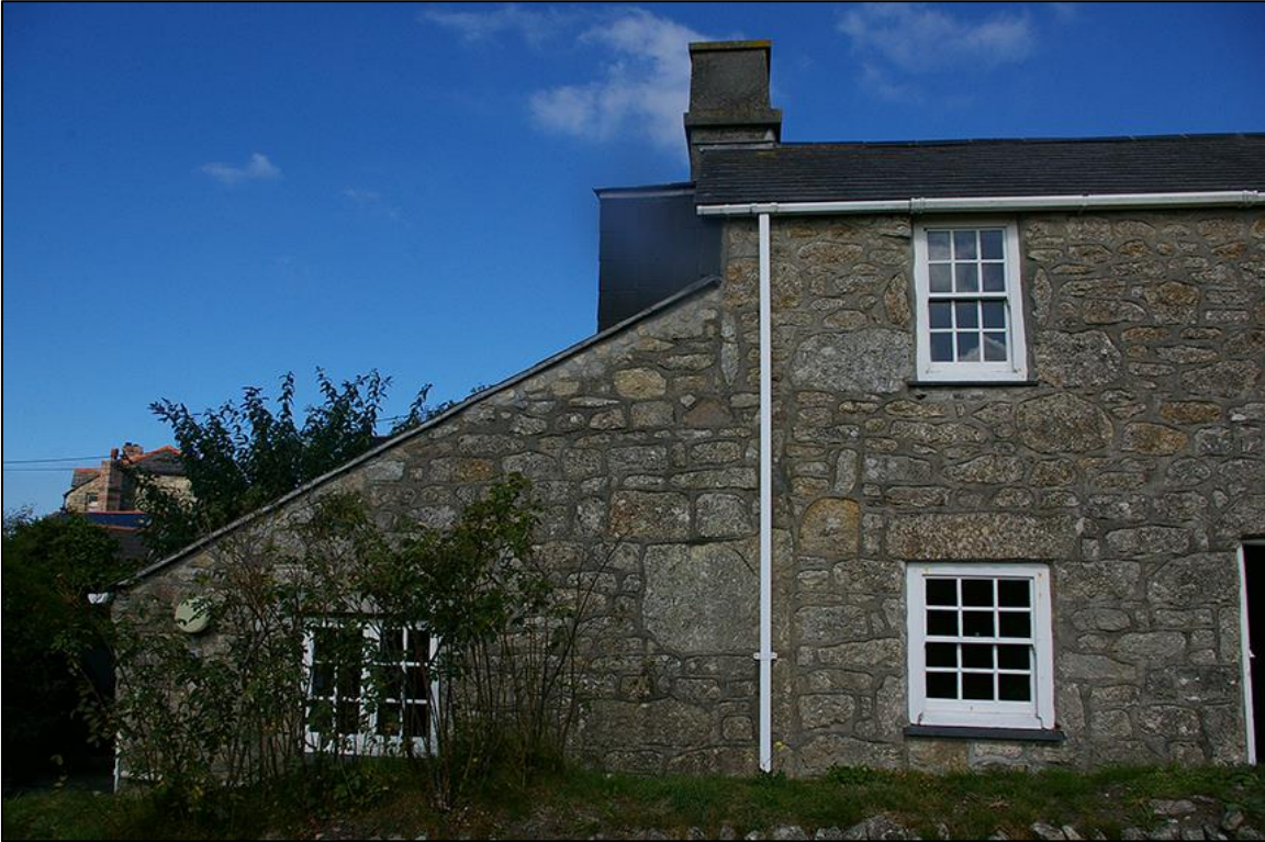
5. BUILDING 1 AND THE LEAN-TO BUILDING 2, WHICH ABUTS IT; FROM THE SOUTH-SOUTH-EAST.
