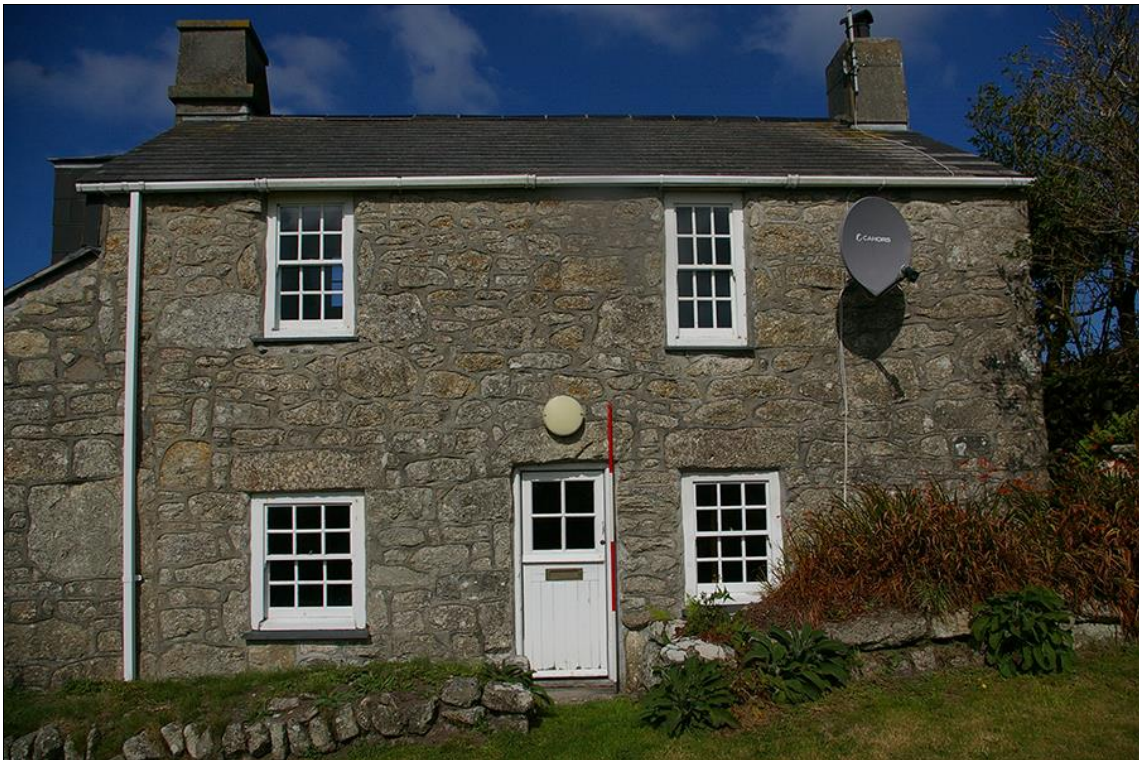
6. THE FRONT OF THE COTTAGE, WITH 2M SCALE; FROM THE SOUTH-SOUTH-EAST.
