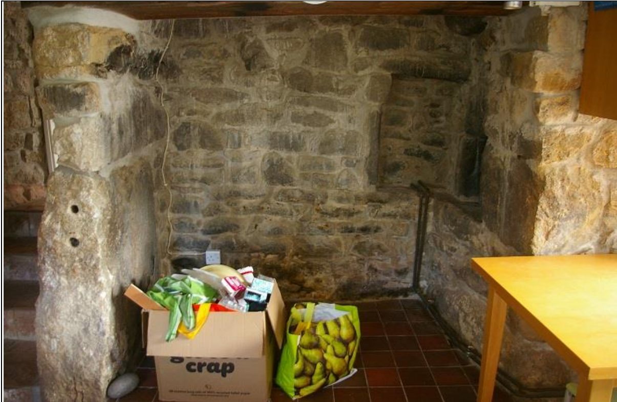
23. THE FIREPLACE IN ROOM, BUILDING 2; FROM THE WEST-SOUTH-WEST.
