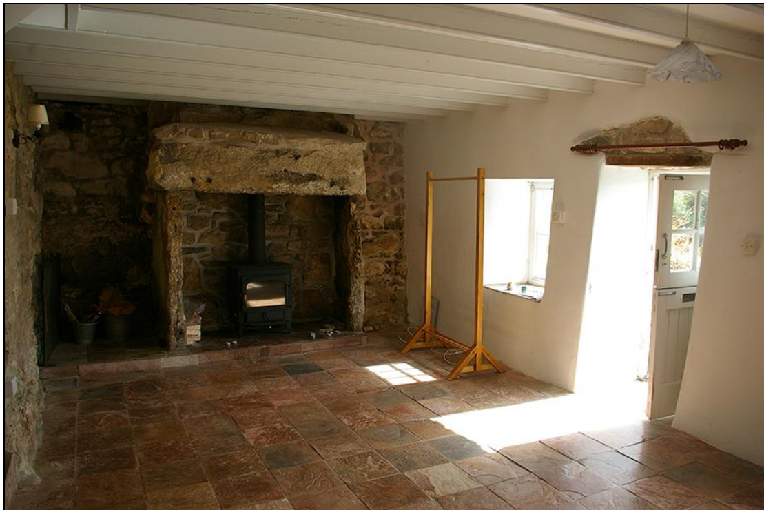
FIGURE 7: THE MAIN GROUND FLOOR SPACE IN BUILDING 1; FROM THE SOUTH-SOUTH-WEST.
