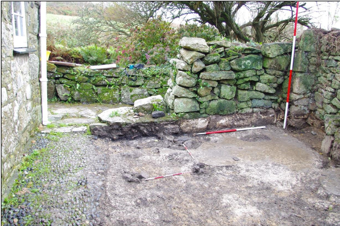
5. THE REBUILT FRONT WALL OF THE RUIN; FROM THE NORTH, WITH OLDER SINGLE COURSE BELOW {048} (2M, 1M AND 0.5M SCALES).
