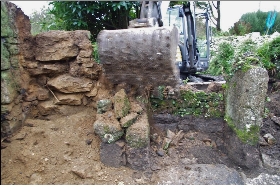
18. THE FIREPLACE {042} BEING DEMOLISHED, WORKING SHOT; FROM THE EAST.
