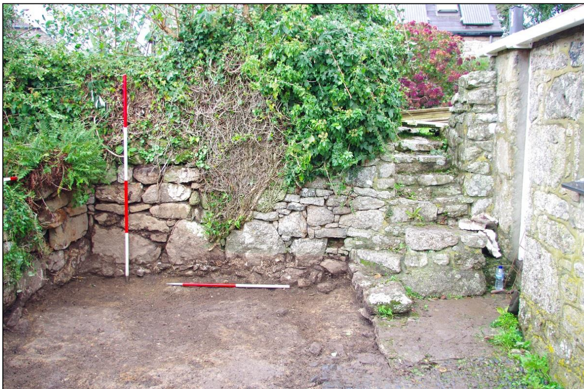
6. THE NORTH WALL OF THE BUILDING – ALTERED WITH STEPS CUT IN – POSSIBLY SET INTO A DOORWAY, WITH RAISED GARDEN LEVEL BEHIND; FROM THE SOUTH (1M AND 2M SCALES).
