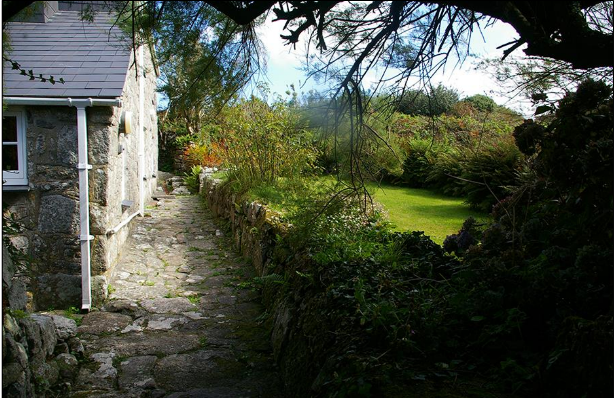
3. THE PATH WHICH RUNS ALONG THE FRONT OF THE COTTAGE, WITH WORN STONE SLABS; FROM THE WEST.
