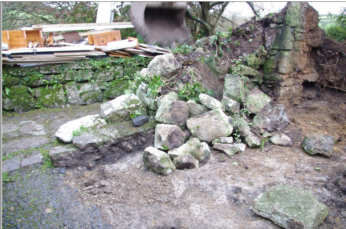
19. THE FRONT WALL {084} BEING DEMOLISHED – SHOWING TOPSOIL CORE; FROM THE NORTH-EAST.
