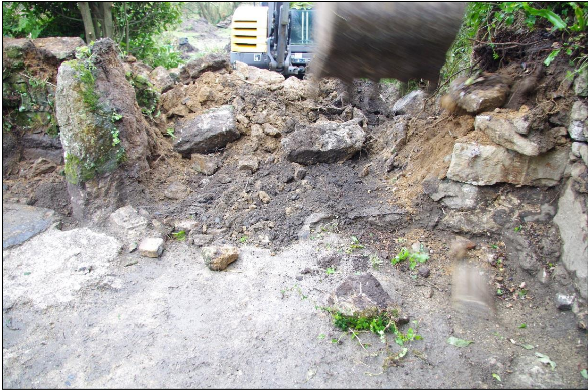
17. DEMOLISHING THE WEST WALL {041}, WORKING SHOT; FROM THE EAST-NORTH-EAST.
