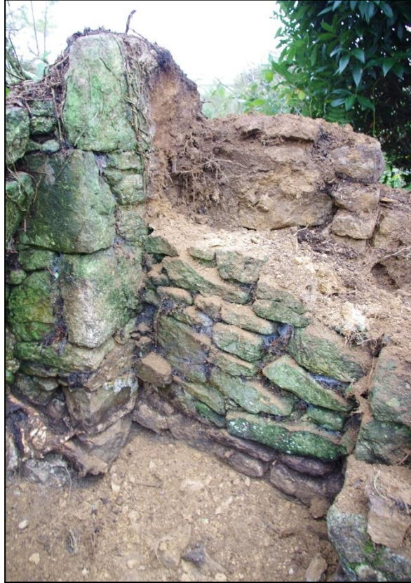
11. THE BLOCKED DOORWAY {022} IN THE WEST WALL, ALTERED BY THE ADDITION OF THE FIREPLACE; FROM THE NORTH-EAST.
