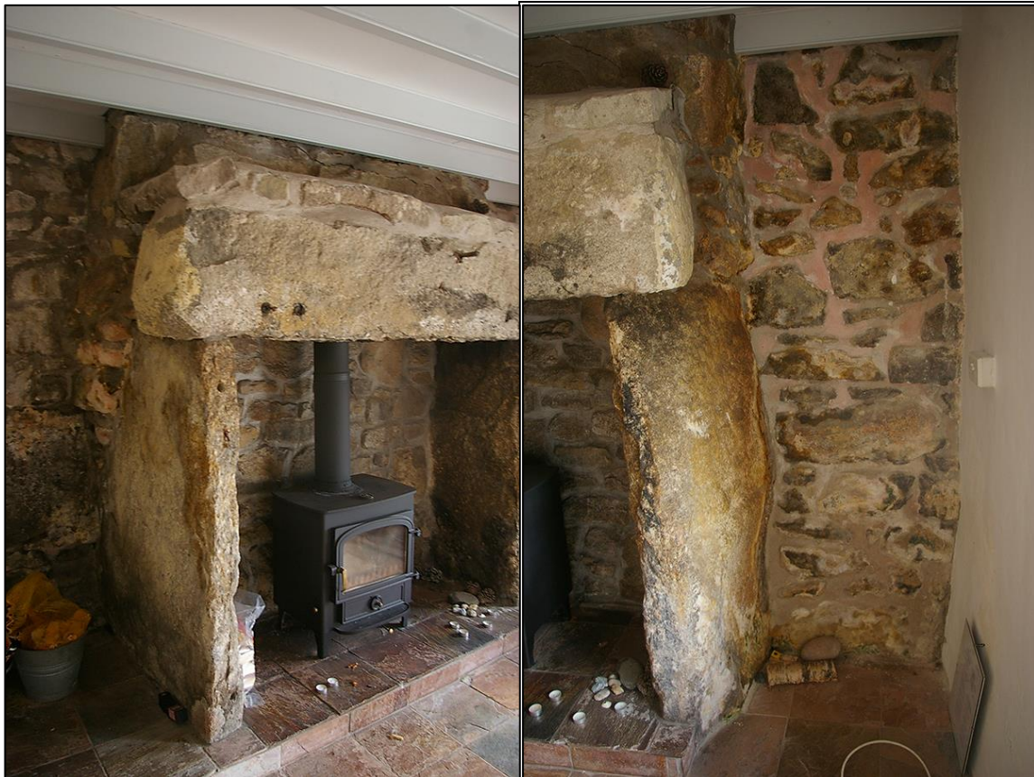
19. THE NORTH/SOUTH SIDES OF THE LARGE ORTHOSTAT FIREPLACE IN ROOM 1.
