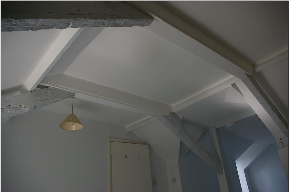
FIGURE 9: THE RUSTIC ROOF TRUSSES IN BUILDING 1, THEIR SPIKED LOW COLLARS REMOVED WHEN THE CEILINGS WERE RAISED; FROM THE EAST-NORTH-EAST.
