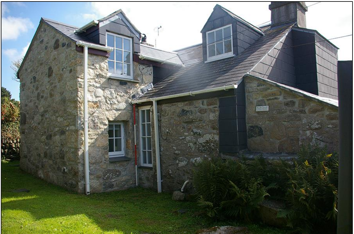
FIGURE 6: BUILDING 1, SHOWING THE RAISED EXTENSION TO A HISTORIC LEAN-TO TO THE REAR OF THE COTTAGE, WITH 2M SCALE; FROM THE NORTH-WEST.
