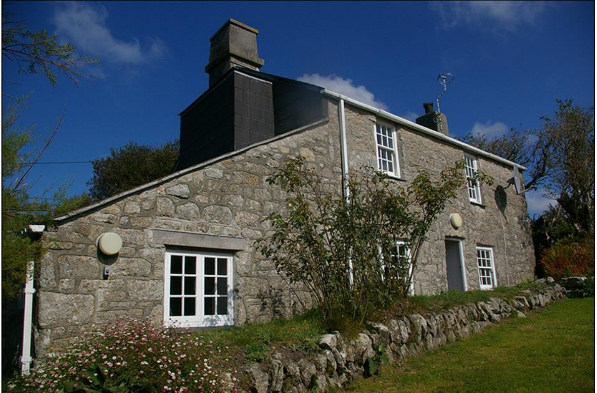
FIGURE 8: BUILDING 2, THE LEAN-TO BUILT UP AGAINST BUILDING 1, THE COTTAGE; FROM THE SOUTH-EAST.
