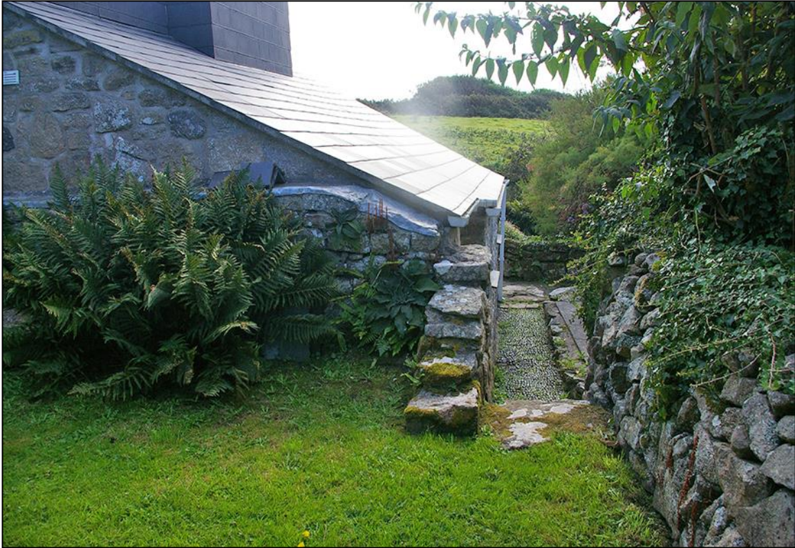
11. THE LEAN-TO, BUILDING 2; FROM THE NORTH-WEST.
