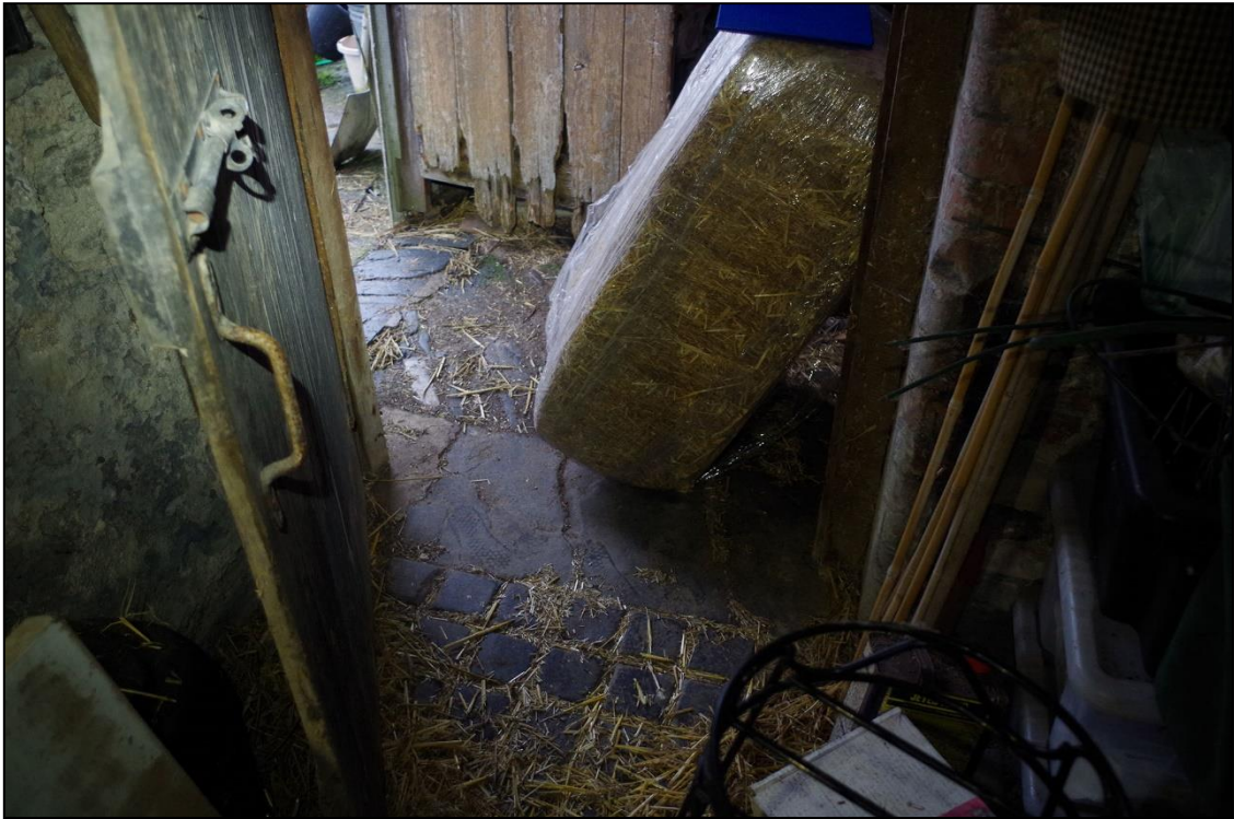
5. THE SLATE HERRINGBONE-PATTERNED FLOOR OF B1A MEETS THE QUARRY TILED FLOORING OF B1B.
