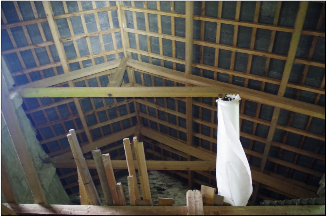
9. 20 TH CENTURY ROOF STRUCTURE IN B1D.
