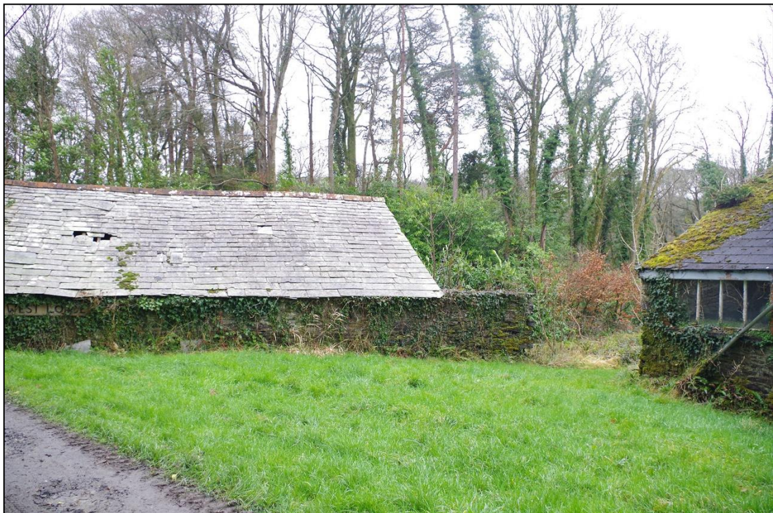
12. RELATIONSHIP BETWEEN B1 & B2 FROM THE NORTH ELEVATION, FORMER OUTBUILDING SAT BETWEEN THE TWO. VIEWED FROM THE WEST.
