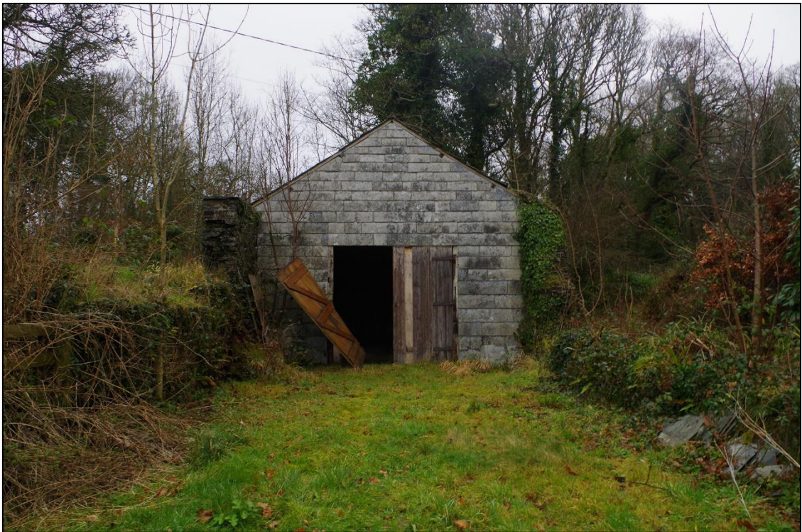
10. SOUTH ELEVATION OF B2, AMONGST RUINOUS B2A. VIEWED FROM THE SOUTH.
