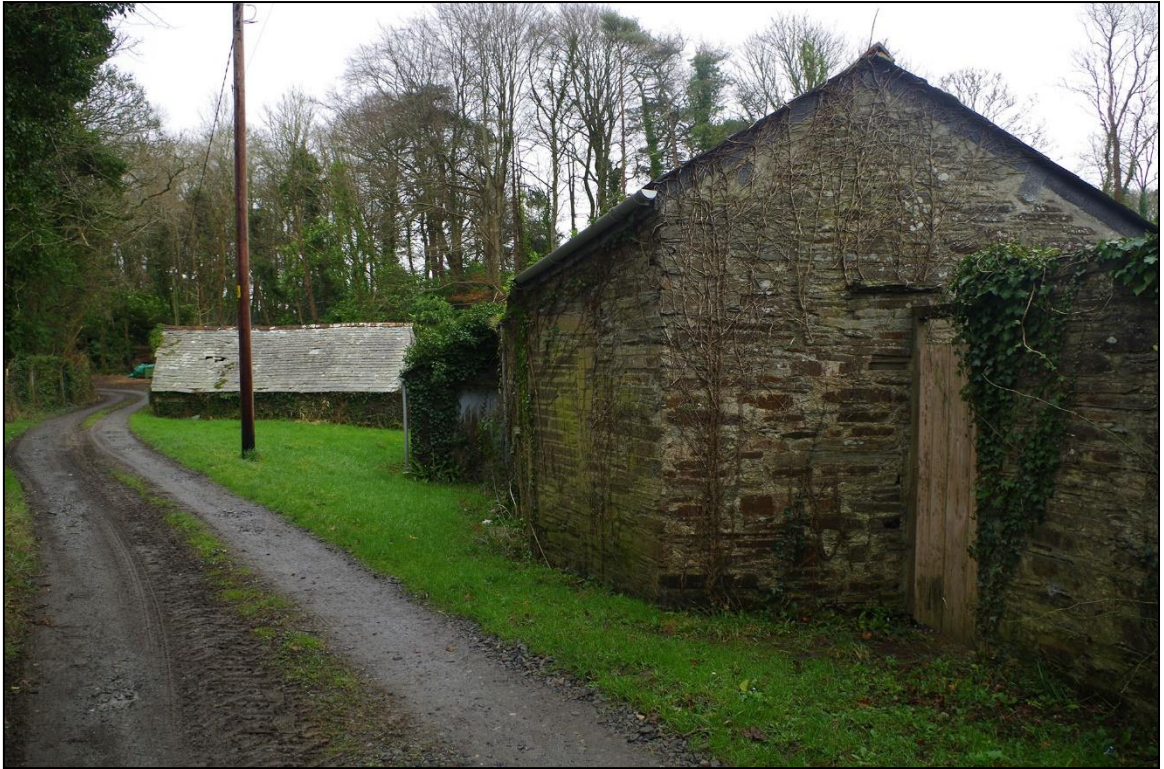
1. THE BARNs FROM THE TRACK, VIEWED FROM THE WEST APPROACH. QUARRY SITS OPPOSITE, GATED OFF.
