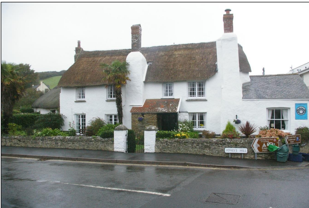
FIGURE 10: BRIDGE FARMHOUSE (GII), VIEWED FROM THE SOUTH-WEST.
