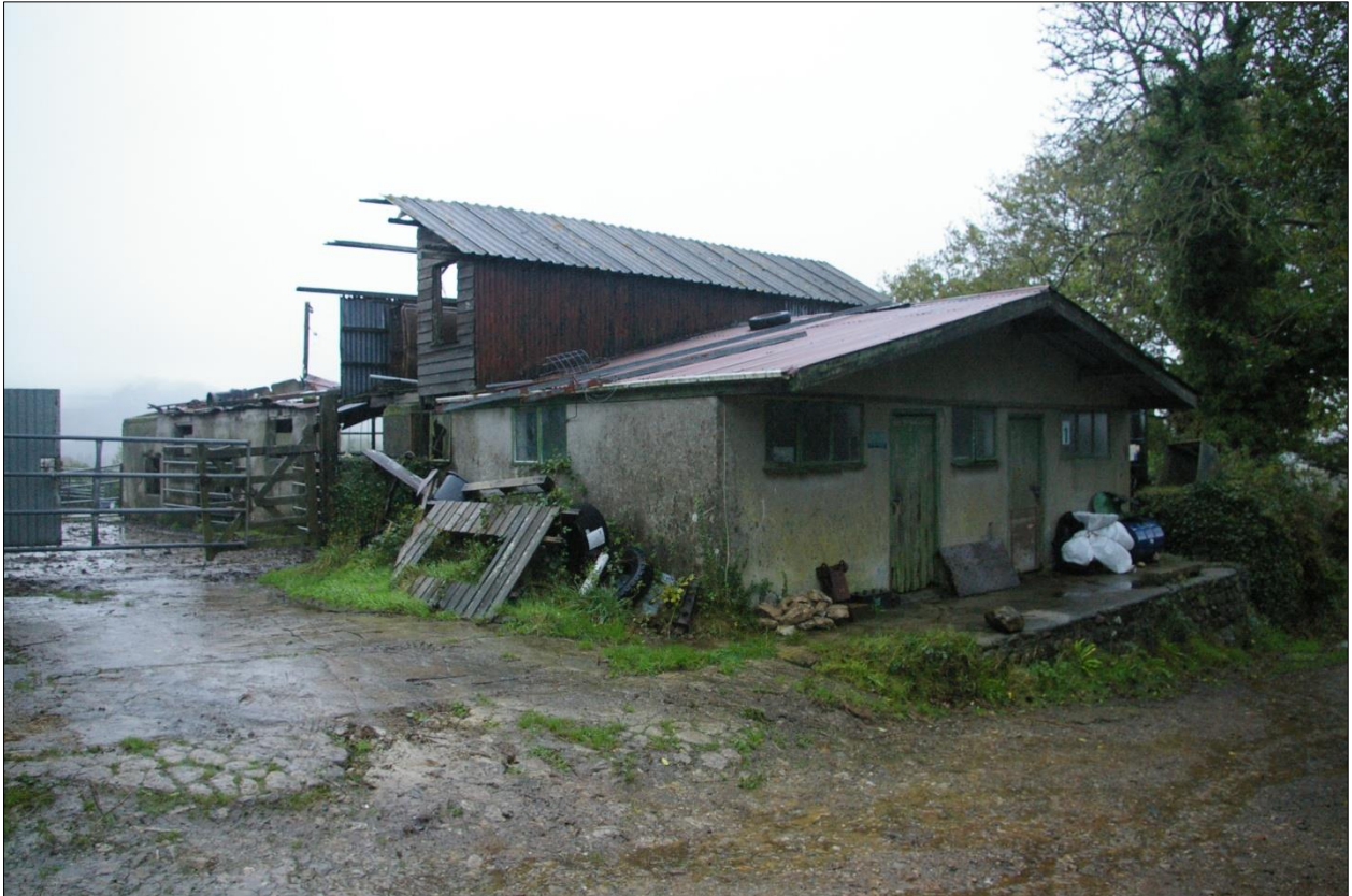
1950/60s farm buildings west of Higher Trehiddle Farm; viewed from the south-west, looking north-east.
