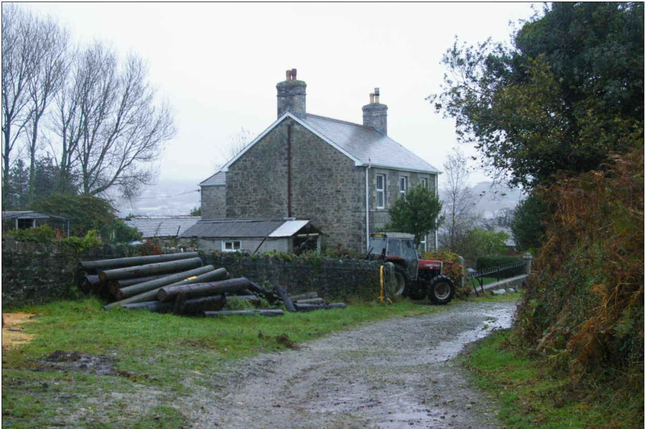
Higher Trehiddle Farmhouse; viewed from the west, looking east.
