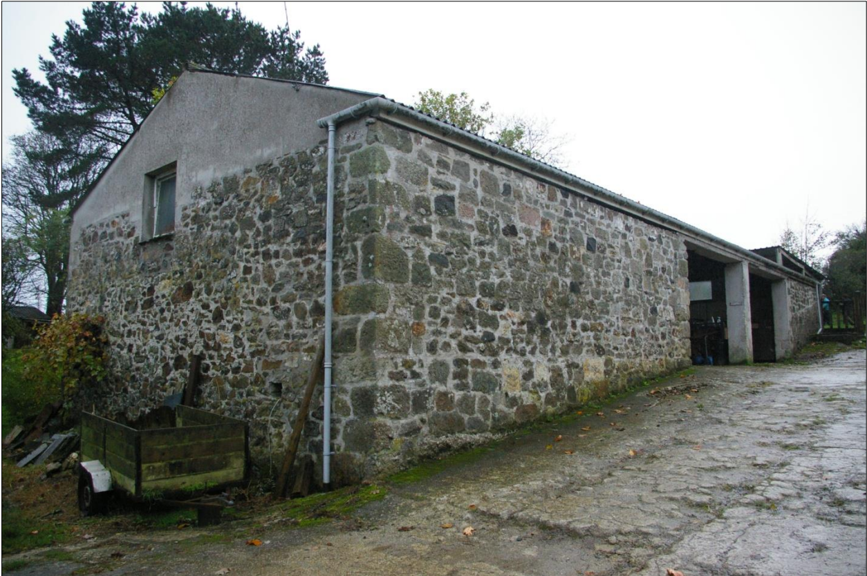
Trehiddle Farm: north elevation of the cartshed(?), viewed from the north-east, looking south-west.
