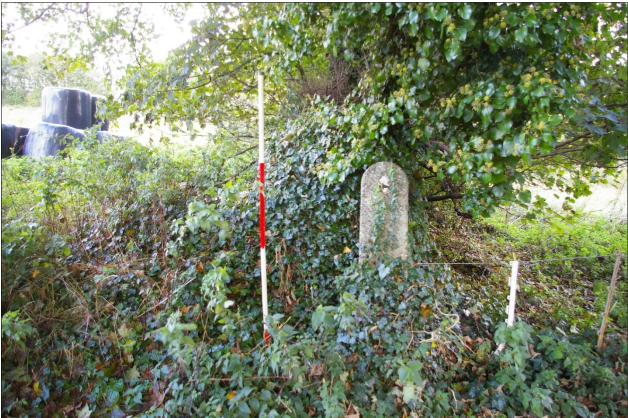
As above, detail of the granite gatepost (scale 2m).
