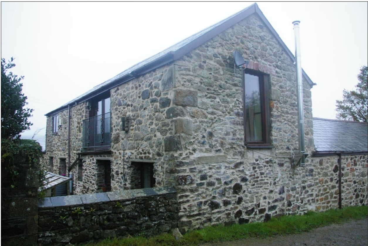
The converted pigsties west of Trehiddle Farm; viewed from the south.
