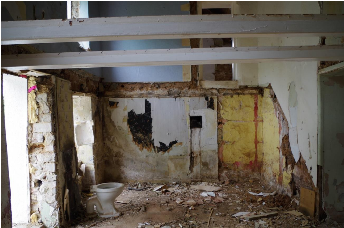
FIGURE 11: THE WEST END OF R3 SHOWING BLOCKED OPENINGS TO THE NORTH THAT SUGGEST A CHANGE IN STAIR PROJECTION. TAKEN FROM THE EAST.
