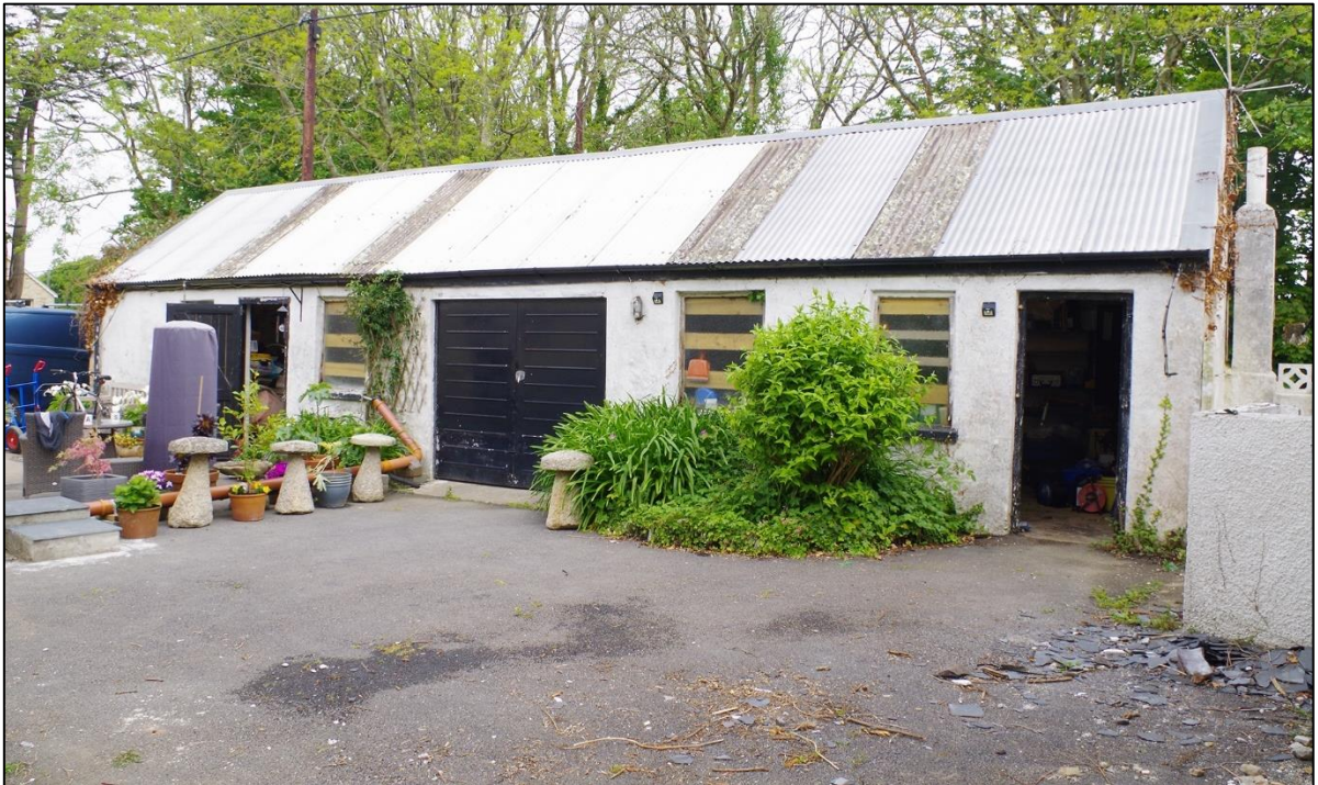
FIGURE 12: THE OUTBUILDING ON THE NORTH BOUNDARY; TAKEN FROM THE SOUTH-EAST.
