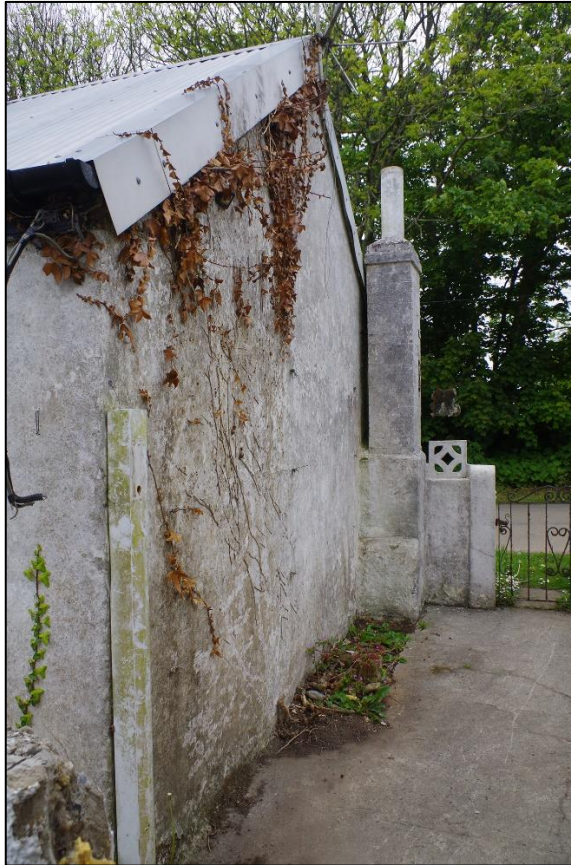
FIGURE 13: BRICK STACK (NOW REMOVED) ON OUTBUILDING TO THE NORTH-EAST CORNER.
