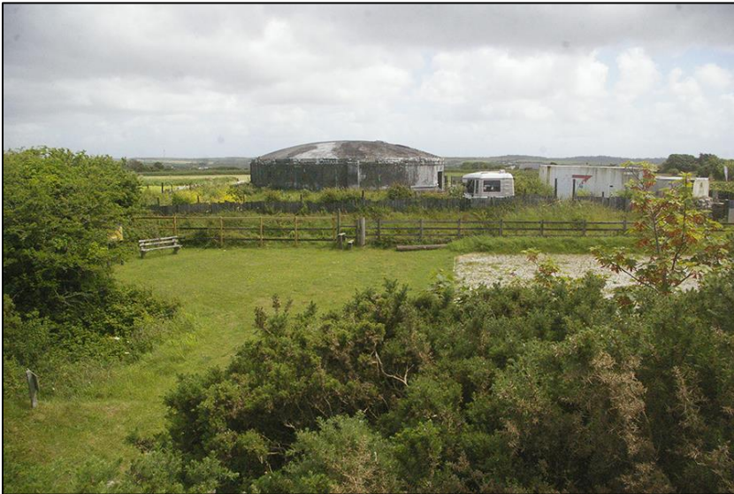
8. VIEW BEYOND THE SOUTH-EAST ENTRANCE TO ROUND; VIEWED FROM THE NORTH-WEST (NO SCALE).
