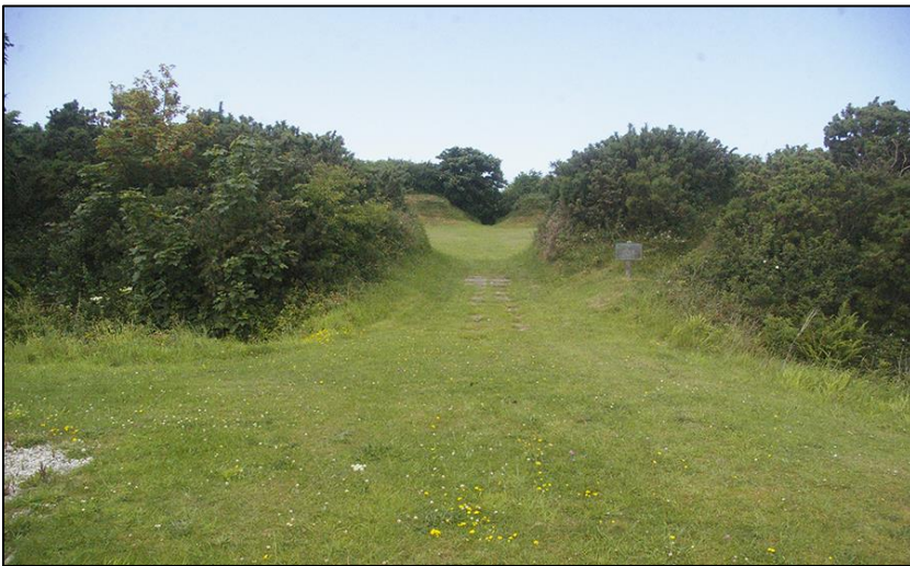
2. SOUTH-EAST ACCESS THROUGH THE BANK TO ST PIRAN'S ROUND; VIEWED FROM THE SOUTH-EAST (NO SCALE).
