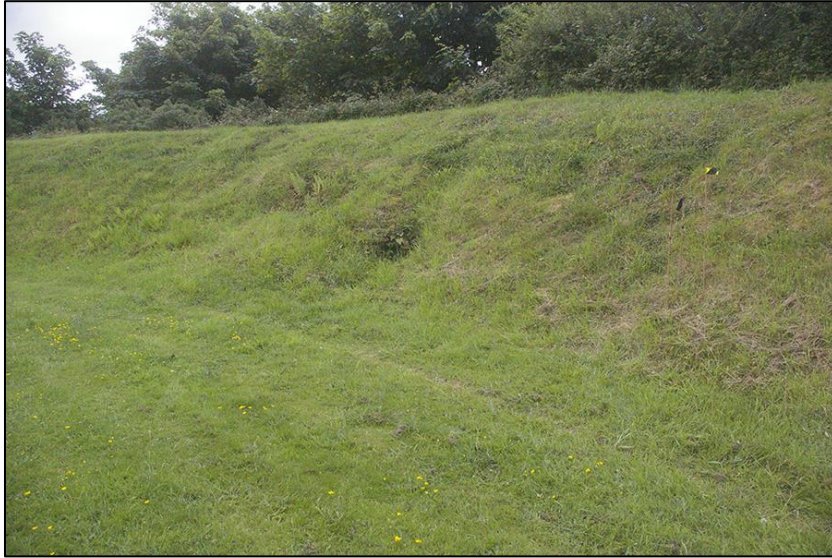
16. BANK EROSION IN THE SOUTH-WEST SEGMENT OF THE ROUND; VIEWED FROM THE NORTH-EAST (NO SCALE).
