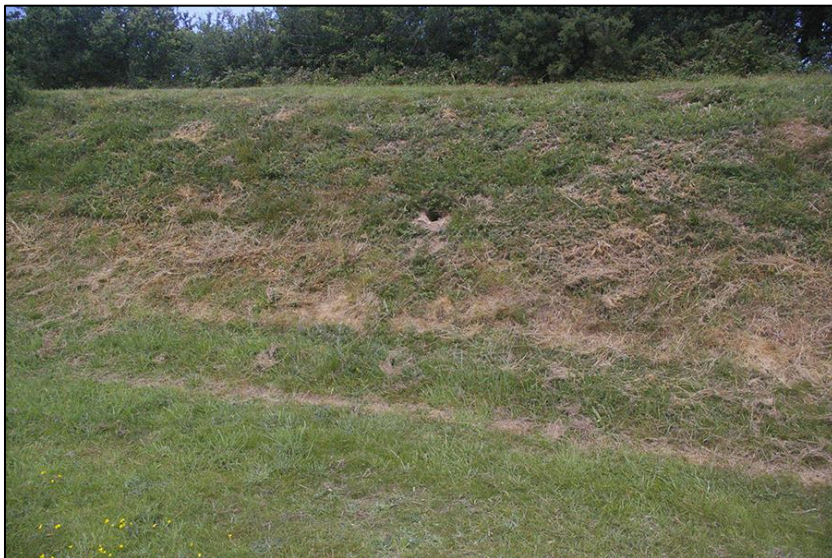
12. RABBIT BURROWS IN THE NORTH SECTION OF THE BANK; VIEWED FROM THE SOUTH-SOUTH-EAST (NO SCALE).
