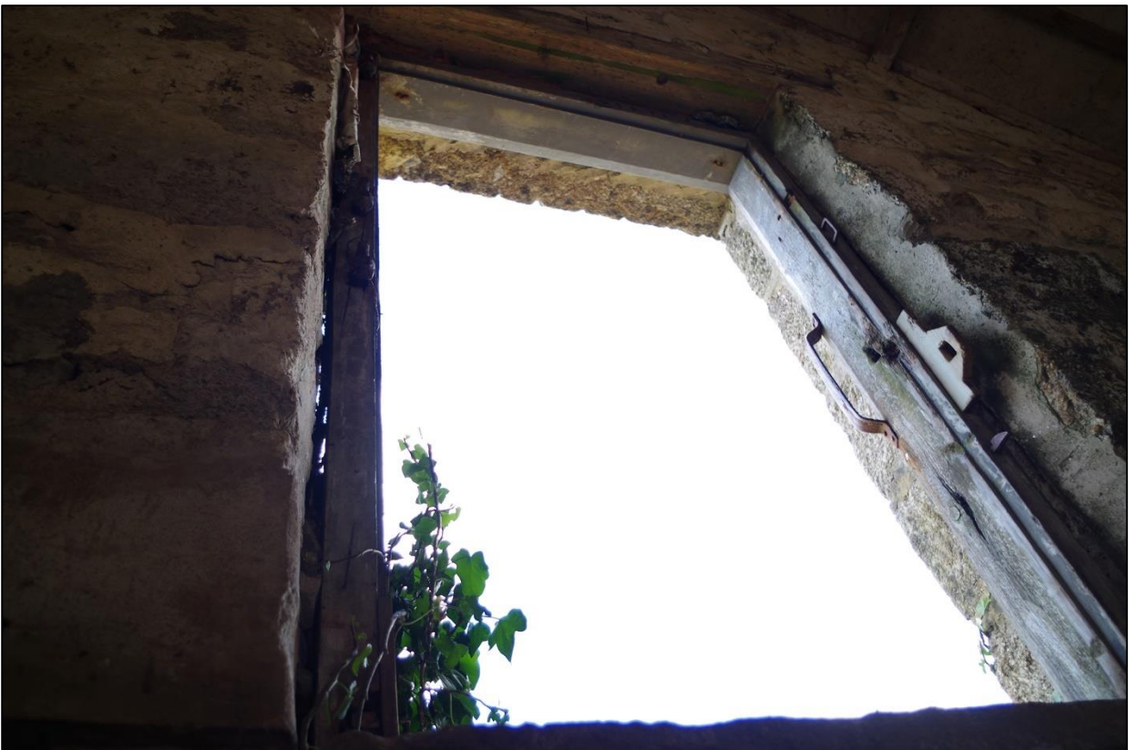
35. B1C, D12 INNER FACE AS SEEN FROM GF.
