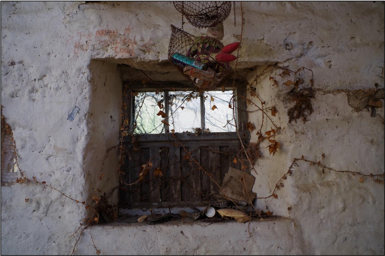
71. W16 INTERNAL FACE; VIEWED FROM THE SOUTH.
