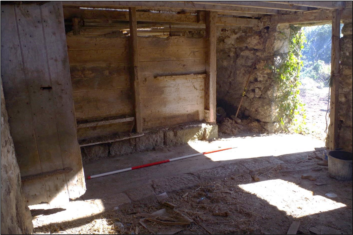
38. B1C, FLOOR WITH POSS. EARLIER PARTITION RUNNING BETWEEN D5 & D6; VIEWED FROM THE NORTH-WEST (SCALE 2M).
