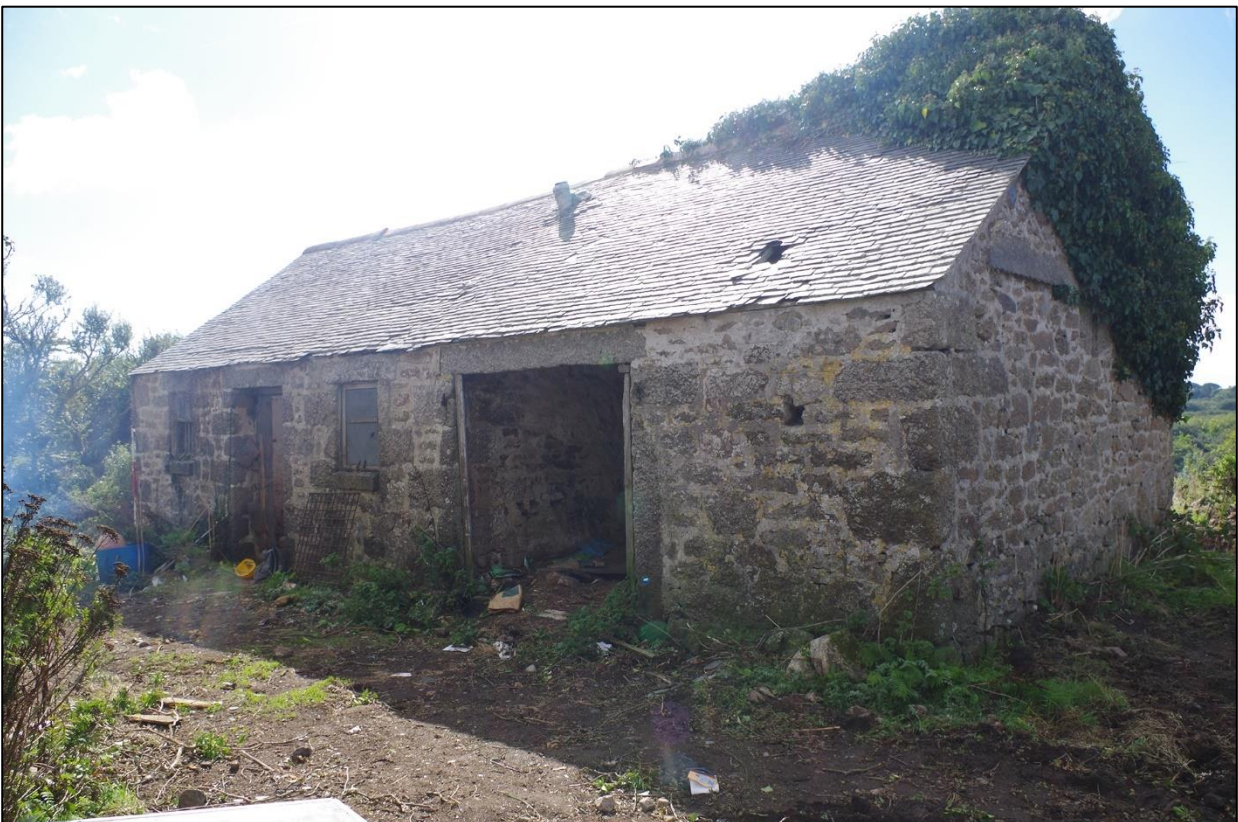
66. B2, NORTH ELEVATION; VIEWED FROM THE NORTH-WEST (SCALE 2M).
