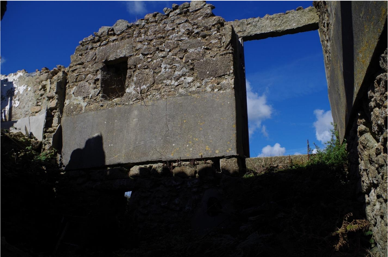
54. B1E, NORTH FF ELEVATION, W14 SLIT VENT AND D11.
