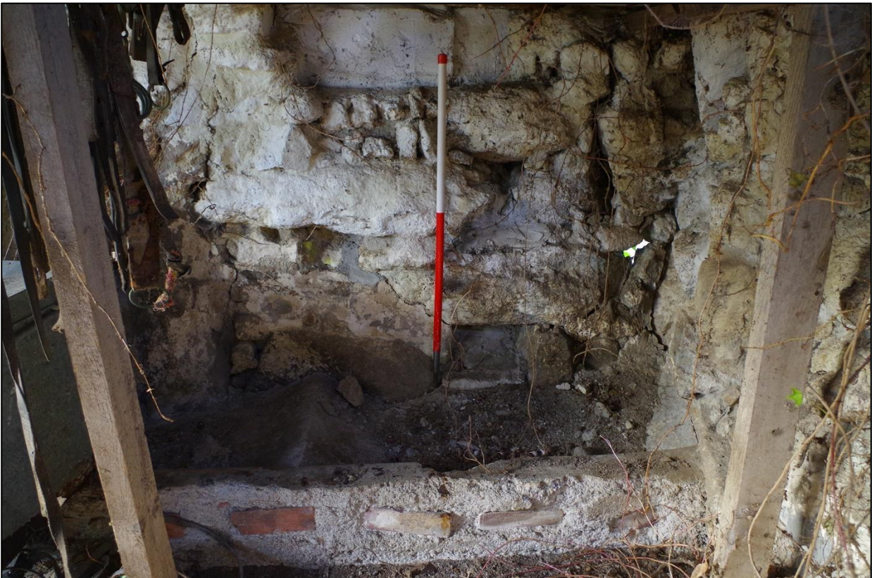
101. B3 SOUTH-WEST CORNER AND REBUILD OF FEED TROUGH, WITH BLOCKED OPENING TO EAVES ABOVE; VIEWED FROM THE NORTH (1M SCALES).
