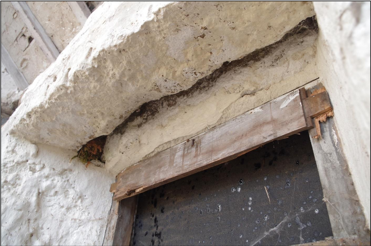
78. B2A, GRANITE LINTEL UNFACED TO W17, WITH ORIGINAL SLATTED TIMBER WINDOW.
