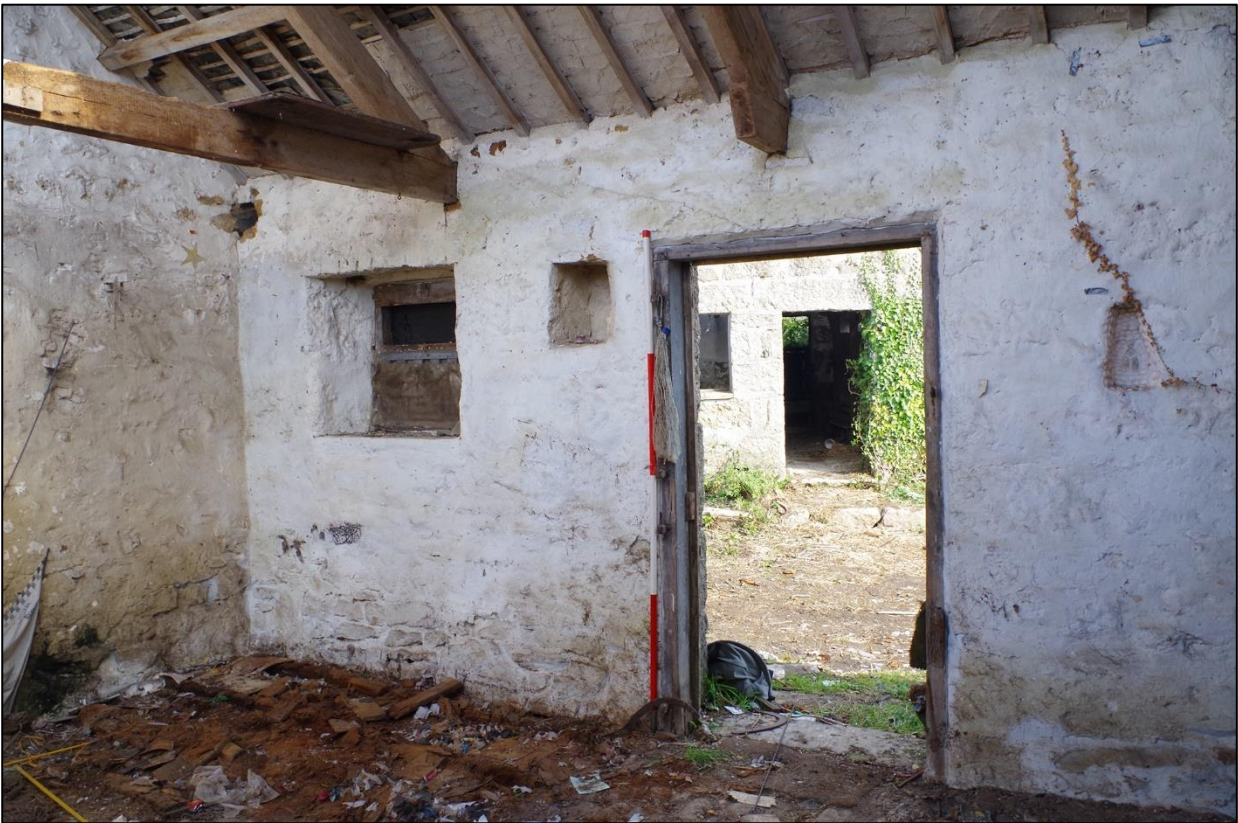
70. THE NORTH-WEST CORNER OF B2A; VIEWED FROM THE SOUTH-EAST (SCALE 2M).
