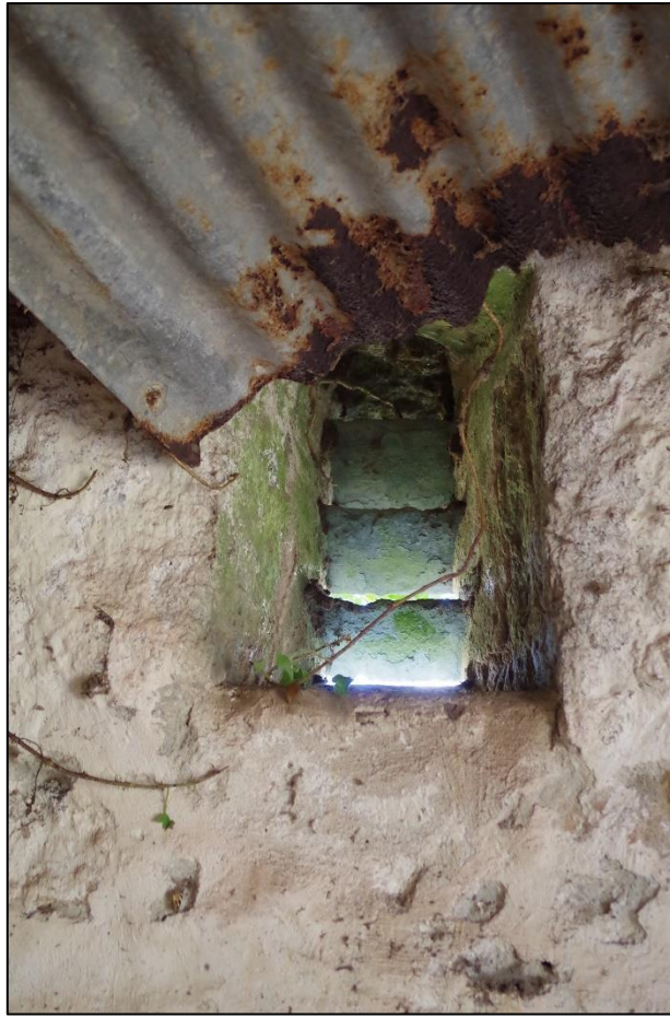
90. B2B SLIT VENT WITH SLATE LOUVRES TO THE WEST WALL.
