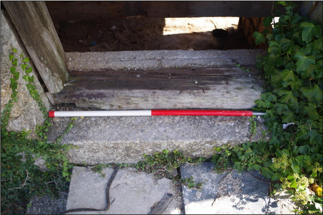
58. B1C, D12 GRANITE THRESHOLD; VIEWED FROM ABOVE (SCALE 1M).
