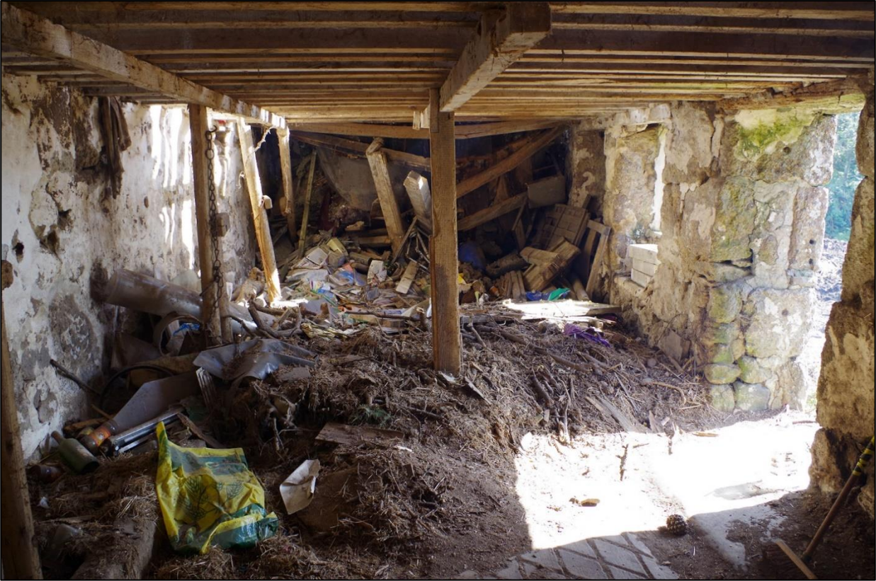
42. B1D, EAST END WAS INACCESSIBLE/UNSAFE; VIEWED FROM THE WEST.
