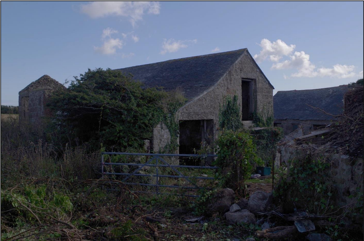
1. B1, NORTH AND WEST ELEVATION; VIEWED FROM THE NORTH-WEST. B2 ROOF TO REAR, AND B3 SOUTH OF GATE.
