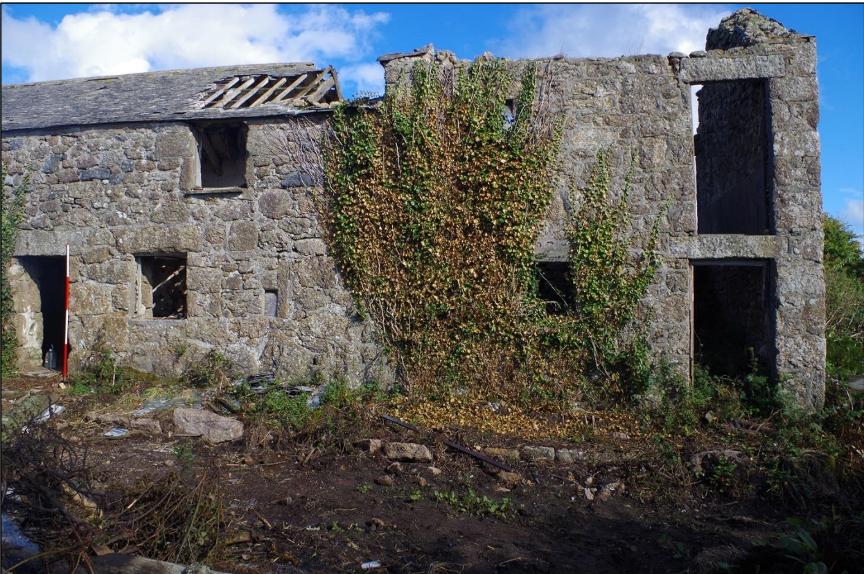
12. B1, EAST END OF SOUTH ELEVATION, SHOWING RAISE; VIEWED FROM THE SOUTH (SCALE 2M).
