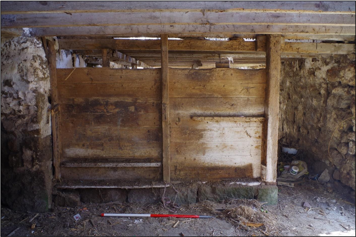
30. B1C, EAST TIMBER PARTITION WALL; VIEWED FROM THE WEST (SCALE 1M).
