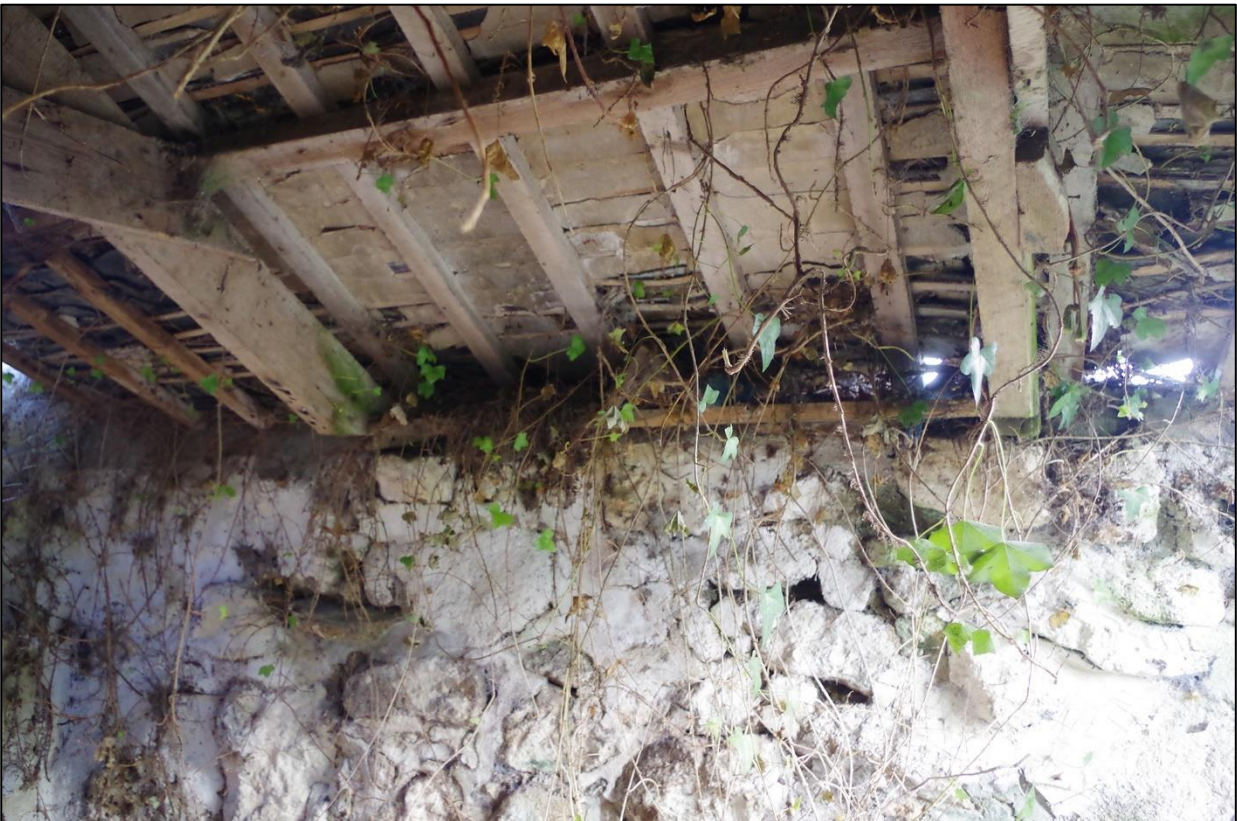
105. B3 NORTH EAVES, VIEWED FROM THE SOUTH-WEST.
