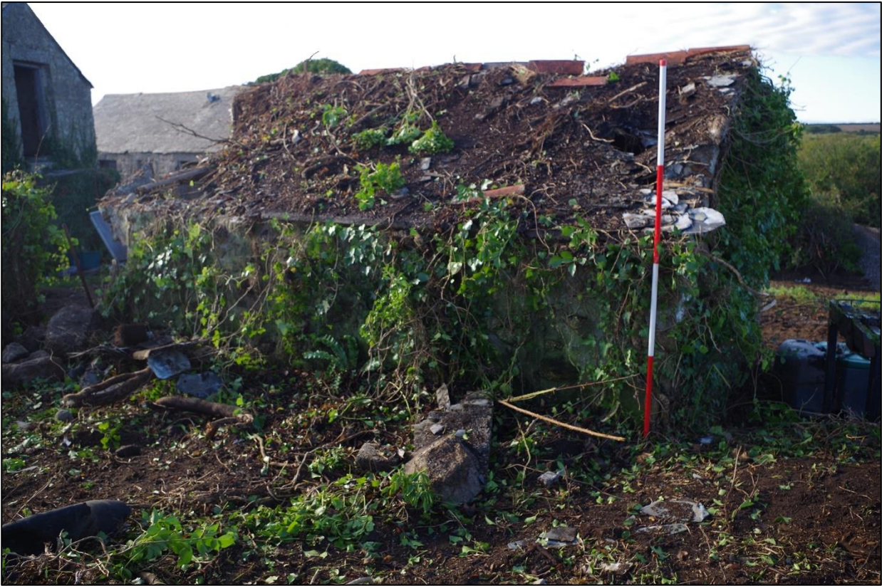
94. B3, NORTH ELEVATION TERRACED INTO BANK; VIEWED FROM THE NORTH-WEST (SCALE 2M).
