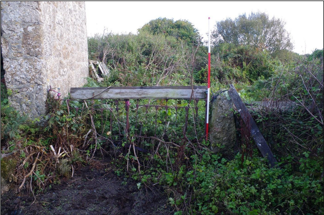
16. FORMER GATE TO OVERGROWN NORTHERN ENCLOSURES, WITH ROUGH GRANITE POST TO EAST SIDE AND REUSED BED FRAMES FOR GATE; VIEWED FROM THE SOUTH (SCALE 2M).
