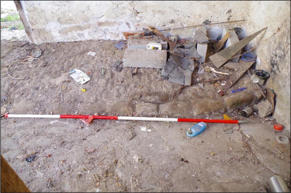
80. B2A, NORTH-EAST CORNER, WITH SPLIT SLATE DRAIN SLOPING TO EAST WITH GRANITE BLOCKS; VIEWED FROM THE SOUTH (SCALE 2M).
