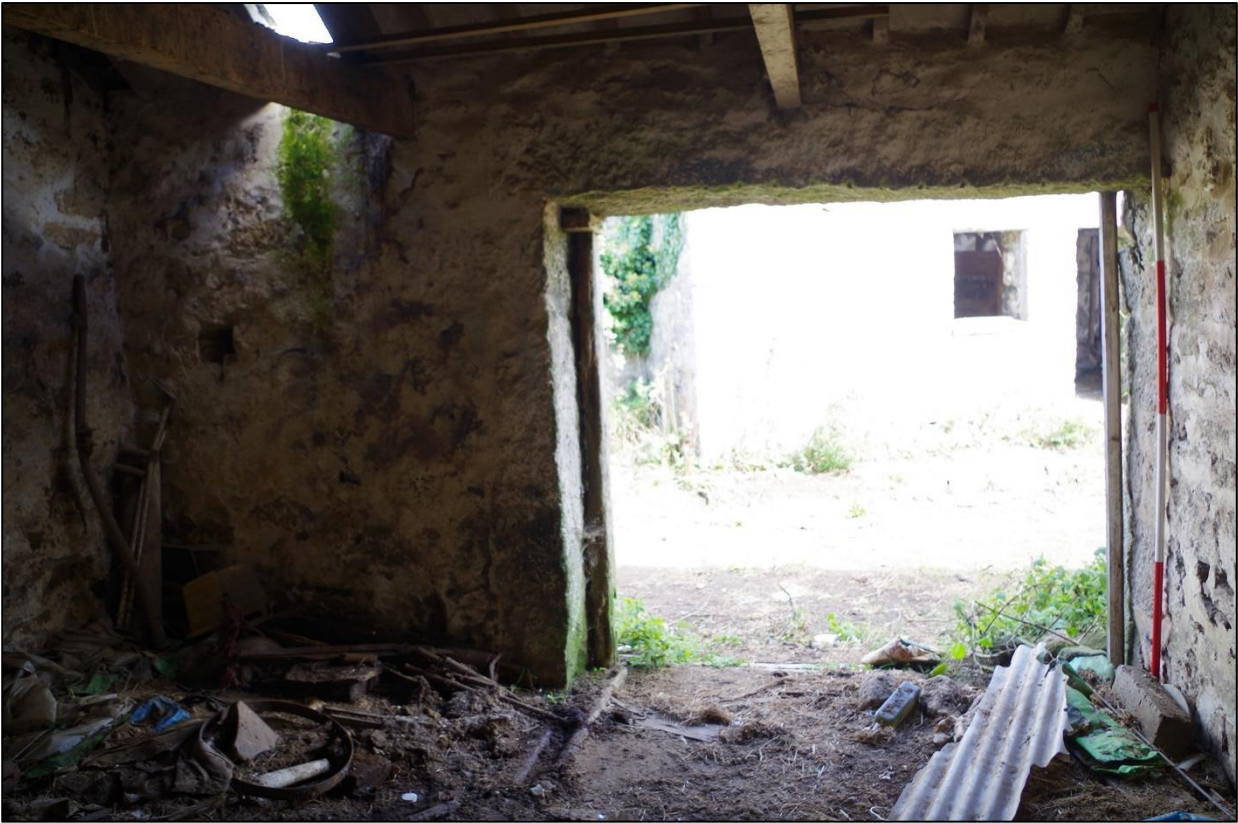
86. B2B, NORTH ELEVATION AND D14; VIEWED FROM THE SOUTH (2M SCALES).
