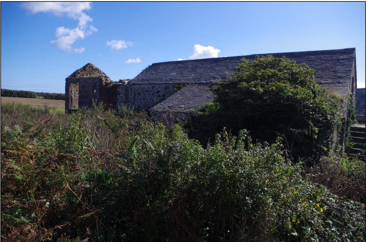
2. NORTH ELEVATION VIEWED FROM WHERE POSSIBLE; VIEWED FROM THE NNW.
