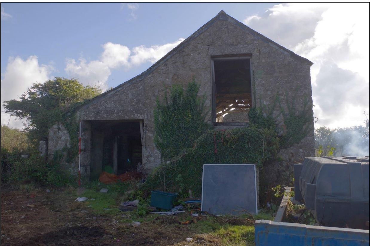
4. B1 WEST GABLE END AND B1A WEST ELEVATION; VIEWED FROM THE WEST (SCALE 2M).
