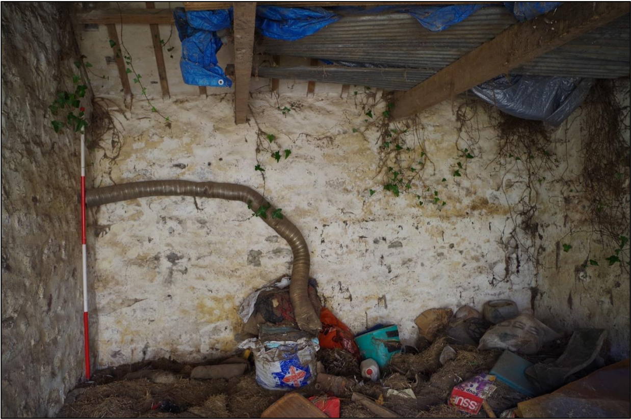
88. B2B THE SOUTH INTERNAL ELEVATION; VIEWED FROM THE NORTH (2M SCALES).
