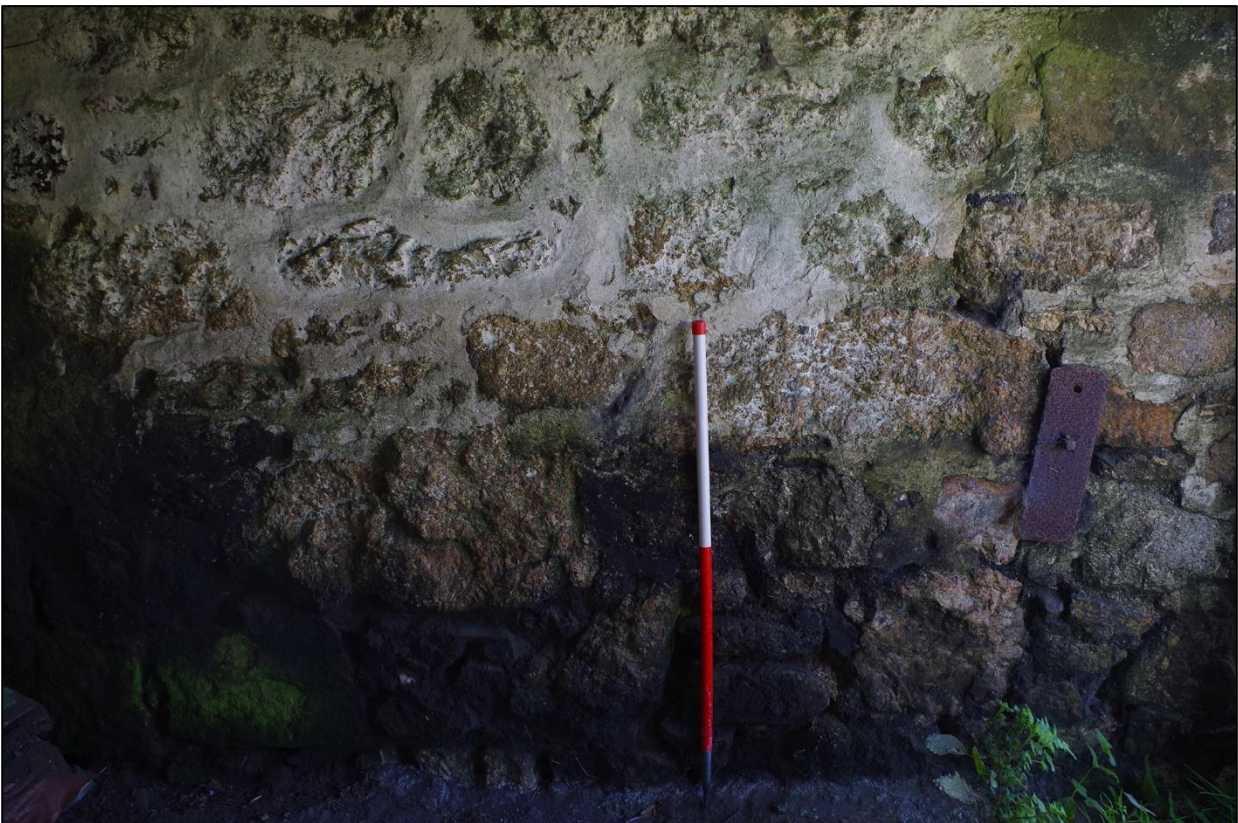
19. SOUTH INTERNAL WALL OF B1A; VIEWED FROM THE NORTH (SCALE 1M).
