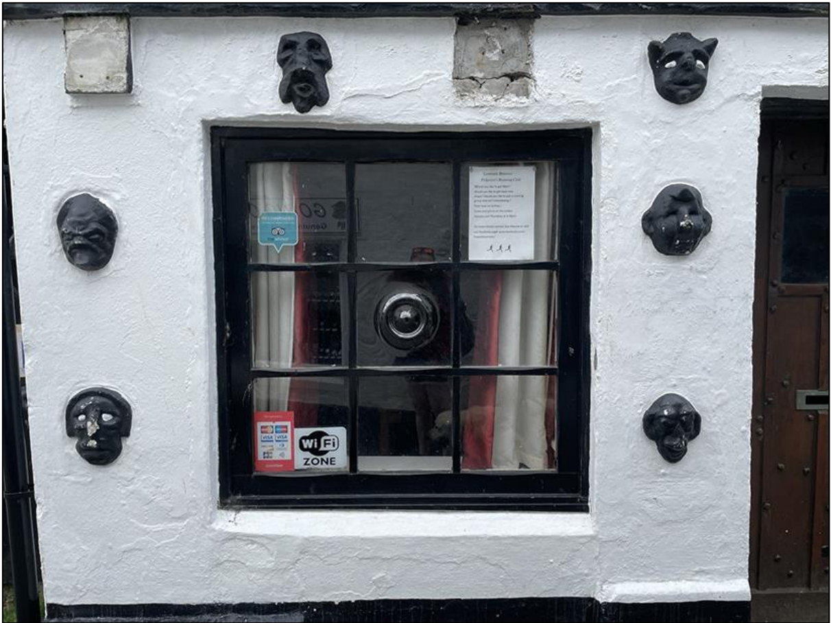
FIGURE 8: WINDOW 3 – A MID-LATE 20 TH CENTURY REPLACEMENT, SURROUNDED BY LATER GOTHIC DÉCOR TO IMITATE PIRATE THEME. THE TIMBER FRAME WAS NOTABLY PLAIN, AND THE OPENING HAS LIKELY BEEN ENLARGED, OR SITS WITHIN A BLOCKED DOORWAY.
