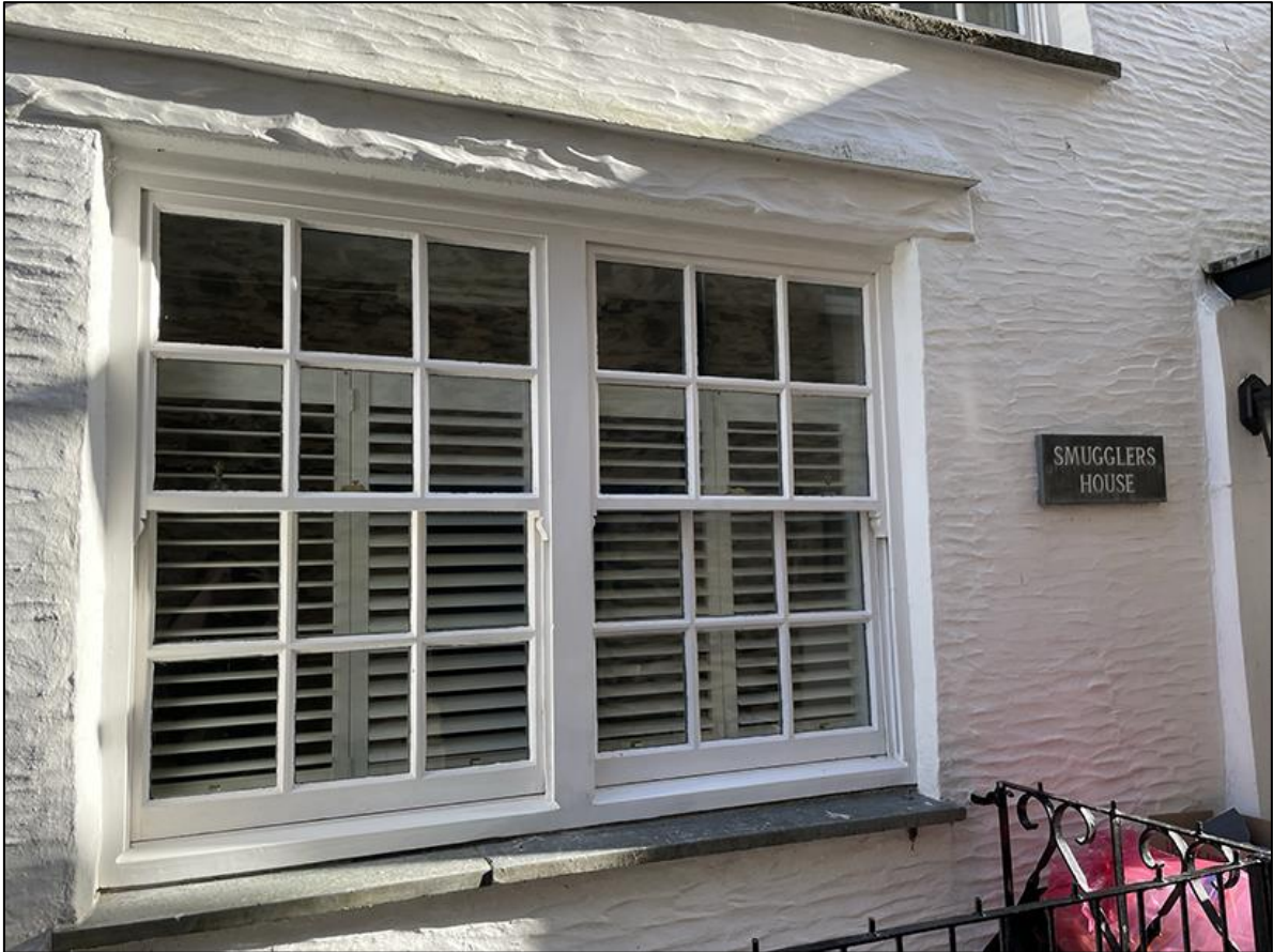
3. GOOD EXAMPLE OF HERITAGE-STYLE REPLACEMENT WINDOWS FURTHER WITHIN THE CONSERVATION AREA OF POLPERRO.
