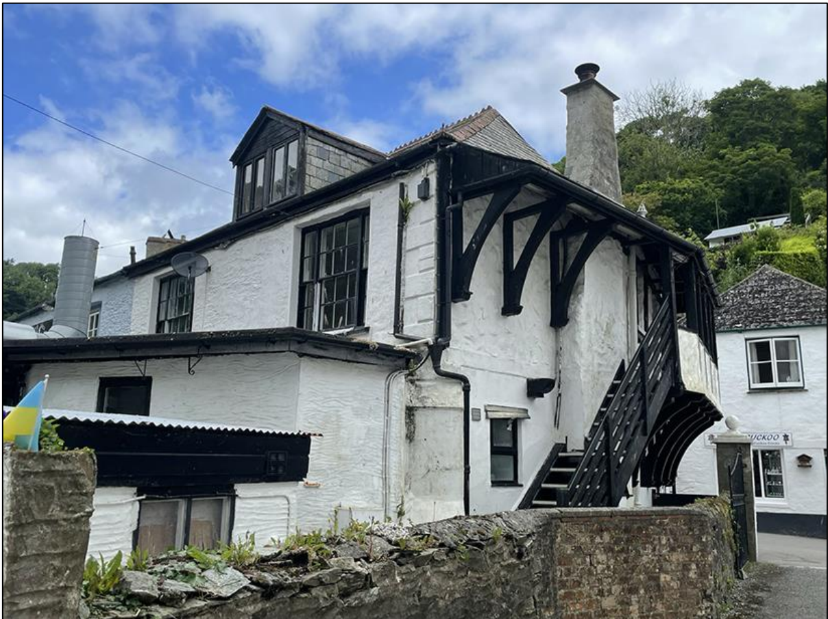
FIGURE 12: THE SOUTH-WEST ELEVATION AND THE TWO TRI-PARTITE SASH WINDOWS, VIEWED FROM THE SOUTH.
