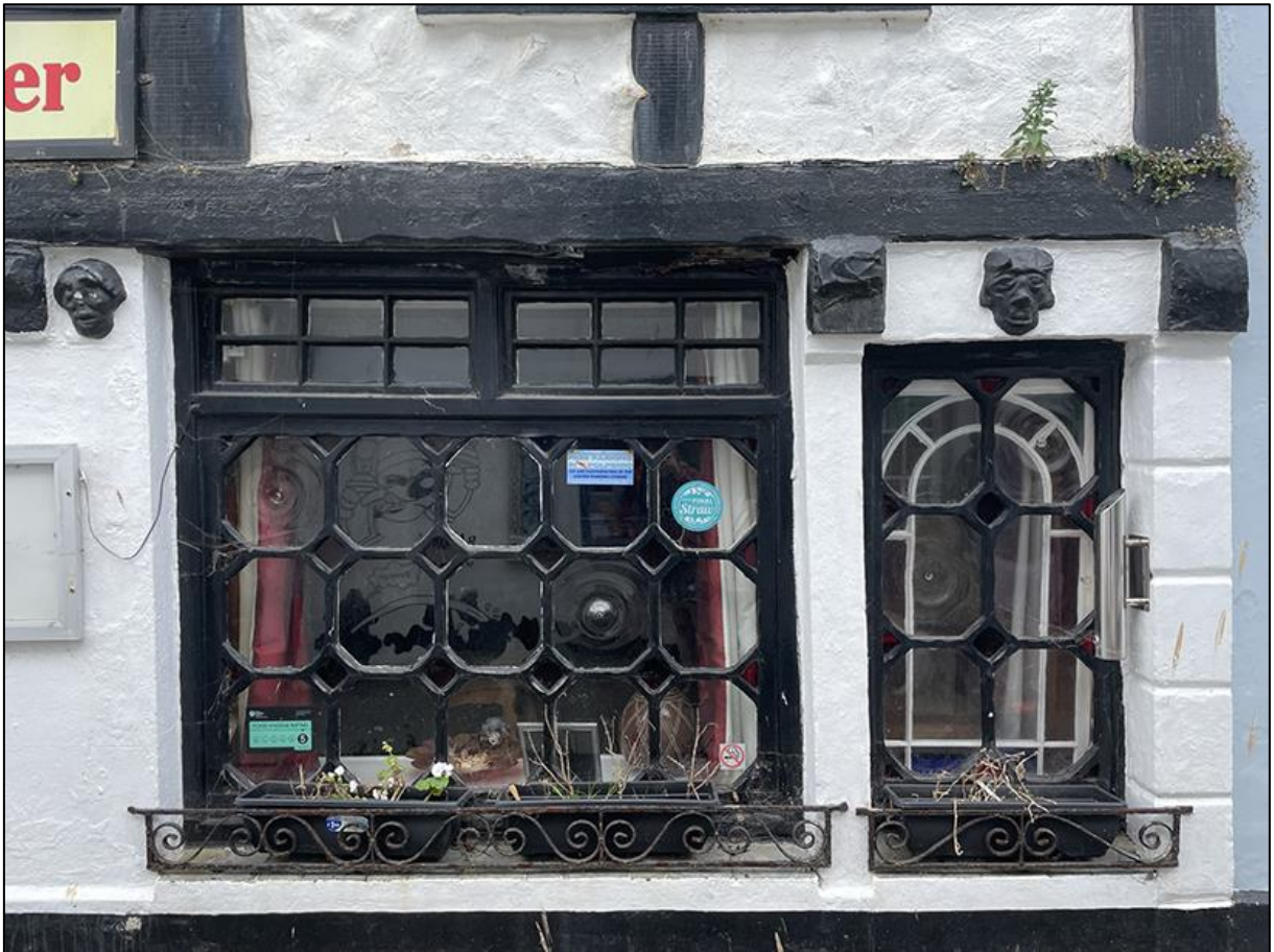
FIGURE 9: THE GF 15-PANE CENTRAL WINDOW AMONGST MEDIEVALIST GARGOYLE DECOR, AND THE SMALLER 6-PANED WINDOW TO THE EAST WITH AN INTERNAL VICTORIAN STAINED-GLASS, ROUND-HEADED WINDOW, VIEWED FROM THE STREET.
