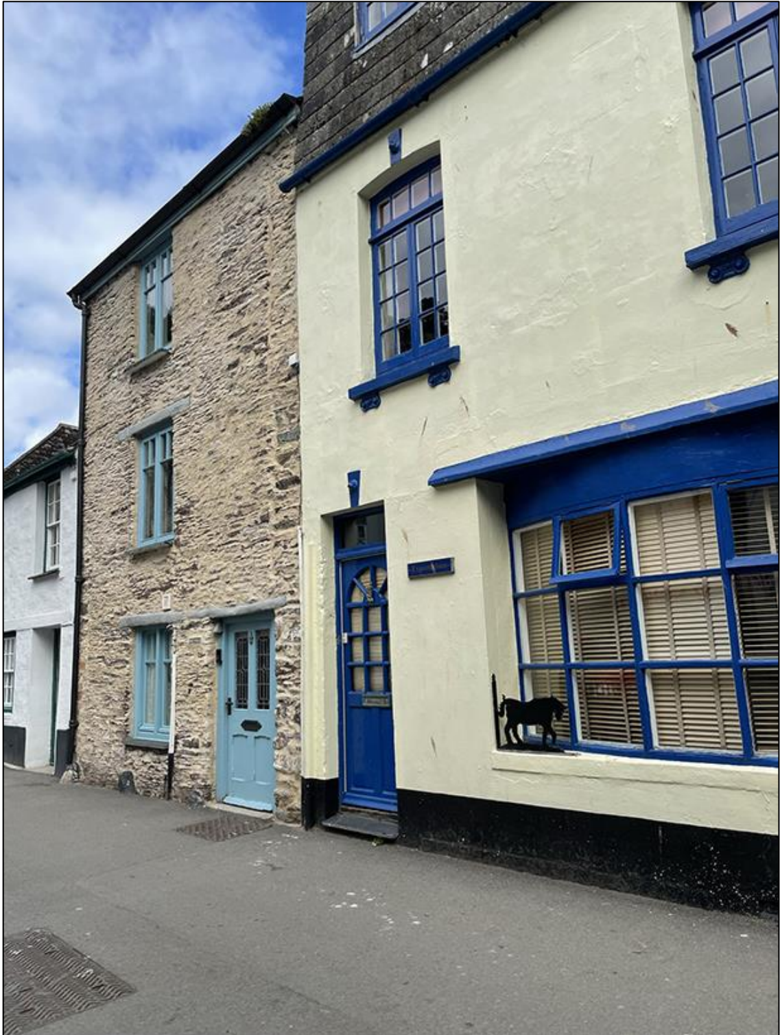
2. PROPERTIES OPPOSITE THE BUCCANEER RETAINING ORIGINAL WINDOWS.
