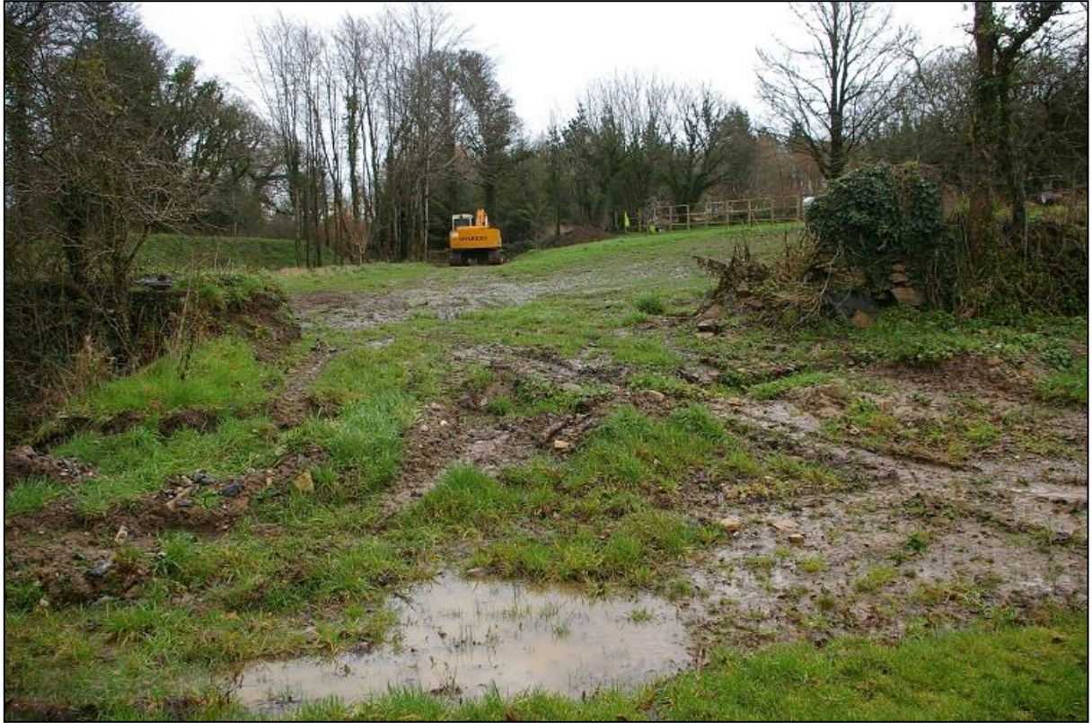
13. VIEW FROM THE FIELD THROUGH THE LARGE BREACH IN THE HEDGE BANK, WITH THE FRAGMENTARY RUINED BUILDING TO THE RIGHT AND CLEARANCE OF THE AREA WITHIN THE BOTTOM OF THE GARDENS; FROM THE WEST.
