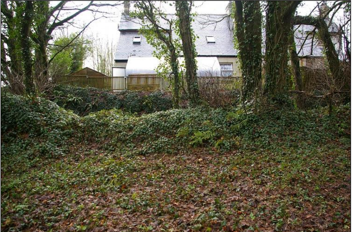
4. VIEW TO THE SLUMPED HEDGE BANK WHICH WILL BE BREACHED TO PROVIDE A NEW ENTRANCE TO THE NEW DRIVEWAY; FROM THE NORTH.
