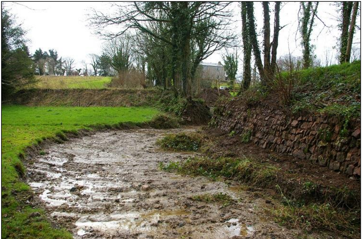
8. VIEW OF THE LOWER DRIVE, WHERE A TARMAC SPUR HAS ALREADY BEEN REMOVED AND THE HEDGE BANK BREACHED; FROM THE NORTH-EAST.
