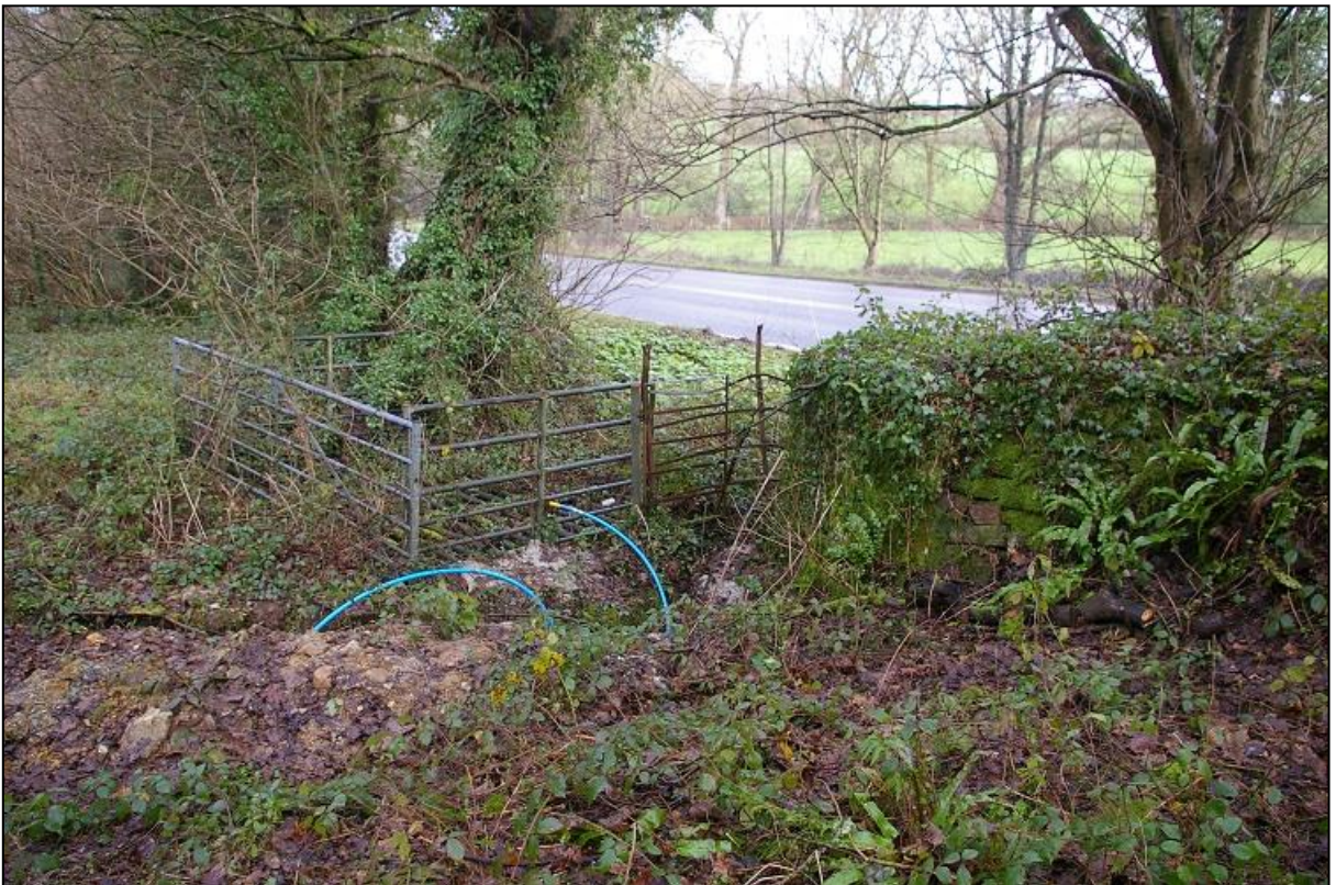
6. THE FORMER MAIN CARRIAGE DRIVE ENTRANCE INTO THE SITE, BLOCKED WITH A RANGE OF LOOSELY TIED GALVANISED GATES; FROM THE SOUTH-WEST.
