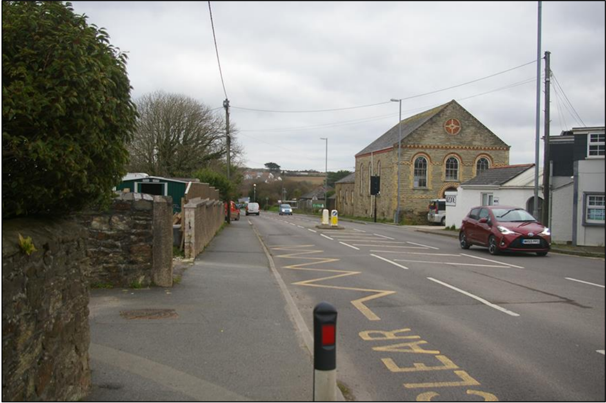
11. ROADSIDE VIEW OF GOONHAVERN METHODIST CHURCH, DEMONSTRATING LOCAL SCREENING; VIEWED FROM THE WEST-SOUTH-WEST.
