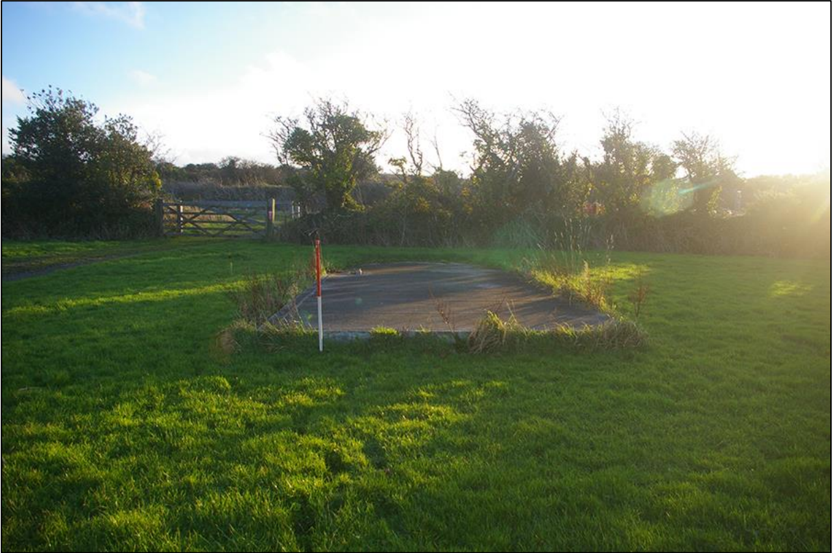
19. F2, DETAIL OF A MODERN CONCRETE PAD; VIEWED FROM THE NORTH (1M SCALE).
