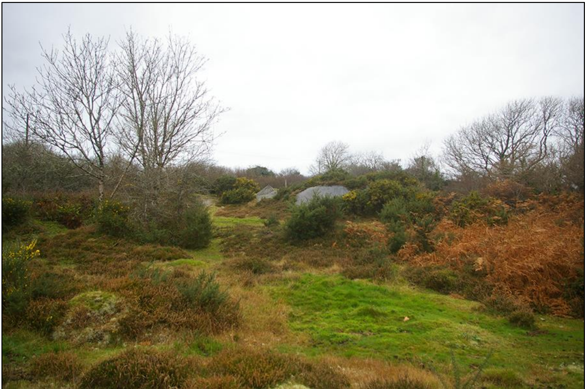
2. VIEW TOWARDS THE AREA OF THE MAPPED NORTH CHIVERTON ENGINE HOUSES, THOUGH NO REMAINS WERE VISIBLE, DEMONSTRATING SPOIL MOUNDS AND CAPPED SHAFT AS WELL AS SCRUB REGENERATION; VIEWED FROM THE SOUTH-SOUTH-EAST.
