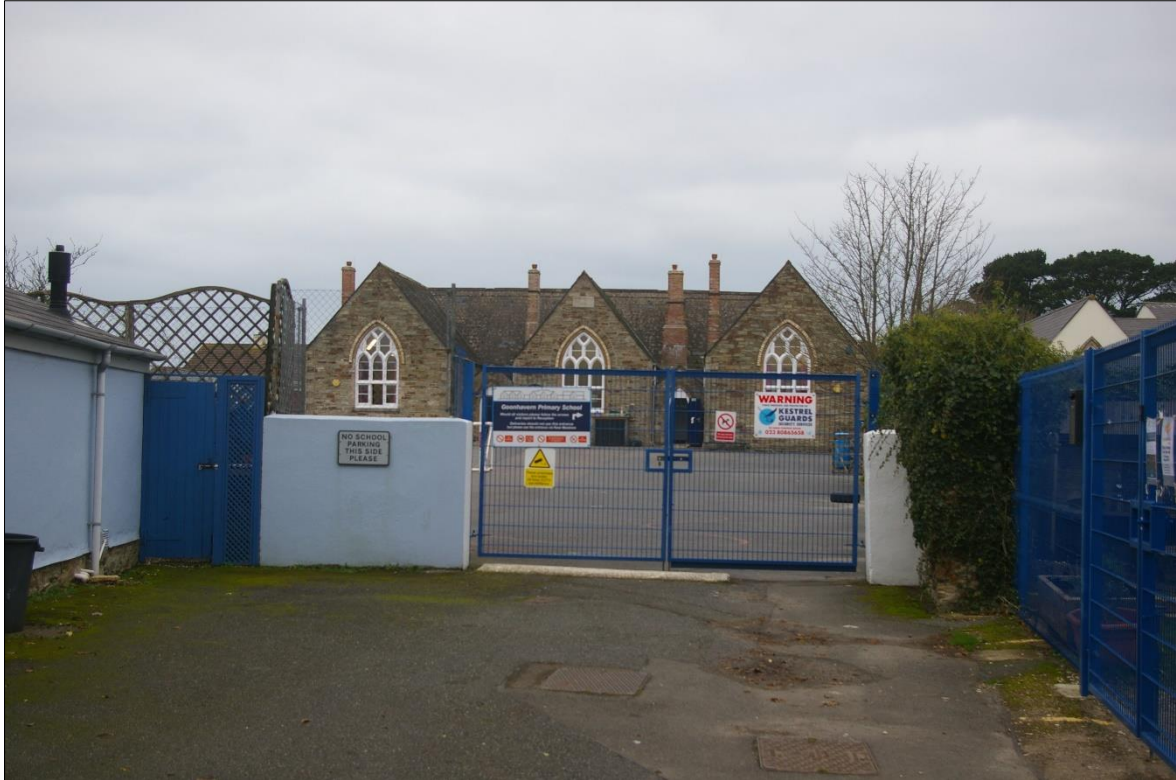
FIGURE 19: GOONHAVERN COUNTY PRIMARY SCHOOL; VIEWED FROM THE SOUTH-EAST.
