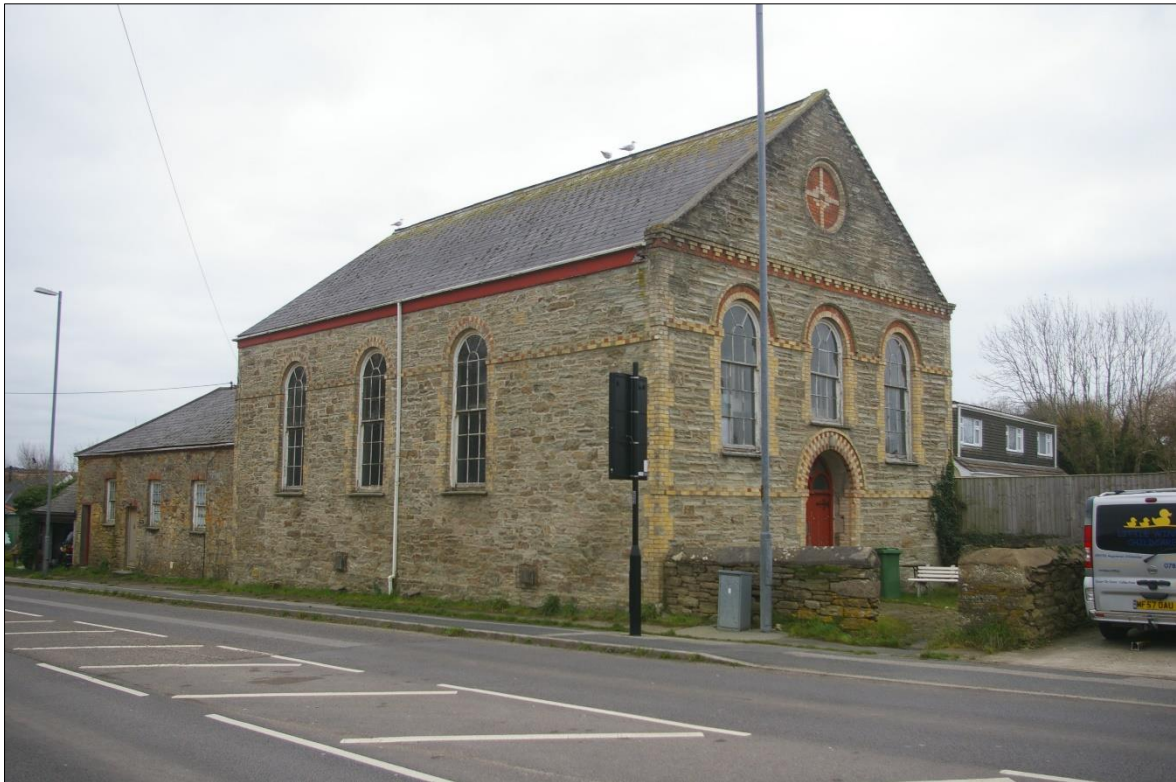
FIGURE 20: GOONHAVERN METHODIST CHURCH; VIEWED FROM THE WEST.
