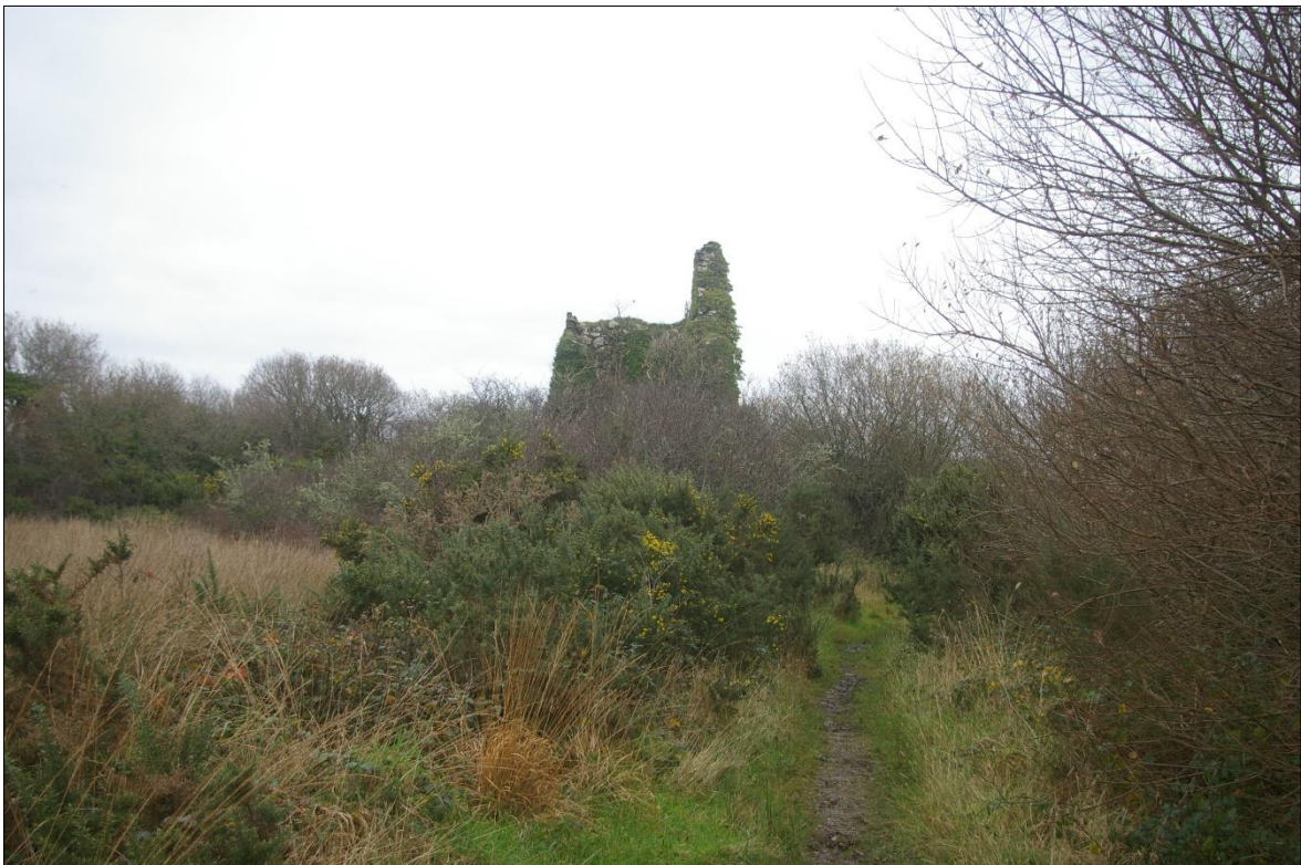
FIGURE 17: THE ENGINE HOUSE AT WHEAL ALBERT; VIEWED FROM THE SOUTH-WEST.
