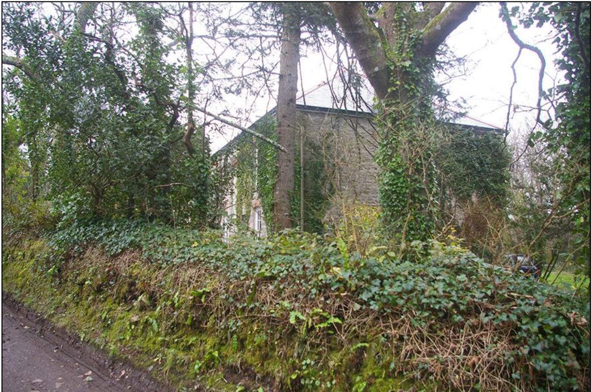
12. VIEW OF WHEAL ANNA HOUSE, LOOKING TOWARDS THE PROPOSAL SITE, DEMONSTRATING EXISTING LOCAL WOODLAND SCREENING; VIEWED FROM THE WEST-SOUTH-WEST.
