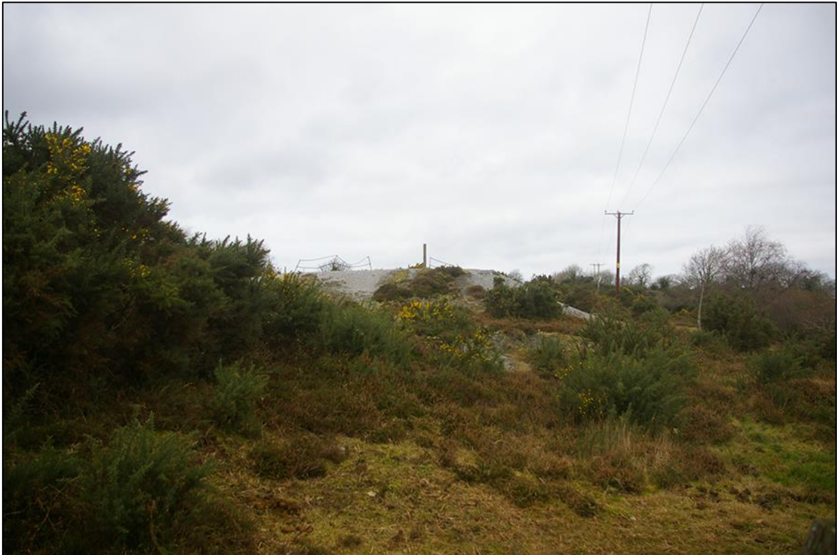
4. DETAIL OF THE SPOIL HEAPS AT THE NORTH CHIVERTON MINE SITE, DEMONSTRATING SCRUB REGENERATION; VIEWED FROM THE SOUTH-SOUTH-EAST.
