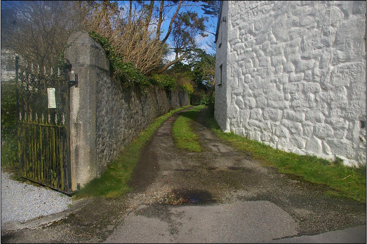
1. THE SERVICE DRIVE TO THE REAR YARD AT VOGUE HOUSE, WHICH CONTAINS THE OUTBUILDING.
