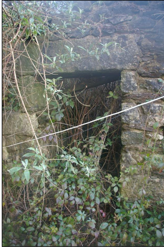
27. THE SECOND DOORWAY ON THE WEST ELEVATION OF BUILDING 2.
