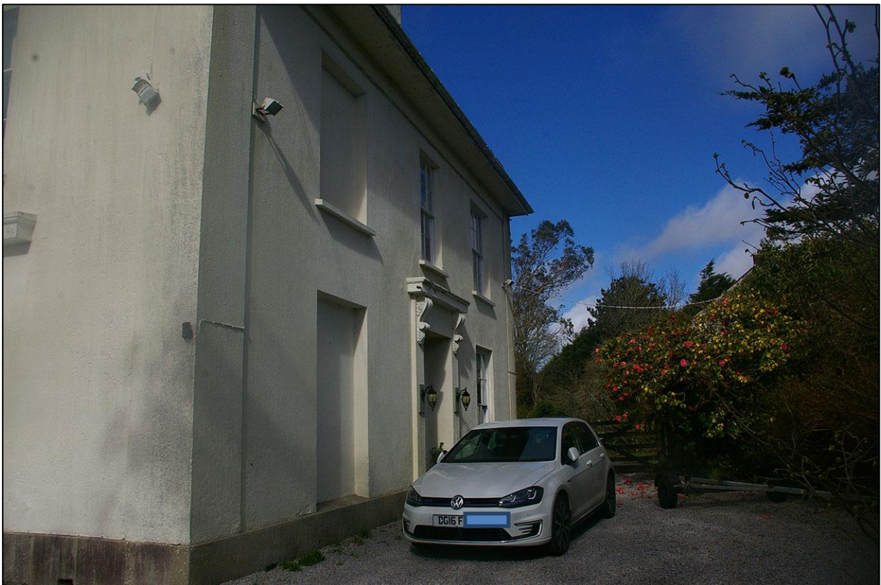
4. THE EAST ELEVATION OF VOGUE HOUSE, WITH MAIN ENTRANCE.
