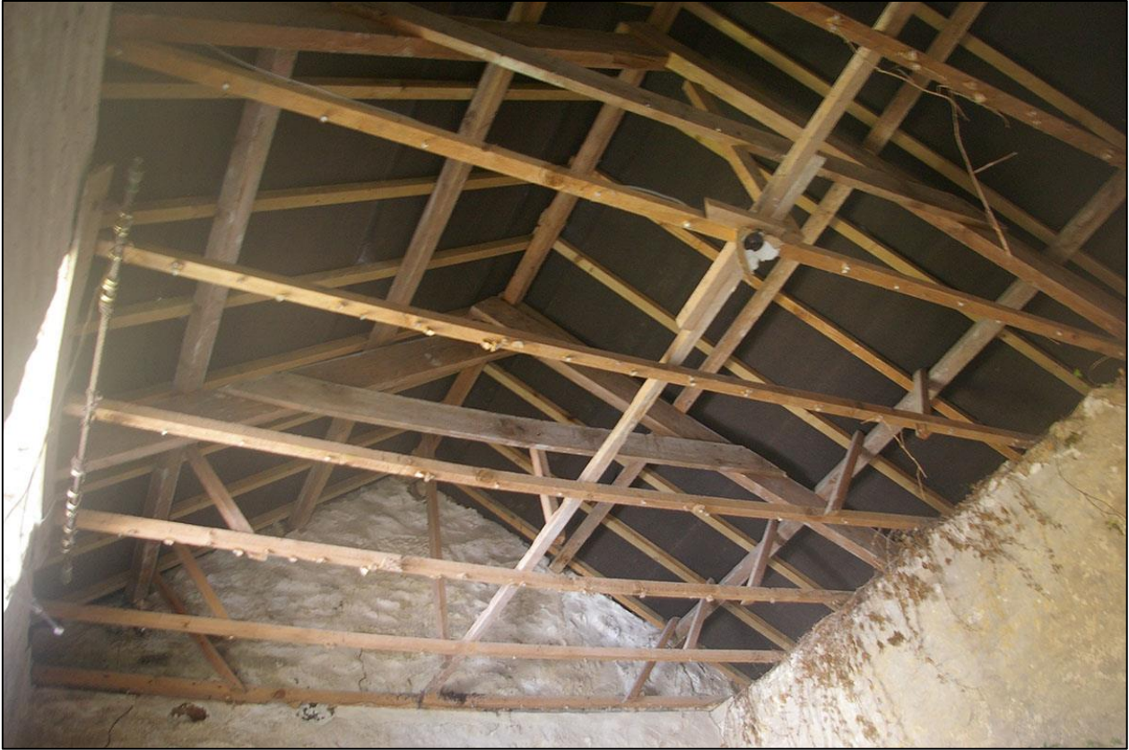
22. THREE BAY ROOF OVER SECTION B, BUILDING 1, WITH TWO TRUSSES.
