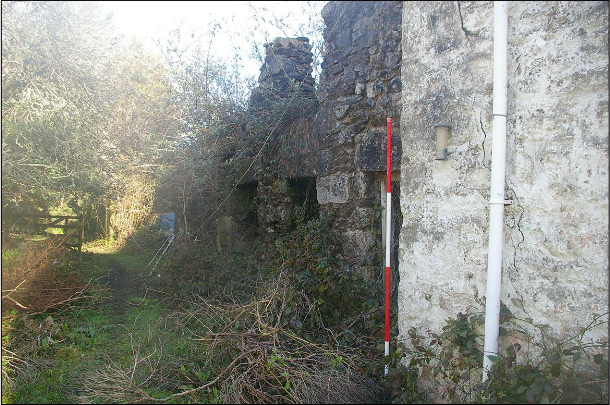
24. VIEW ALONG THE FRONT OF BUILDING 2, WITH 2M SCALE.
