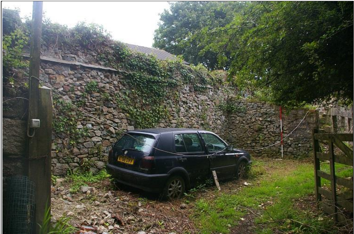
12. SECTION D, FORMER OPEN FRONTED BARN, BUILDING 2, WITH 2M SCALE; FROM THE NORTH-WEST.
