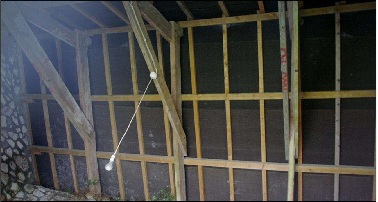
16. THE FOUR BAY ROOF OVER SECTION A, BUILDING 1, SHOWING THREE TRUSSES.
