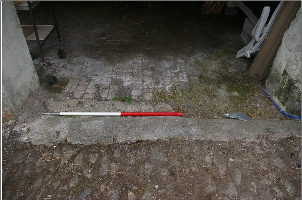
5. ONE OF THE ORIGINAL GRANITE THRESHOLDS TO THE PAVED FLOOR TO SECTION A, BUILDING 1; FROM THE WEST, WITH 1M SCALE.
