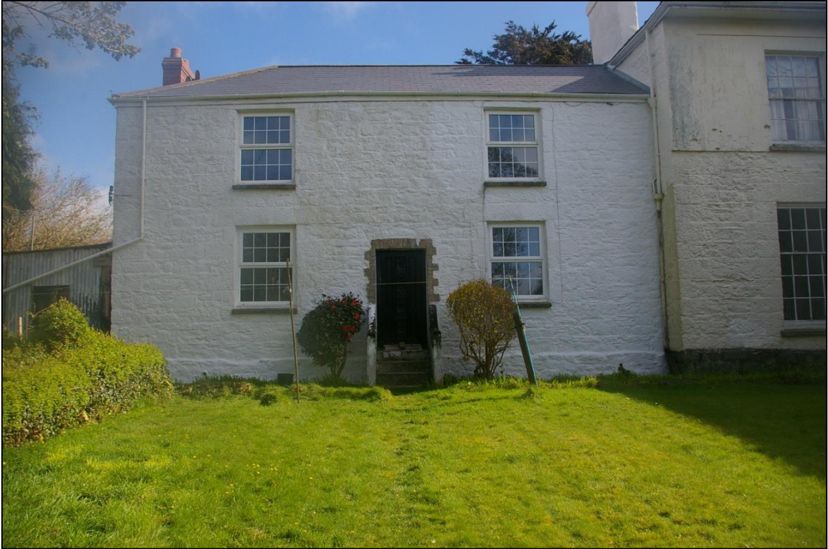
FIGURE 5: THE REAR NORTH WING OF VOGUE HOUSE, PARALLEL WITH THE SERVICE OUTBUILDING; FROM THE WEST.
