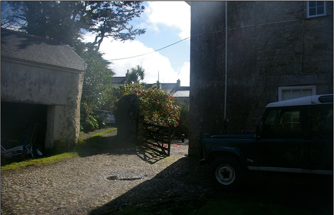
9. THE RELATIONSHIP BETWEEN THE OUTBUILDING, DRIVEWAY AND VOGUE HOUSE, WITH COBBLED COURTYARD.
