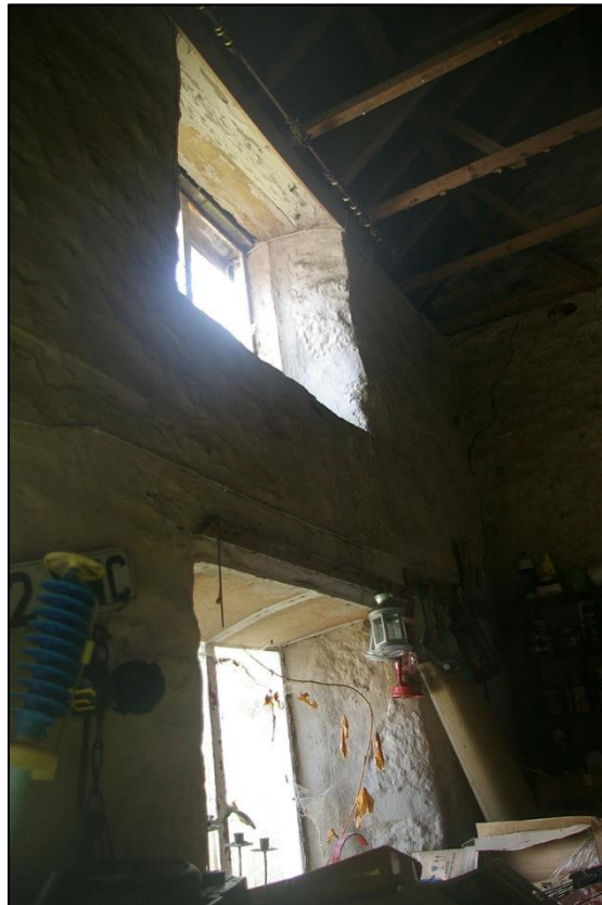
23. THE INTERIOR FACE OF THE WALL WITH W1 AND W2, SHOWING CURTAIN POLES, INDICATING DOMESTIC FUNCTION AT SOME POINT IN THE EARLY-MID 20TH CENTURY.
