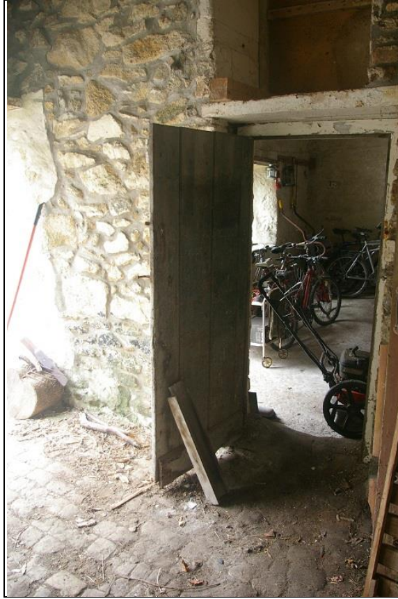
3. D2, THE PLANK DOOR BETWEEN SECTION A & B; FROM THE SOUTH-EAST.
