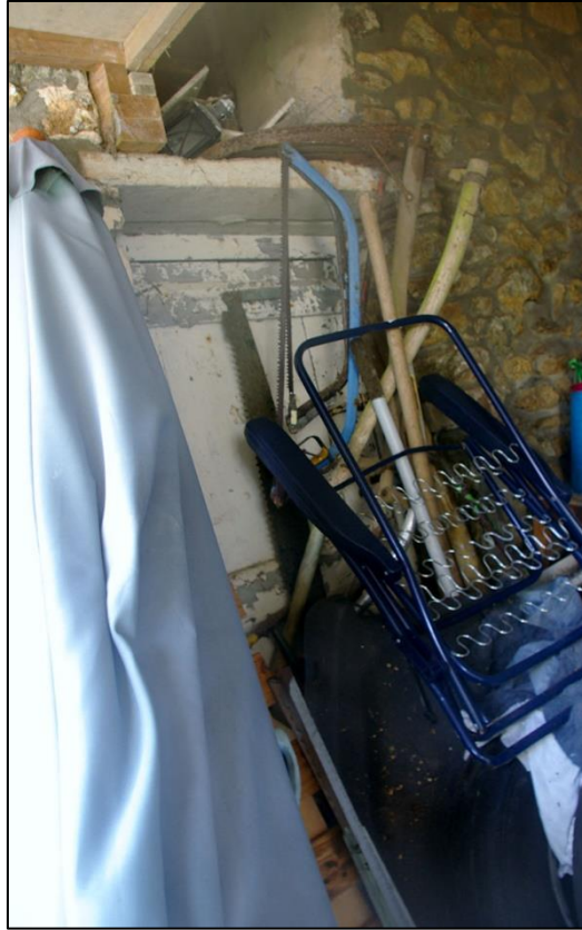
18. OBSCURED VIEW OF THE PLANK DOOR TO D2, SECTION A, BUILDING 1.
