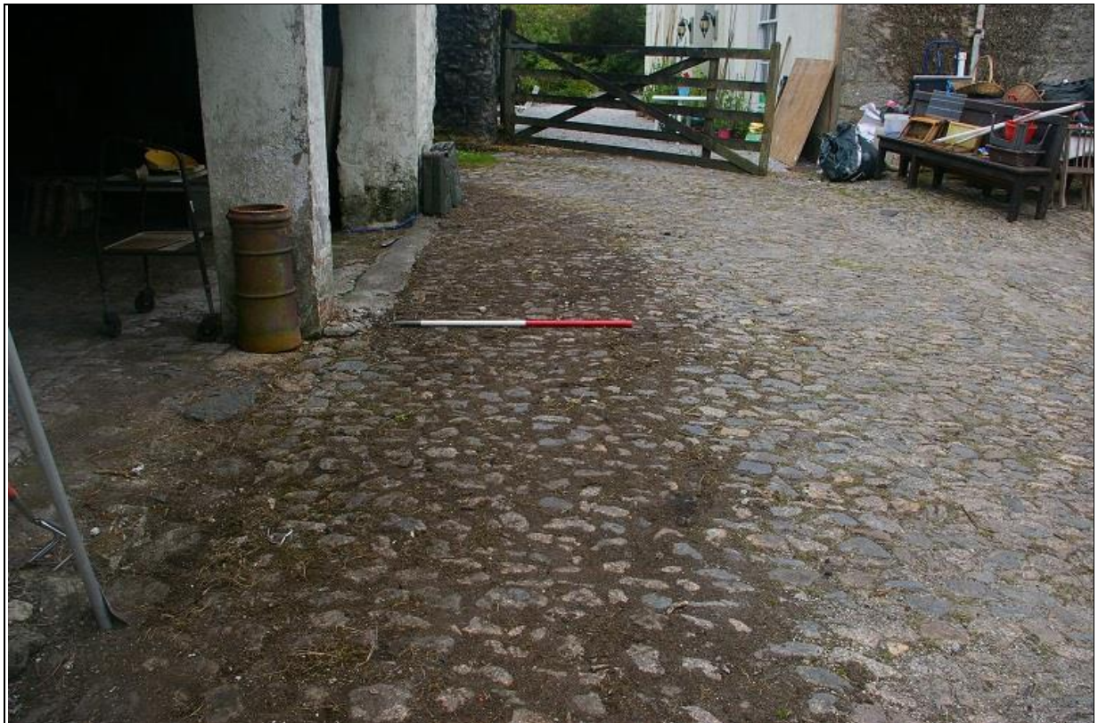
6. COBBLED COURTYARD AND FORMER THRESHOLD TO BUILDING 1, WITH 1M SCALE; FROM THE NORTH.
