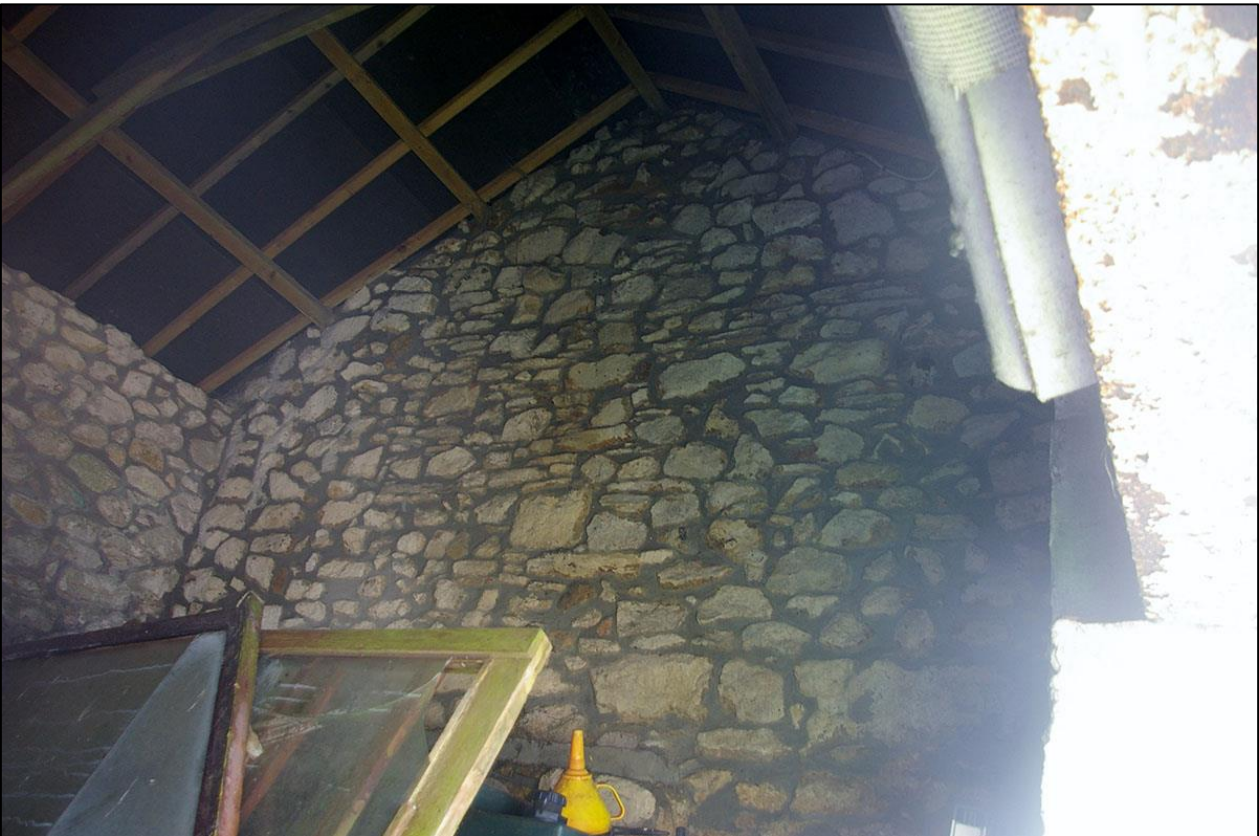
13. THE INTERIOR RE-POINTED FACE OF THE SOUTH GABLE.
