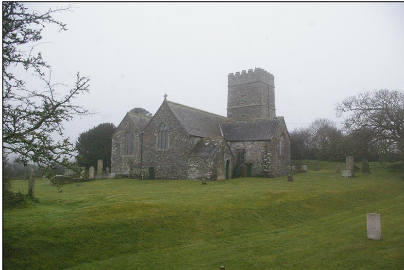
2. ST MICHAEL'S CHURCH ON ITS RAISED AREA; VIEWED FROM THE NORTH-EAST (NO SCALE).
