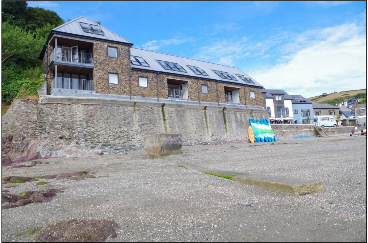
3. THE DOMINATING, RECENTLY RENOVATED FORMER FISH CELLAR – THE BAY. TAKEN FROM THE SOUTH-EAST. OCEAN WAVES CAN BE SEEN TO THE RIGHT.
