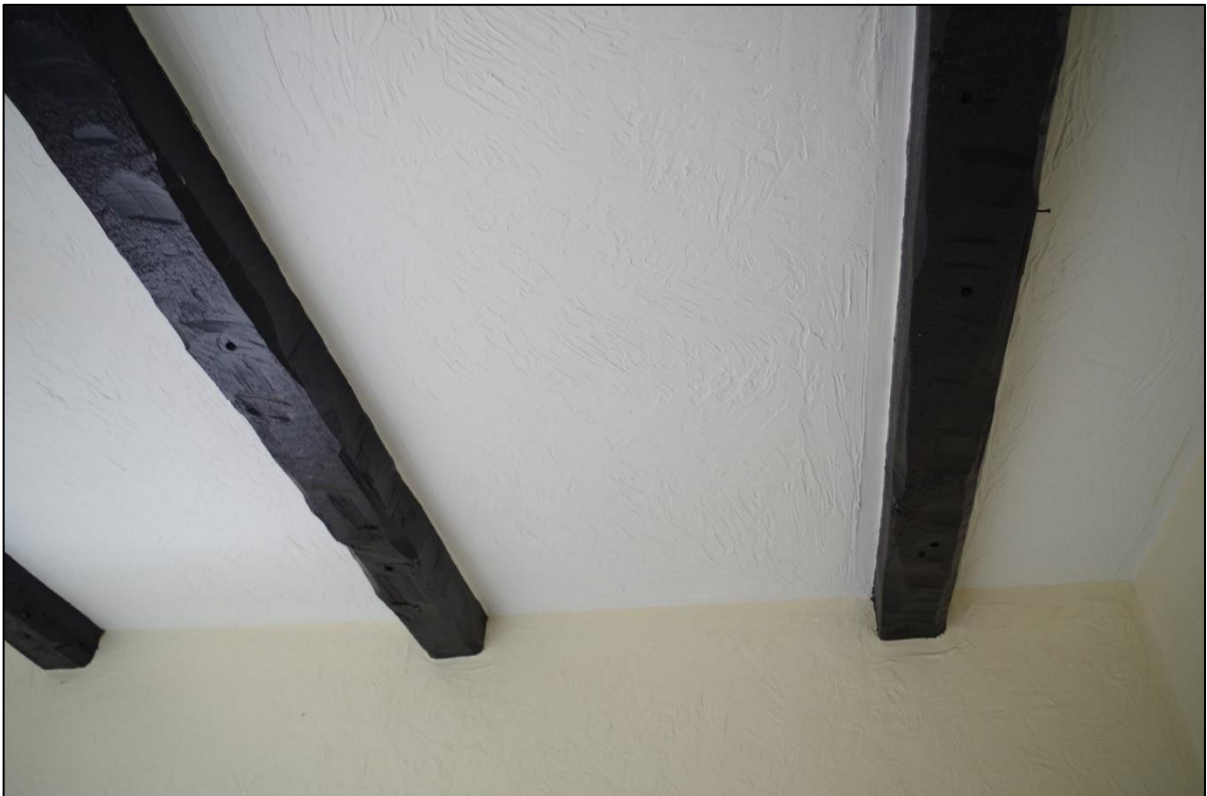
12. THE MOCK-STYLISED INTERNAL BEAMS, GIVING THE EFFECT THE BUILDING IS EARLIER.
