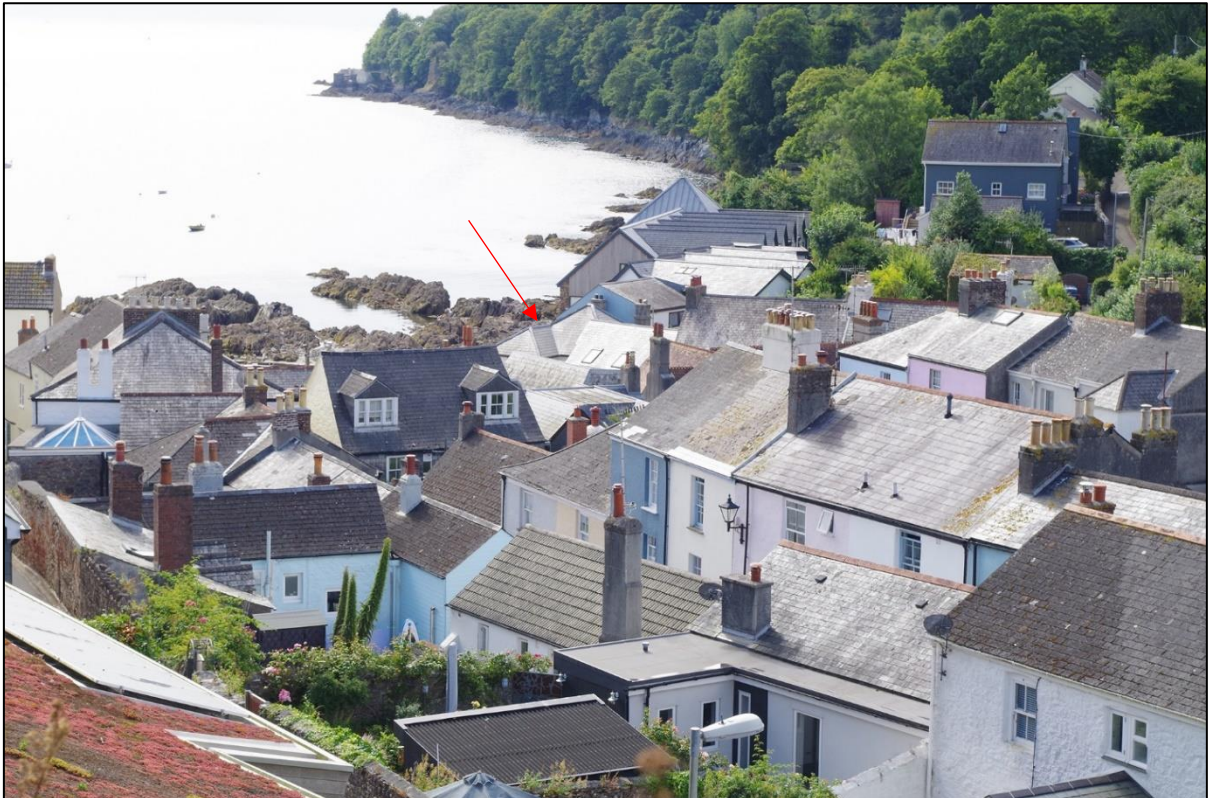
4. THE ROOFSCAPE OF CAWSAND, OCEAN WAVES CAN BE SEEN (ARROWED) ALONGSIDE MANY OTHER GABLED DORMERS AND VELUXES.
