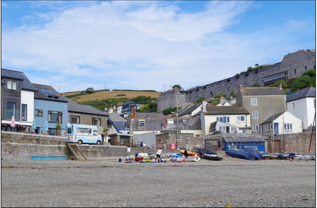
1. THE BOUND AND FRONT, TAKEN FROM THE SOUTH-EAST, CAWSAND FORT TO THE REAR.
