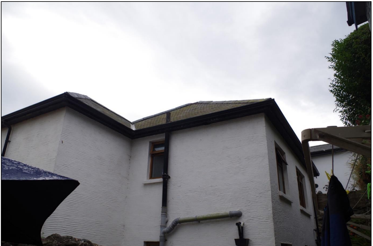
8. THE NORTH-WEST CORNER, WHICH WILL KNOCKED THROUGH TO CREATE AN EXTENSION; TAKEN FROM THE NORTH.
