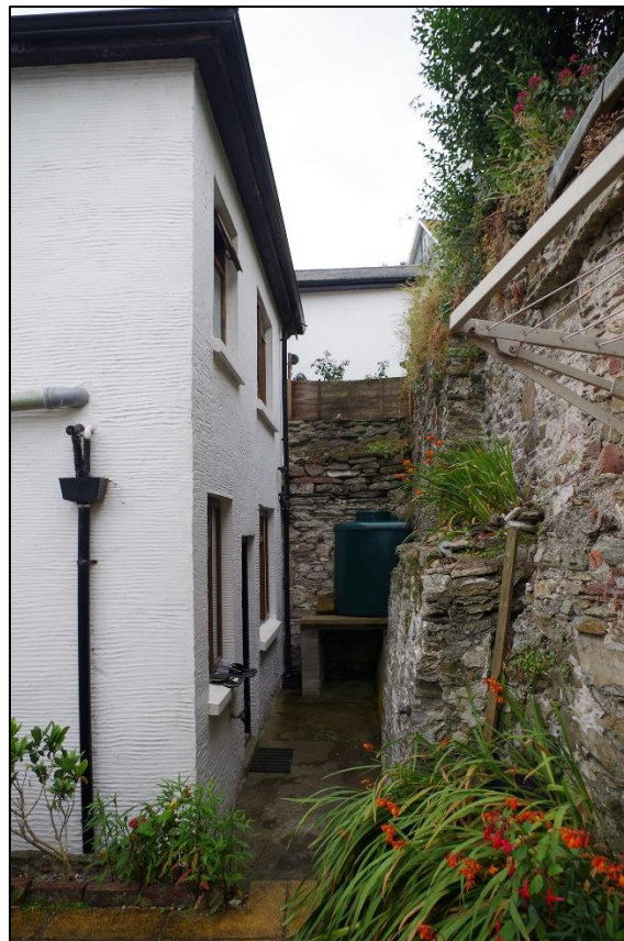
FIGURE 11: THE WEST ELEVATION AND WEST BOUNDARY WALL. TAKEN FROM THE NORTH.
