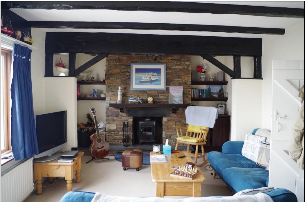
11. THE GROUND FLOOR LIVING ROOM, WITH ALTERED FIREPLACE, AND CHUNKY LINTEL POSSIBLY ARCHITECTURAL SALVAGE. TAKEN FROM NORTH.
