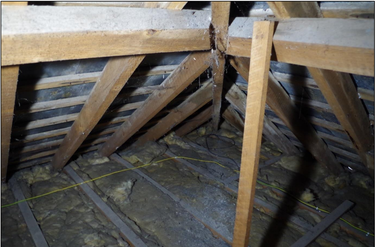
FIGURE 13: THIN TIMBER TIES PLOTTED IN THE CORNERS ATTACH THE ROOF STRUCTURE TO THE JOISTS.
