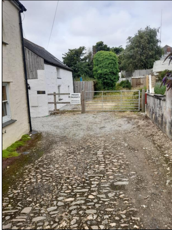
8. Cobbled trackway leading along the eastern side of Wellesley farmhouse (from the south). This would become the entrance into the proposed development.
