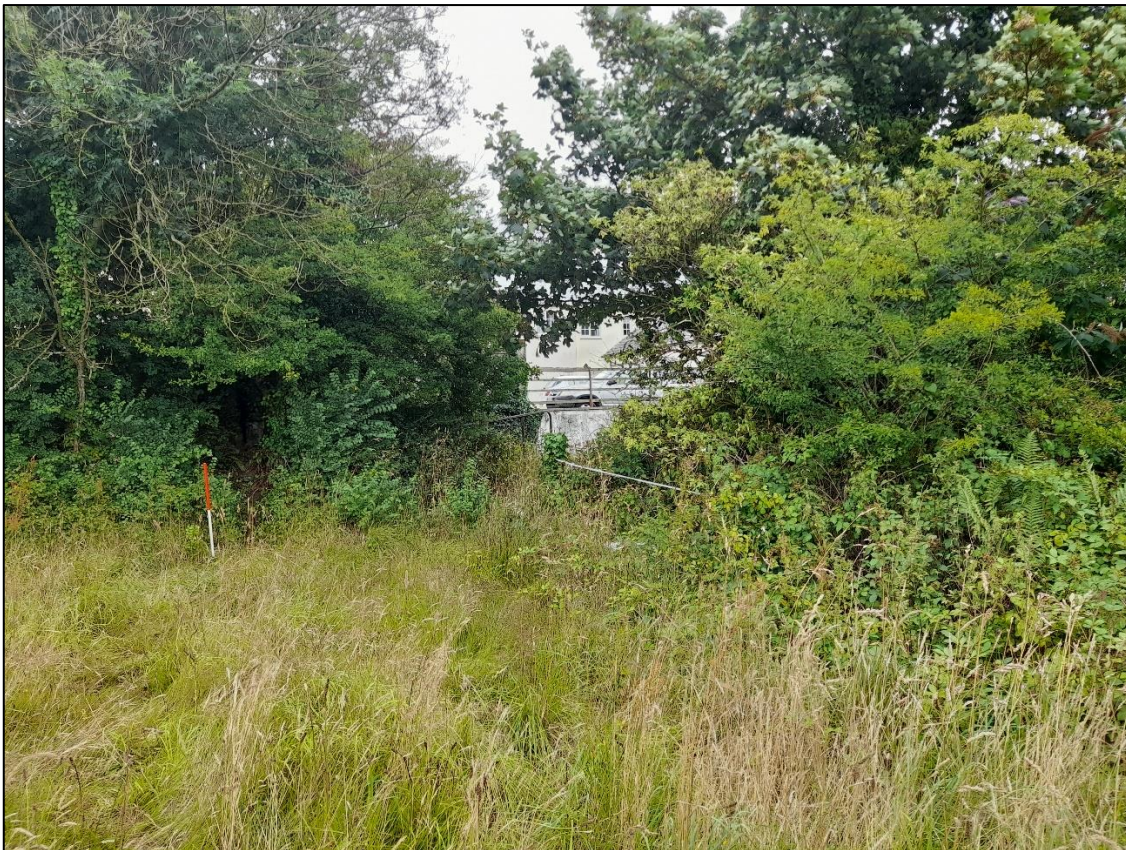
3. Boundary of development site showing modern galvanised gate.
