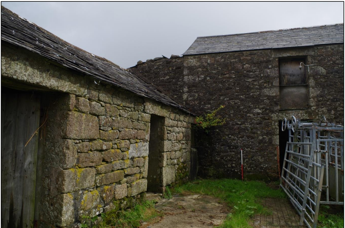
21. WEST ELEVATION SHOWING BUILDING 4 ABUTTING BUILDING 2; FROM THE WEST (1M SCALE).
