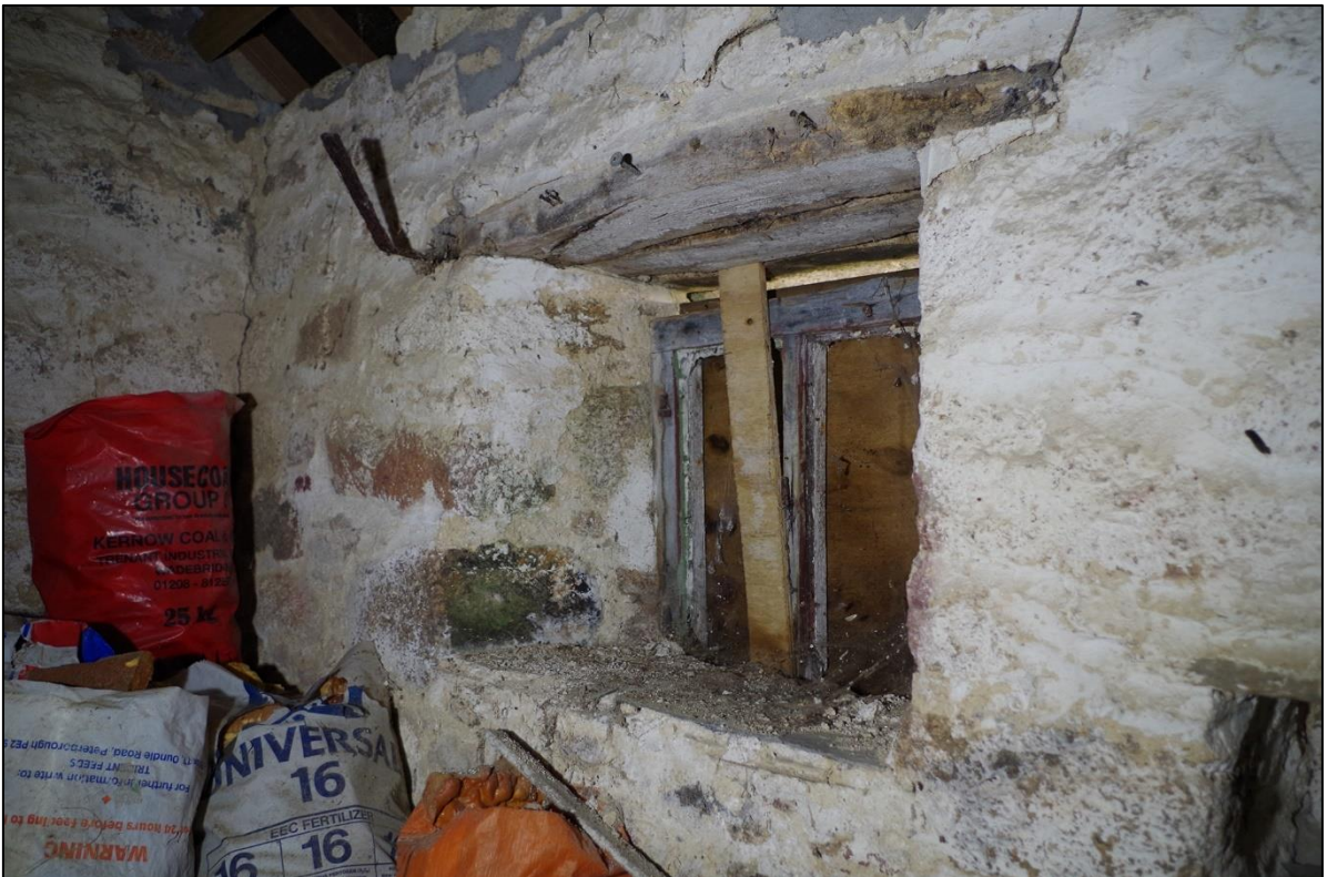
30. FF WINDOW W3 WITH RUSTIC TIMBER LINTEL, SLATE SILL AND REUSED DOMESTIC WINDOWS OF VICTORIAN CHARACTER; FROM THE SOUTH-WEST.
