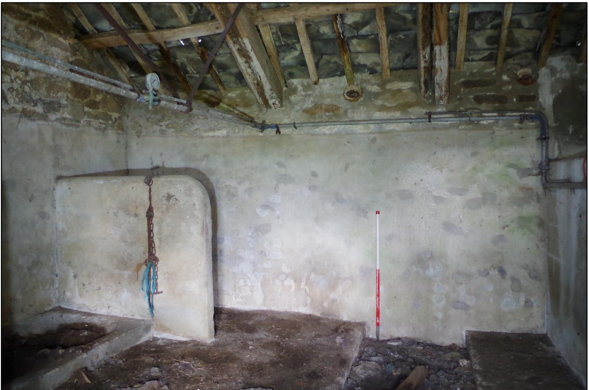
54. NORTH ELEVATION OF BUILDING 4A WITH TERRACOTTA VENTS AND RENDERED WALLS; FROM THE SOUTH (1M SCALE).
