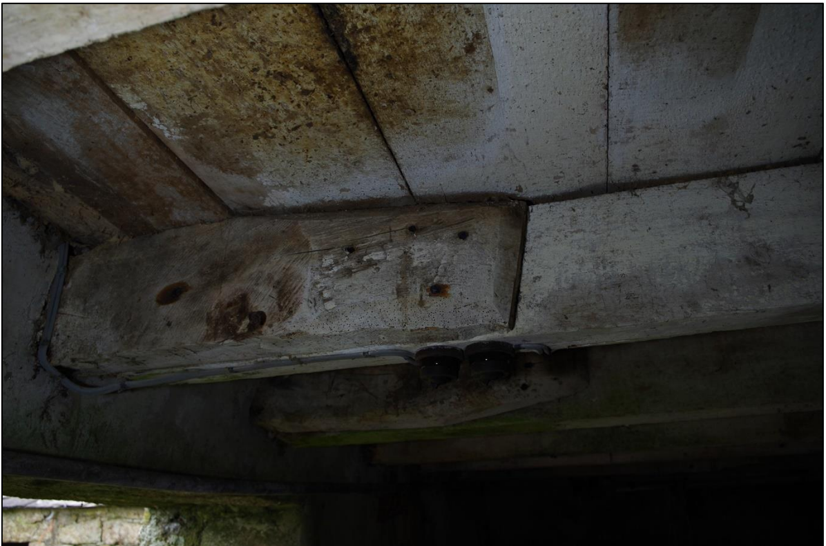
38. BRACED JOISTS ABOVE DOOR TO GF B2.
