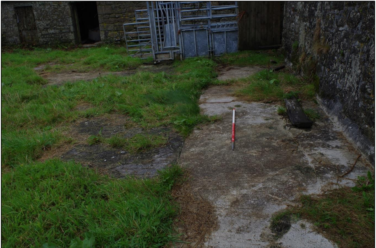
43. LIMECRETE YARD ALONG WEST ELEVATION OF B2 ; FROM THE SOUTH (1M SCALE).
