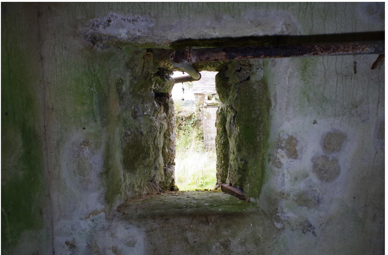
36. W6 SLIT VENT WITH DEEPLY SPLAYED SIDES, LARGELY RENDERED WITH LARGE SPIKE TO SILL; FROM THE EAST.
