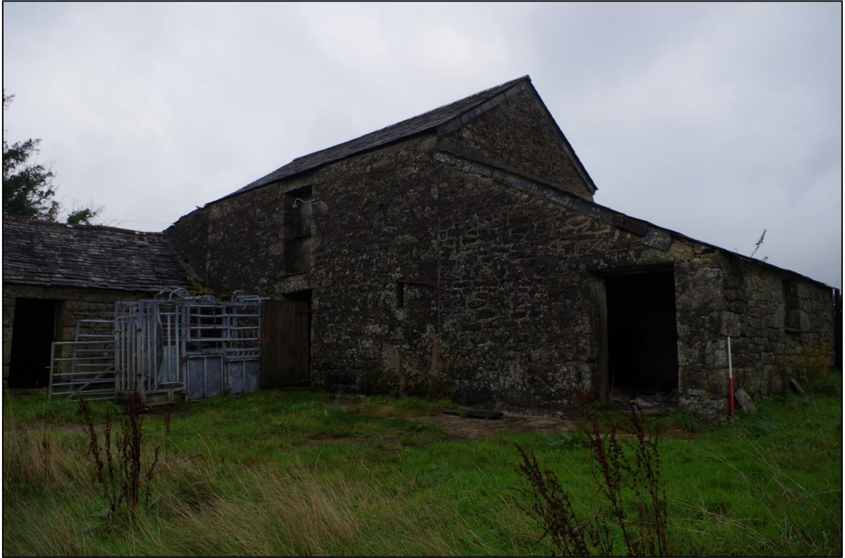
18. WEST ELEVATION OF BUILDING B2 AND B3; FROM THE SOUTH-WEST, (1M SCALE).
