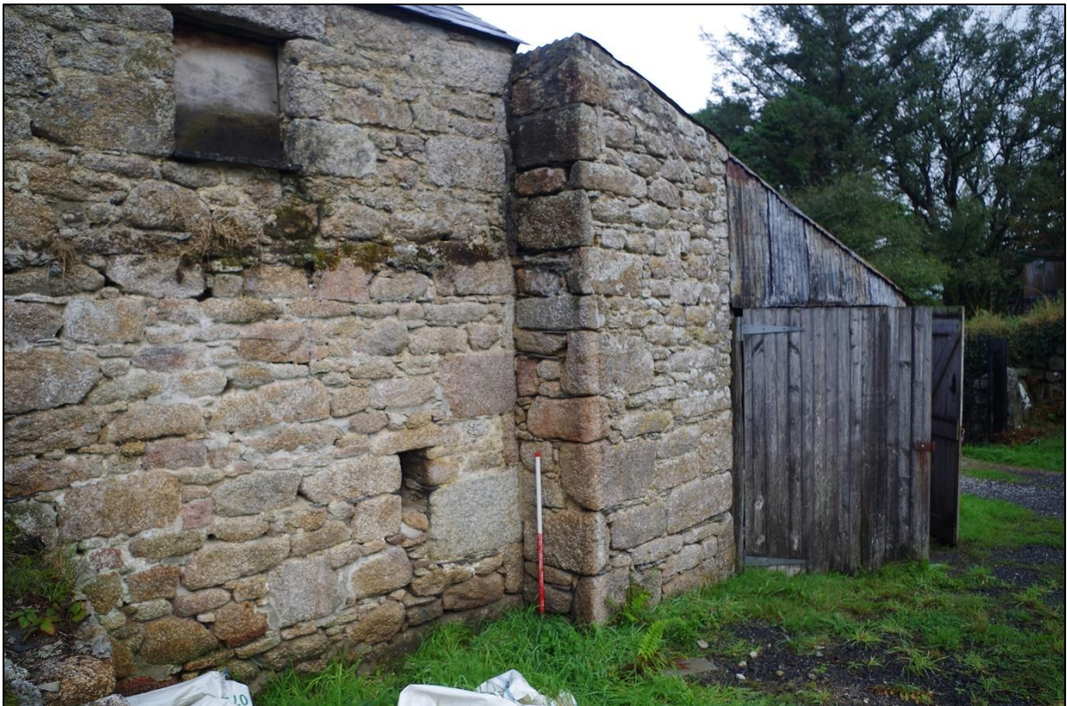
12. EAST ELEVATION SHOWING BUILDING 1 ABUTTING BUILDING 2; FROM THE SOUTH-EAST, (1M SCALE).
