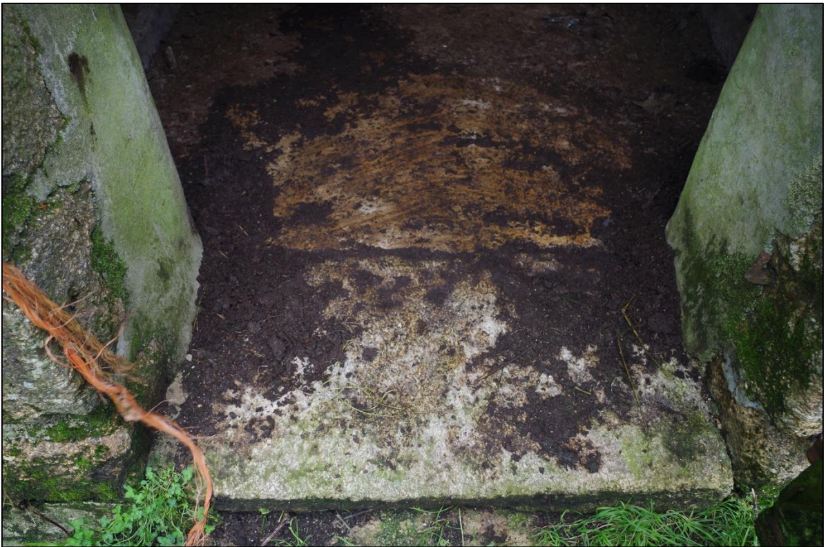
42. SLABBED GRANITE THRESHOLD TO GF ENTRANCE OF B2.
