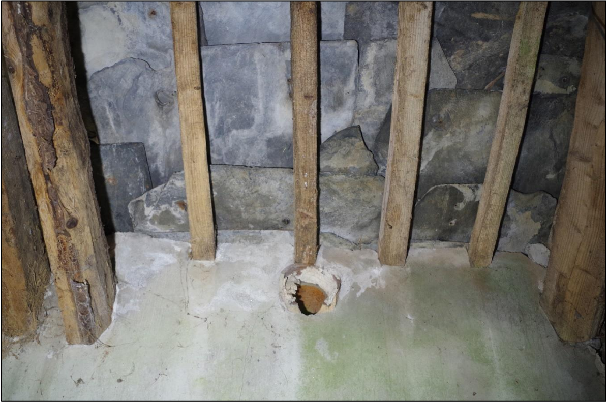
59. TERRACOTTA AIR VENTS TO EAVES OF B4A & B.
