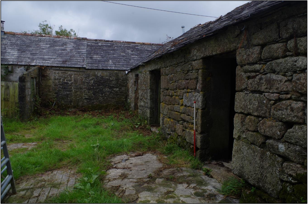
FIGURE 15: B4 AGAINST ANOTHER SMALLER BLOCK NOW CONVERTED INTO A HOLIDAY LET. BLOCKED DOORWAY VISIBLE, SUGGESTING THE BLOCK ADDRESSED THIS YARD INITIALLY, WITH LATER INFILL TO THE NORTH; FROM THE EAST (1M SCALE).
