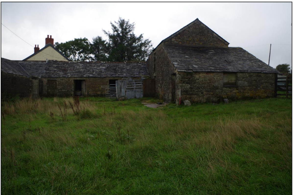
17. CENTRAL OVERGROWN FARMYARD; TAKEN FROM THE SOUTH (1M SCALE).
