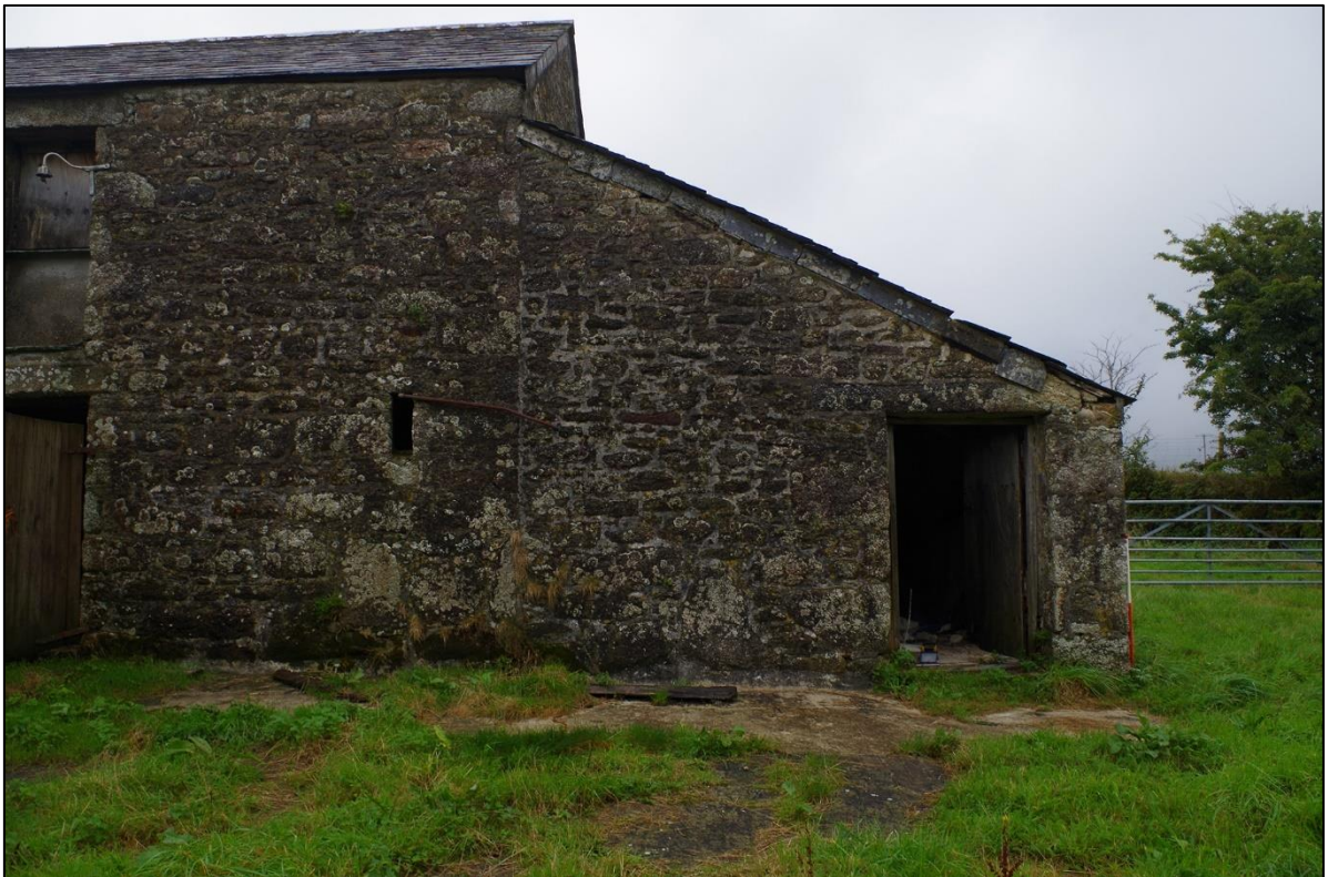
19. WEST ELEVATION SHOWING BUILDING 3 ABUTTING BUILDING 2; FROM THE WEST (1M SCALE).
