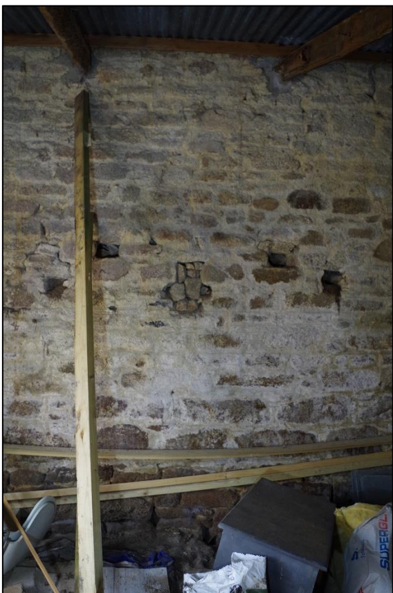
25. (LEFT) REMAINING FORCED SOCKET HOLES TO THE SOUTH ELEVATION – FOR EARLIER MACHINERY. TAKEN FROM THE NORTH.
