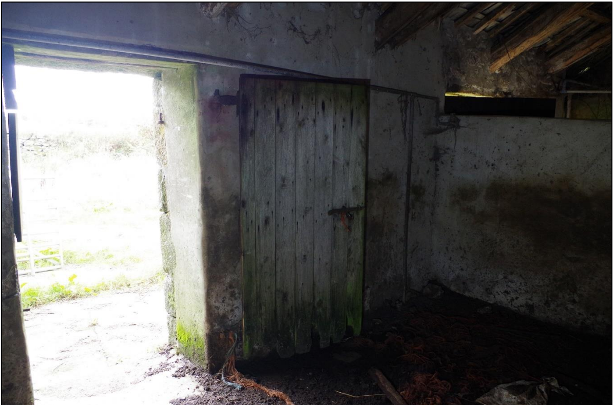
58. MODERN DOOR ON EARLIER HEAVY LINTELS AND STRAPS ON D7 TO B4B; FROM THE NORTH-EAST.
