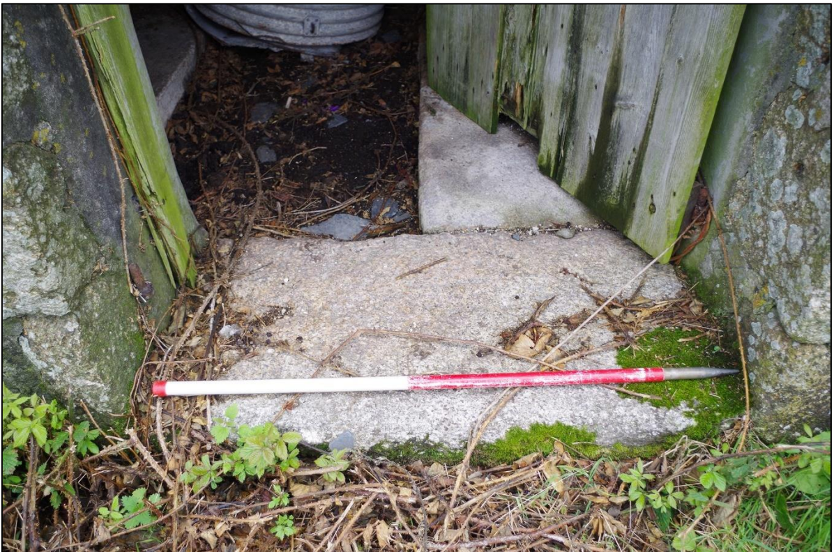
50. GRANITE SLABBED THRESHOLD TO B4A; (1M SCALE).
