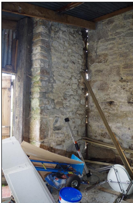
25. (LEFT) REMAINING FORCED SOCKET HOLES TO THE SOUTH ELEVATION – FOR EARLIER MACHINERY. TAKEN FROM THE NORTH.
