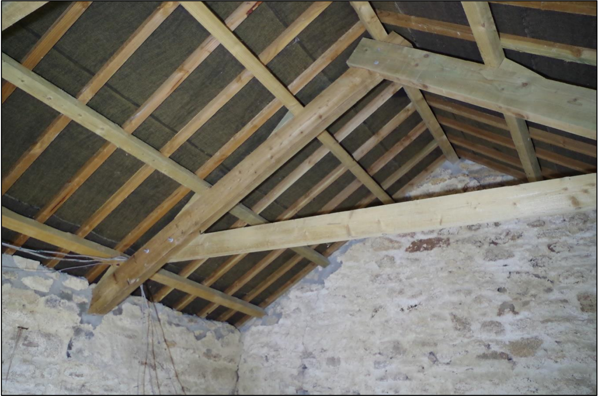
29. MODERN ROOF REPLACEMENT TO B2.
