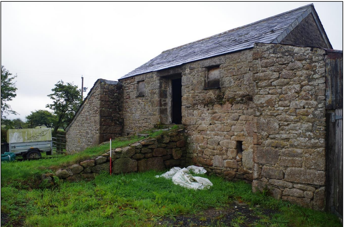
10. THE EAST ELEVATION OF B2 WITH STEEP EARTHEN RAMP TO FF LEVEL – A LATER RESTRUCTURE; FROM THE NORTH-EAST (1M SCALE).
