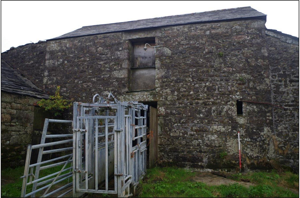
20. WEST ELEVATION OF BUILDING 2; TAKEN FROM THE WEST (1M SCALE).
