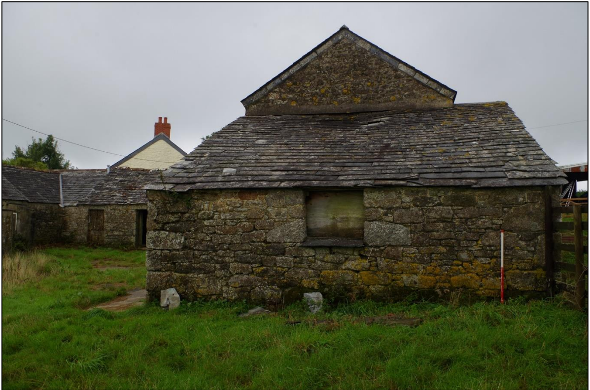
16. SOUTH ELEVATION OF BUILDING 3; FROM THE SOUTH (1M SCALE).
