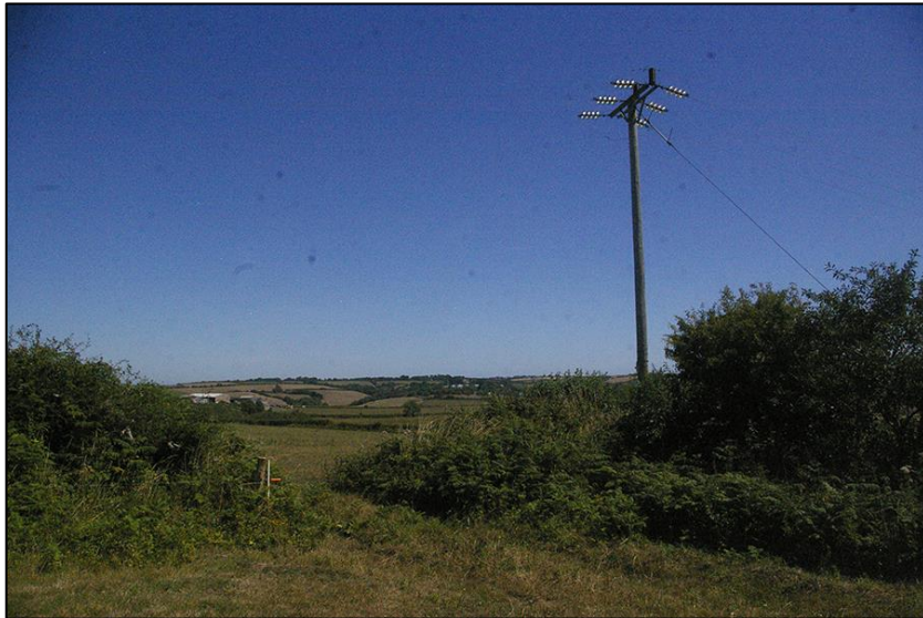
11. OVERHEAD CABLES BESIDE ACCESS GATE IN EAST CORNER OF SITE; VIEWED FROM THE WEST (1M SCALE).
