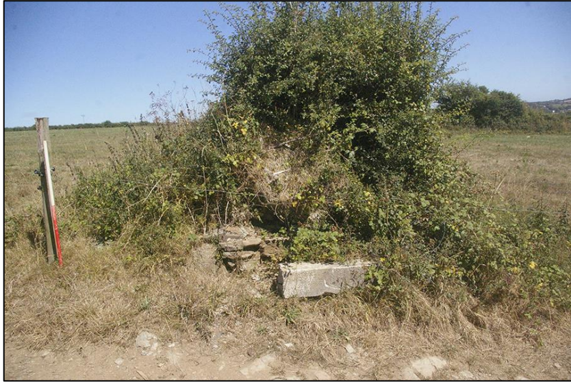
7. BOUNDARY BANK IN ACCESS GATE (PHOTO 6); VIEWED FROM THE SOUTH-WEST (1M SCALE).
